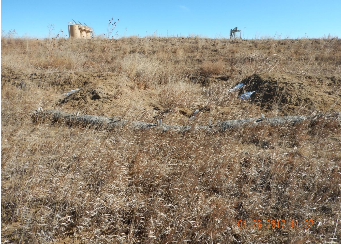
Photo 6. Photo taken from the southern sediment trap along the western location, facing East. Sediment was observed outside of containment area beyond the wattle.
