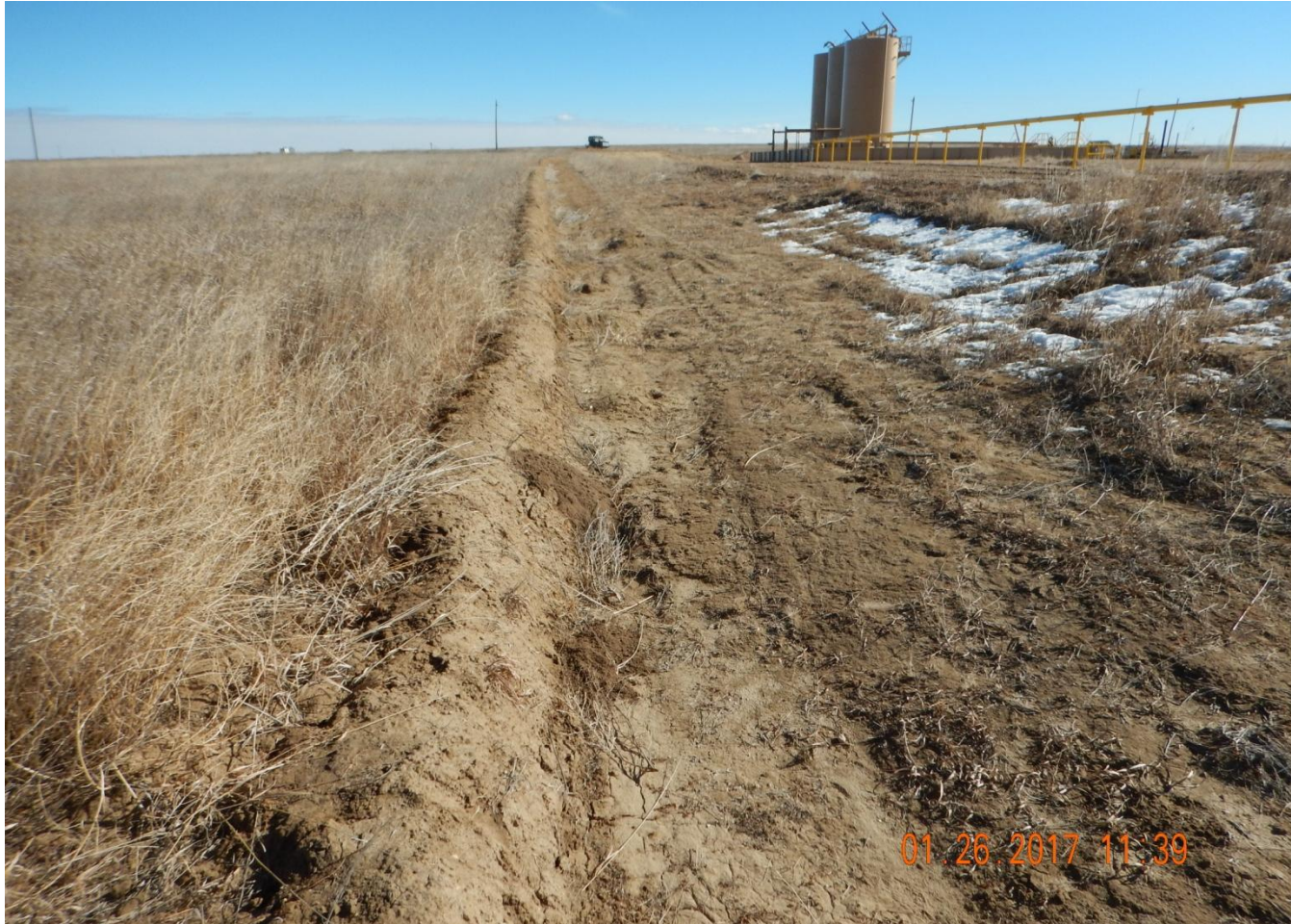
Photo 8. Photo taken from the northwest corner of location, facing East. Berm BMP installed along the northern location.
