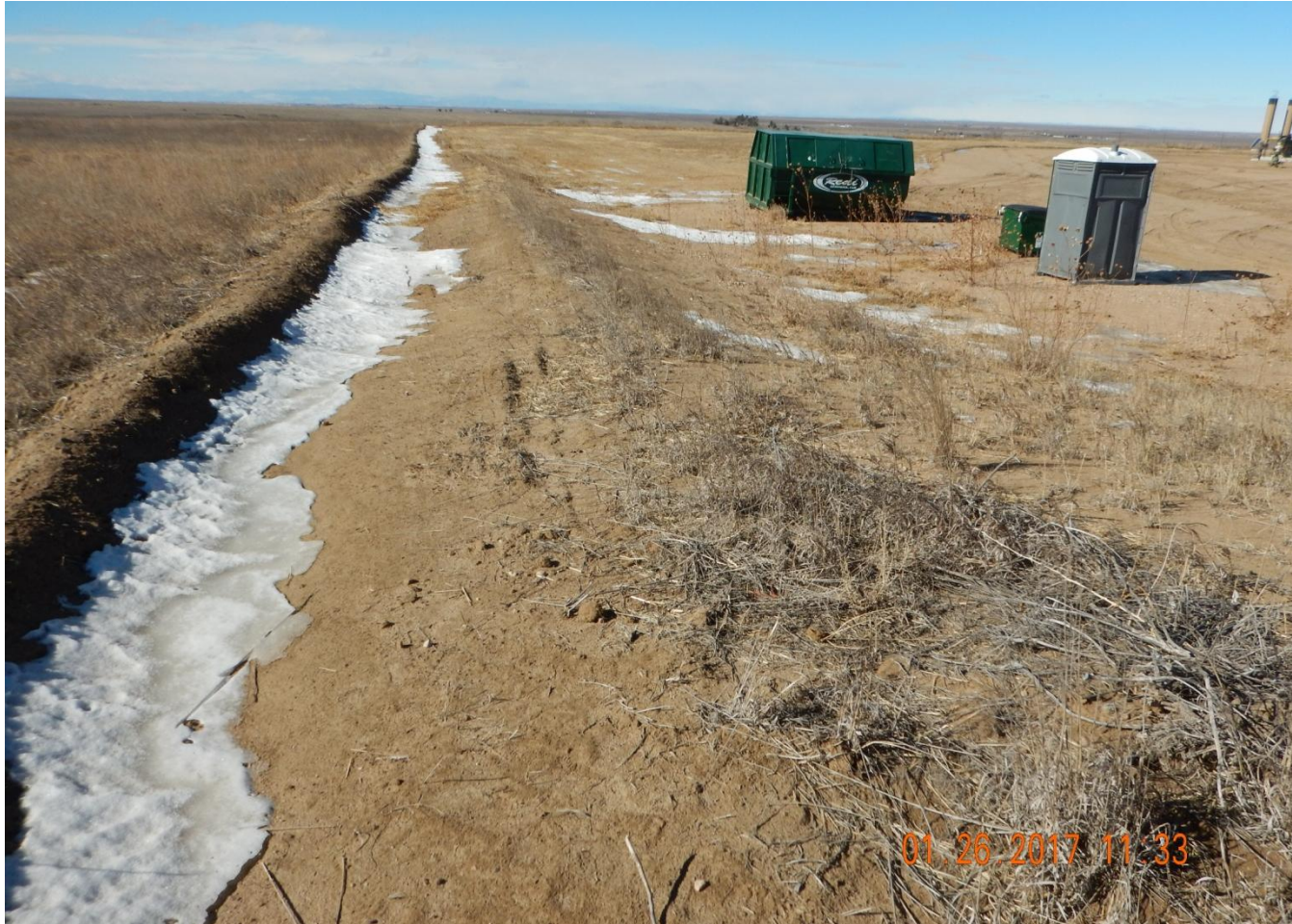
Photo 2. Photo taken from the southeast location, facing West. Ditch and berm BMP installed along the southern location.
