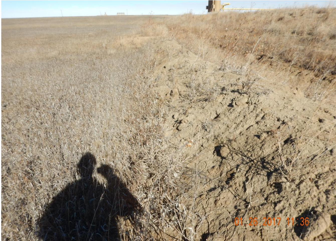
Photo 5. Photo taken from the western location, facing North. The outer berm does not appear to be compacted and active rill erosion is occurring.
