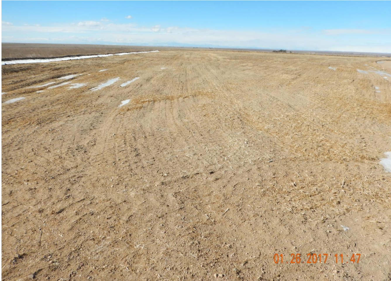
Photo 11. Photo taken of the southern interim area, facing West. Evidence of reclamation activities apparent but mulch does not appear to be sufficiently crimped. Mulch was observed in throughout the perimeter of the disturbance area. May need to monitor interim areas to ensure areas are protected from erosion.
