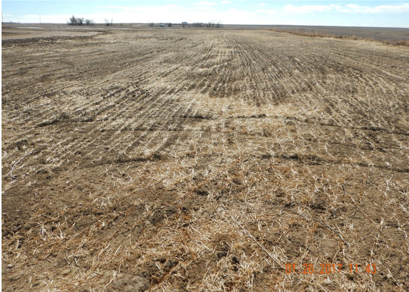
Photo 10. Photo taken of the northern interim area, facing South. Evidence of reclamation activities apparent but mulch does not appear to be sufficiently crimped. Mulch was observed in throughout the perimeter of the disturbance area. May need to monitor interim areas to ensure areas are protected from erosion.
