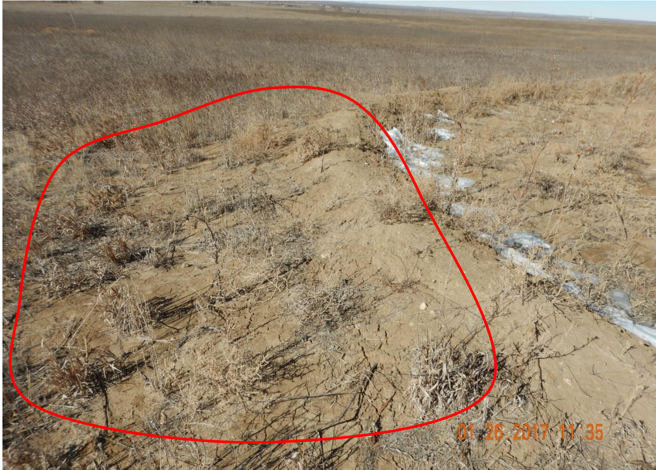
Photo 3. Photo taken from the southwest location, facing Northwest. Appears sediment has either discharged from location or sediment erosion has occurred because the berm BMP was never compacted properly.
