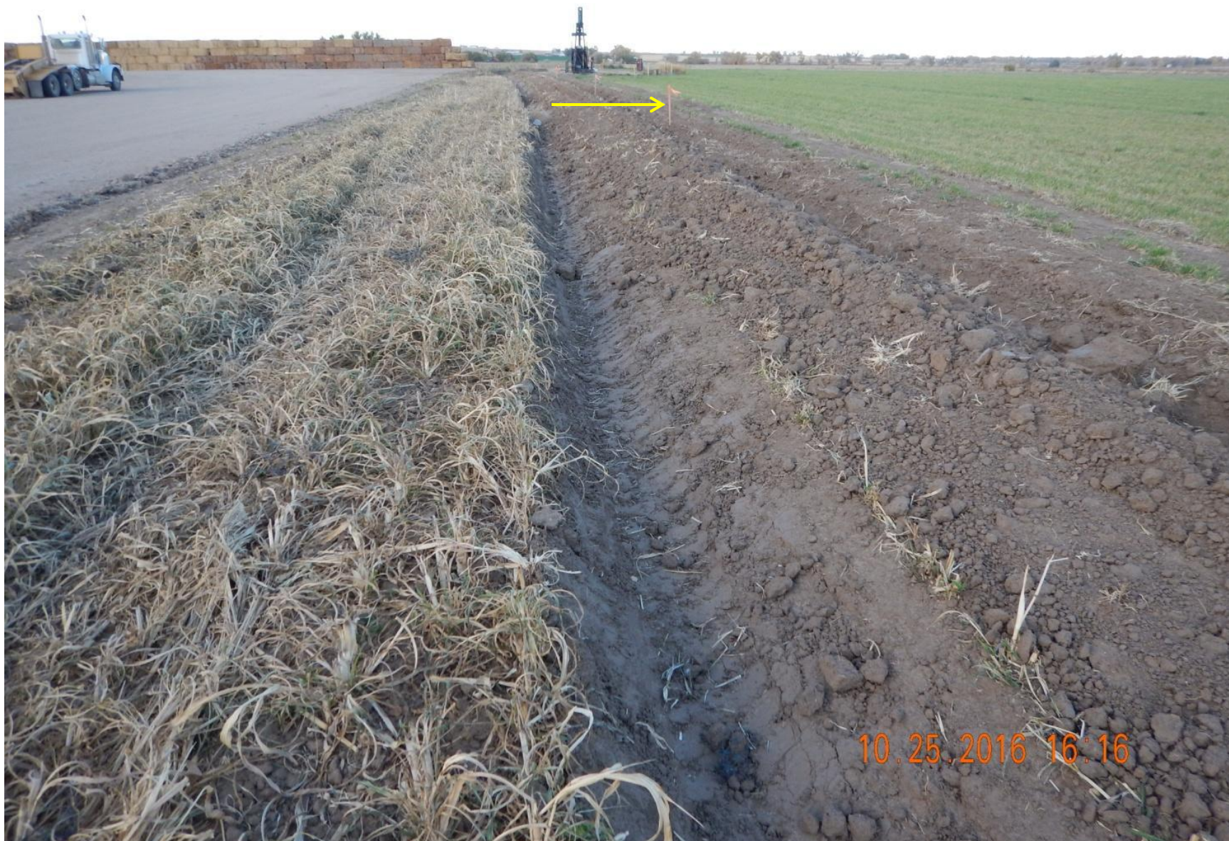
Figure 9: Photo taken from inspection doc. #682401425. This was a construction, pre-drill inspection. Photo shows ditch on the east end of the location, and the soil deposited on the adjacent surface owners property. Stakes shown with yellow arrow marks property line.
