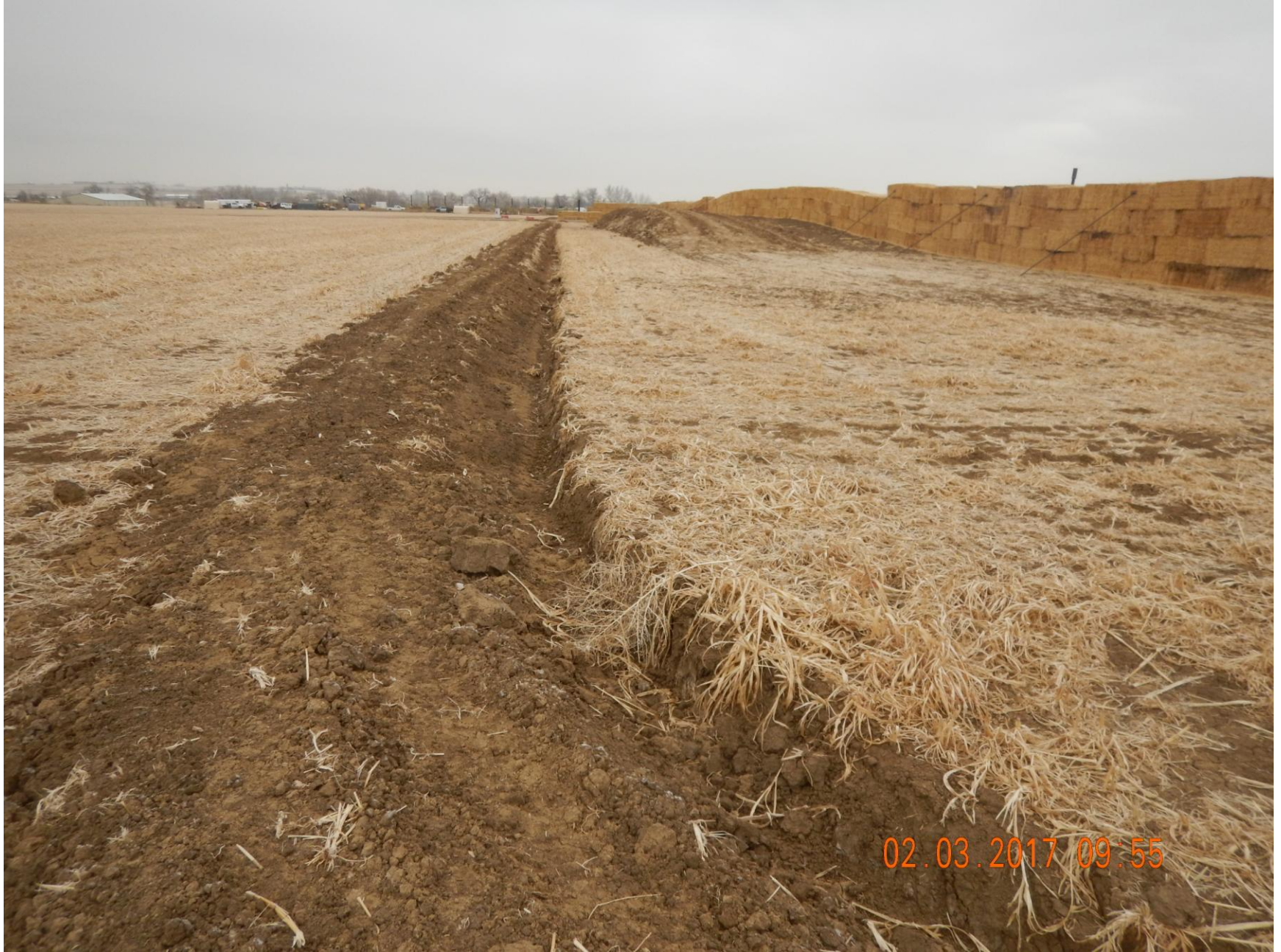
Figure 13: Photo taken from the southwest corner of the location, facing north. Photo shows ditch along the perimeter of the location constructed as a stormwater and sediment control BMP. Photo also shows topsoil stockpile.
