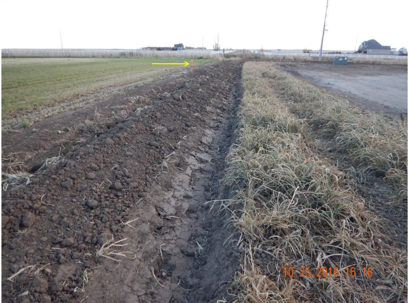
Figure 8: Photo taken from inspection doc. #682401425. This was a construction, pre-drill inspection. Photo shows ditch on the east end of the location, and the soil deposited on the adjacent surface owners property. Stakes shown with yellow arrow marks property line.
