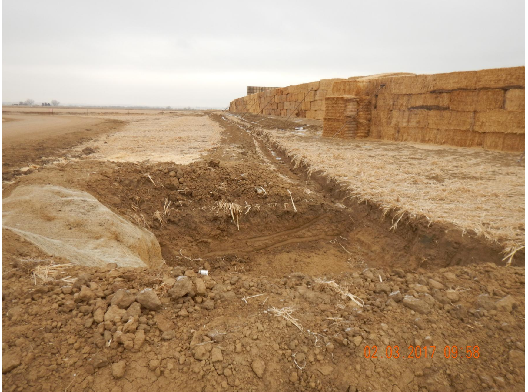
Figure 18: Photo taken from the northwest corner of the location, facing east. Photo shows ditch along the perimeter of the location, and sediment trap constructed as a stormwater and sediment control BMPs.
