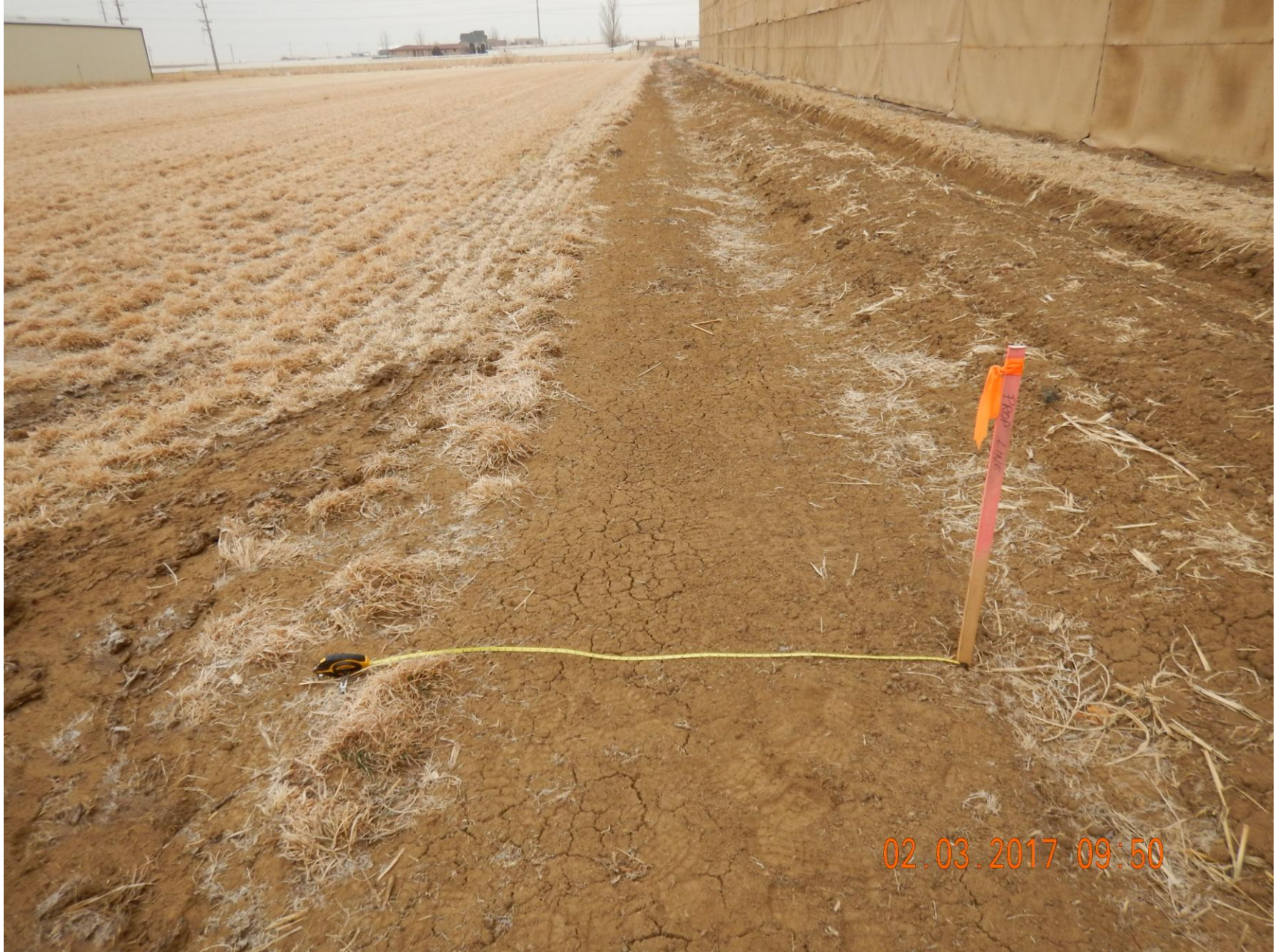
Figure 6: Photo taken from the east end of the location, facing south. Photo shows a five (5) foot wide strip on the adjacent surface owner's land that is void of vegetation due to disturbances caused during construction.
