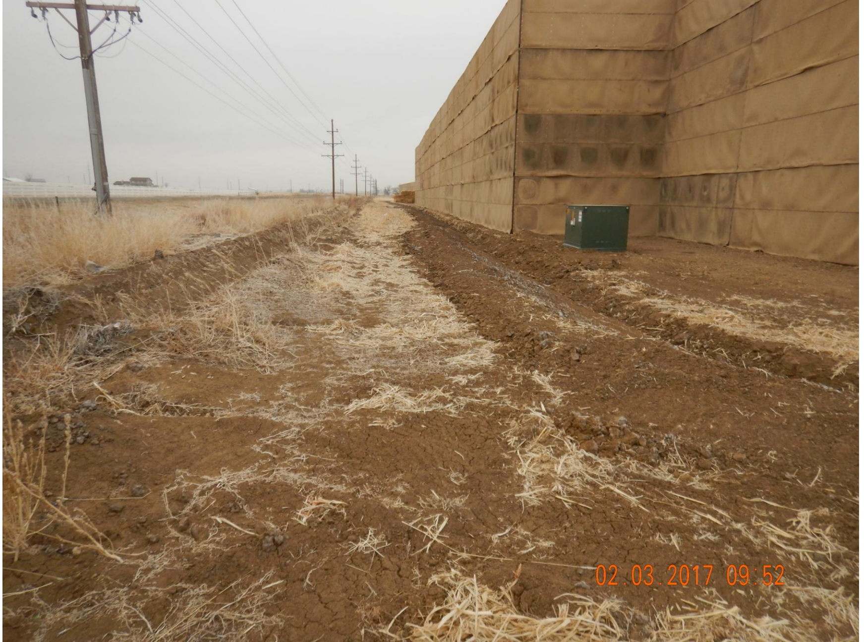
Figure 11: Photo taken from the southeast corner of the location, facing west. Photo shows ditch along the perimeter of the location constructed as a stormwater and sediment control BMP.
