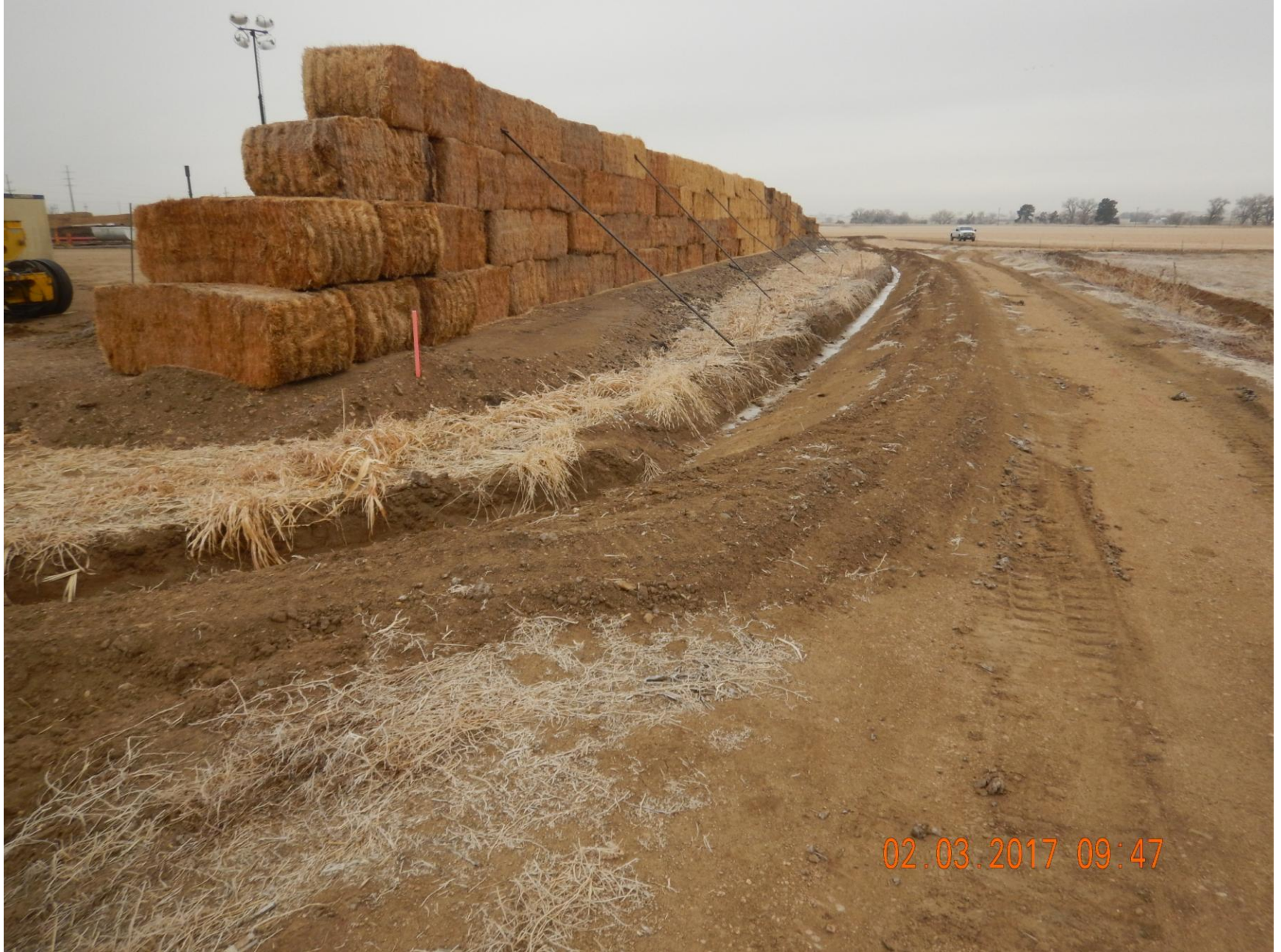
Figure 1: Photo taken from the northeast corner of the location, facing west. Photo shows ditch along the perimeter of the location constructed as a stormwater and sediment control BMP.
