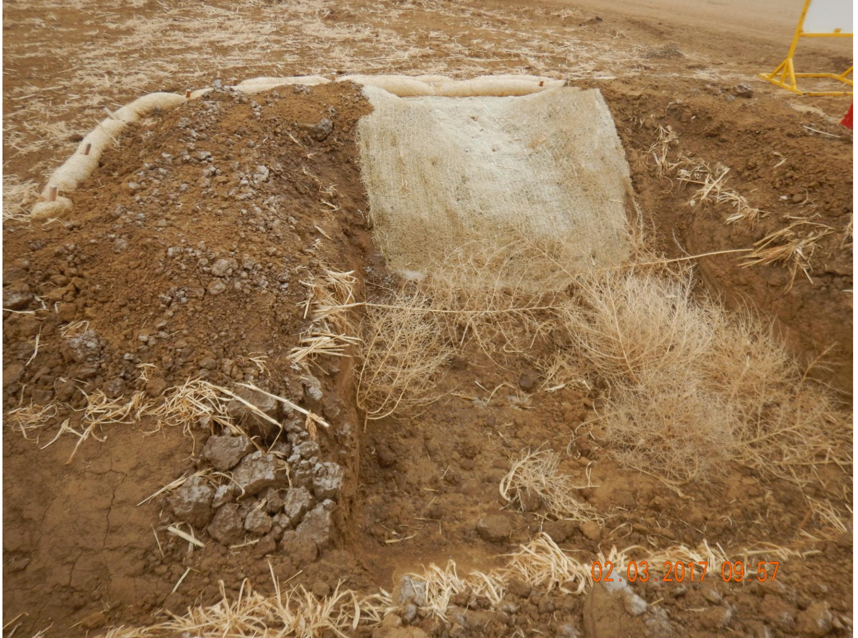
Figure 14: Photo taken from the northwest end of the location, near location entrance. Photo shows one of two sediment traps used as a stormwater and sediment control BMP.
