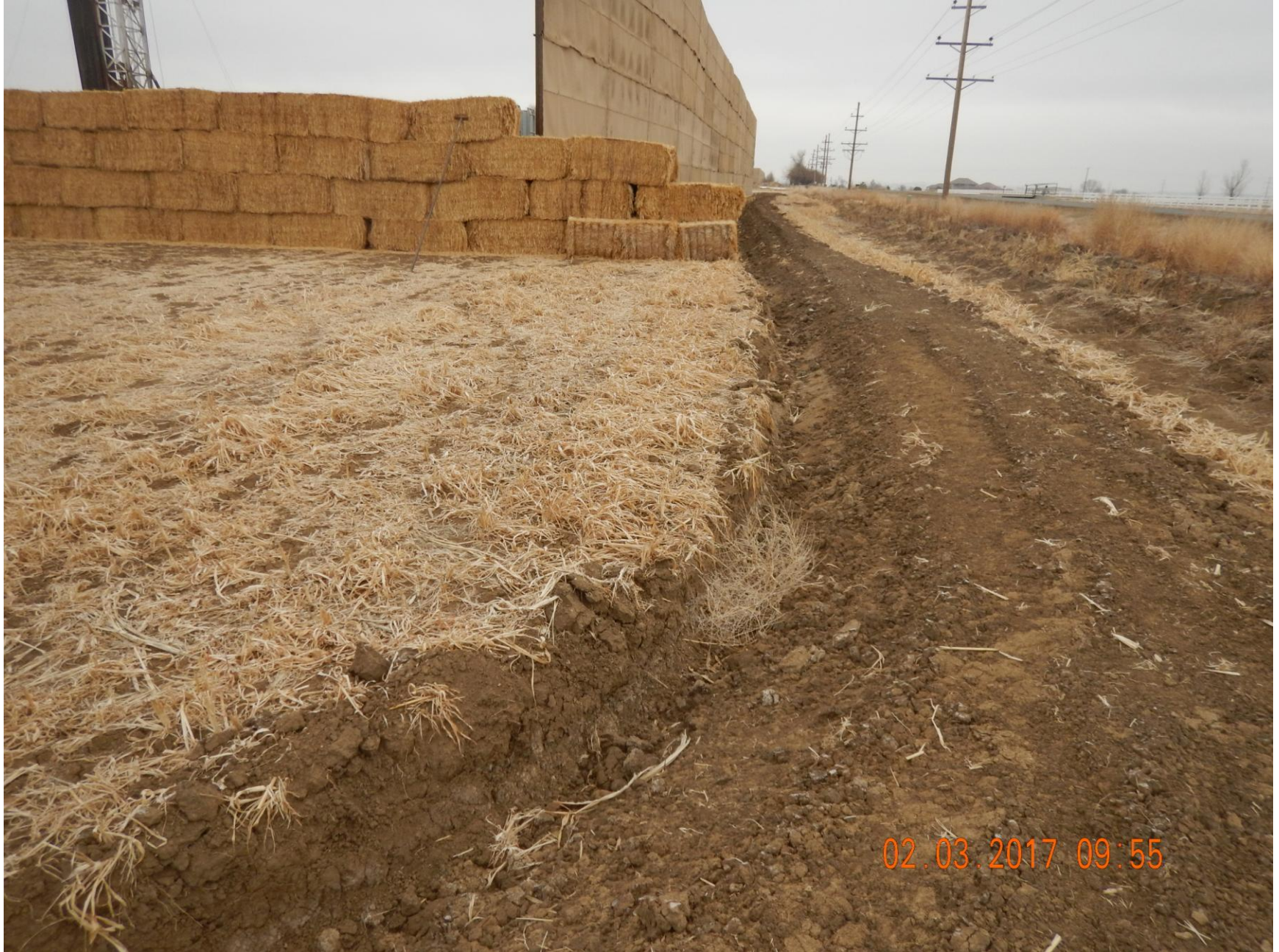
Figure 12: Photo taken from the southwest corner of the location, facing east. Photo shows ditch along the perimeter of the location constructed as a stormwater and sediment control BMP
