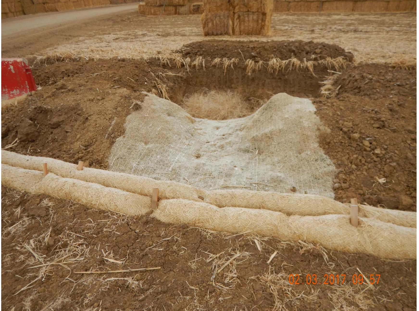
Figure 15: Photo taken from the northwest end of the location, near location entrance. Photo shows one of two sediment traps used as a stormwater and sediment control BMP.
