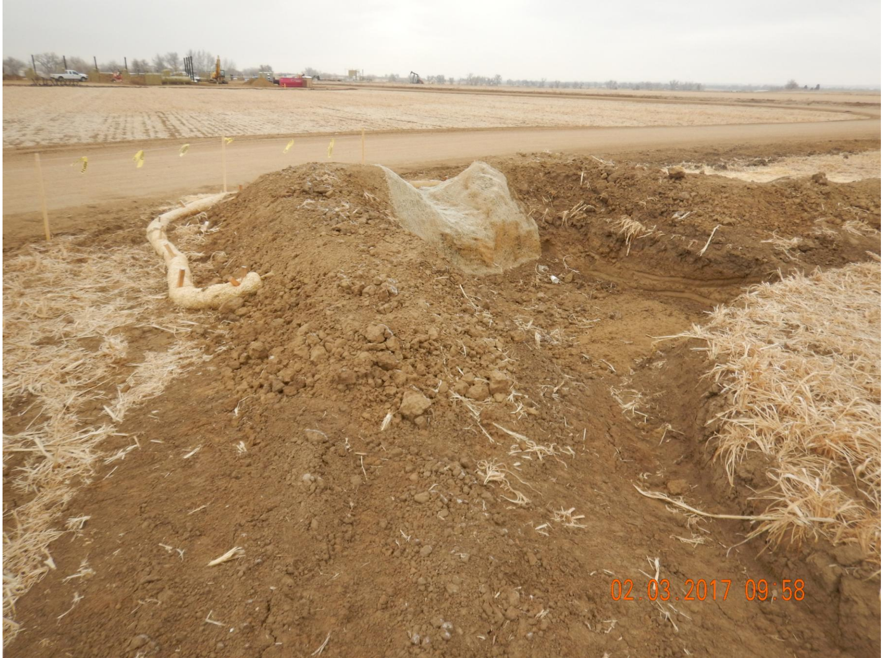
Figure 16: Photo taken from the northwest end of the location. Photo shows second sediment trap use as a stormwater and sediment control BMP.
