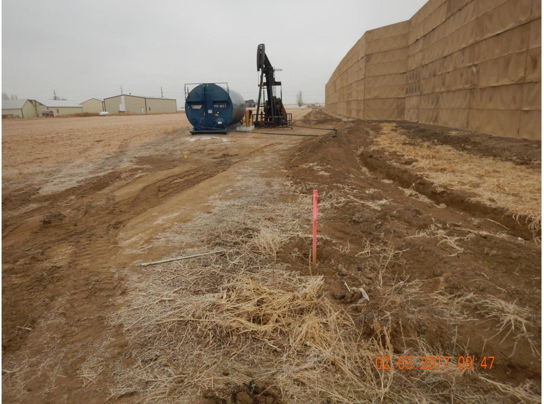
Figure 2: Photo taken from the northeast corner of the location, facing south. Photo shows ditch along the perimeter of the location constructed as a stormwater and sediment control BMP. Pump jack and well seen in photo not associated with the location in this inspection.
