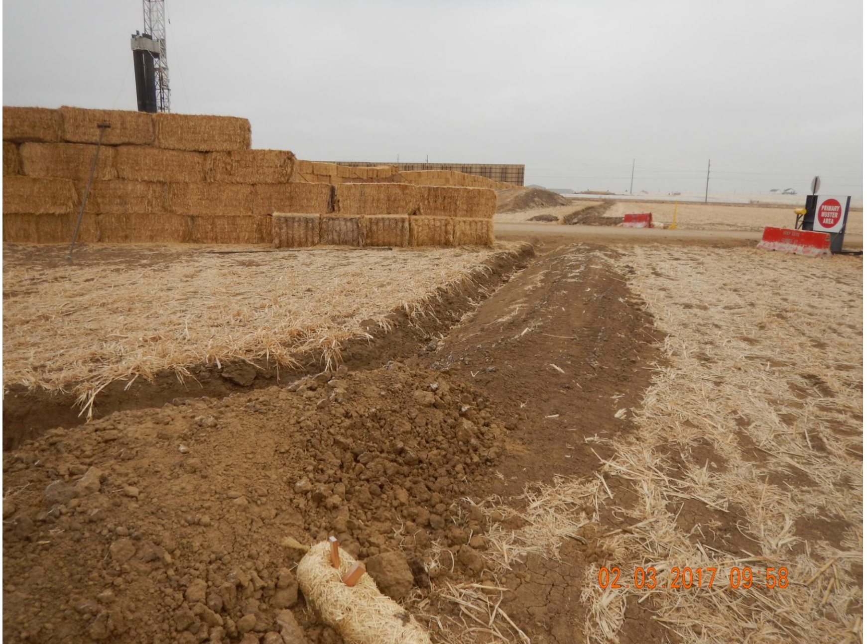
Figure 17: Photo taken from the northwest corner of the location, facing south. Photo shows ditch along the perimeter of the location constructed as a stormwater and sediment control BMP.
