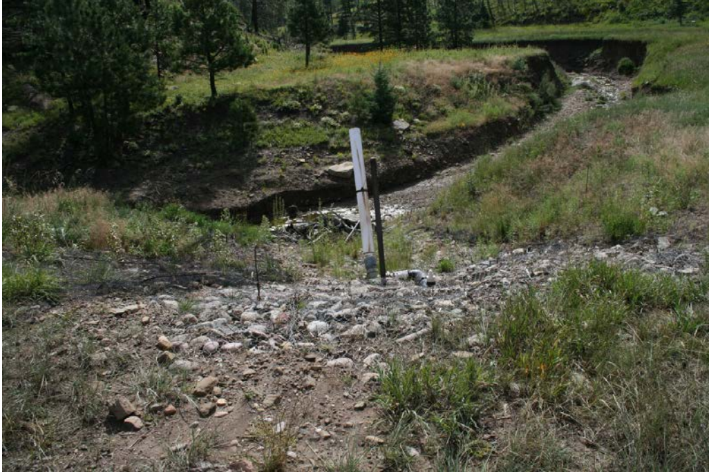
Photograph 3. Pond E, facing east from south end of dam.
