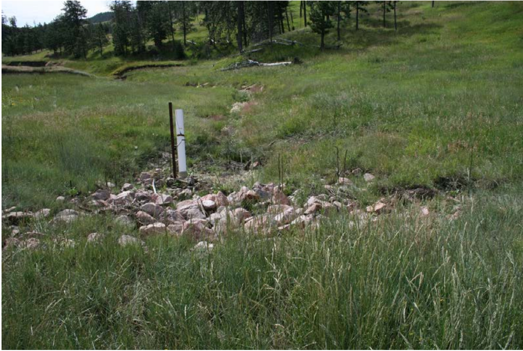
Photograph 3. Pond D, facing southeast from dam.
