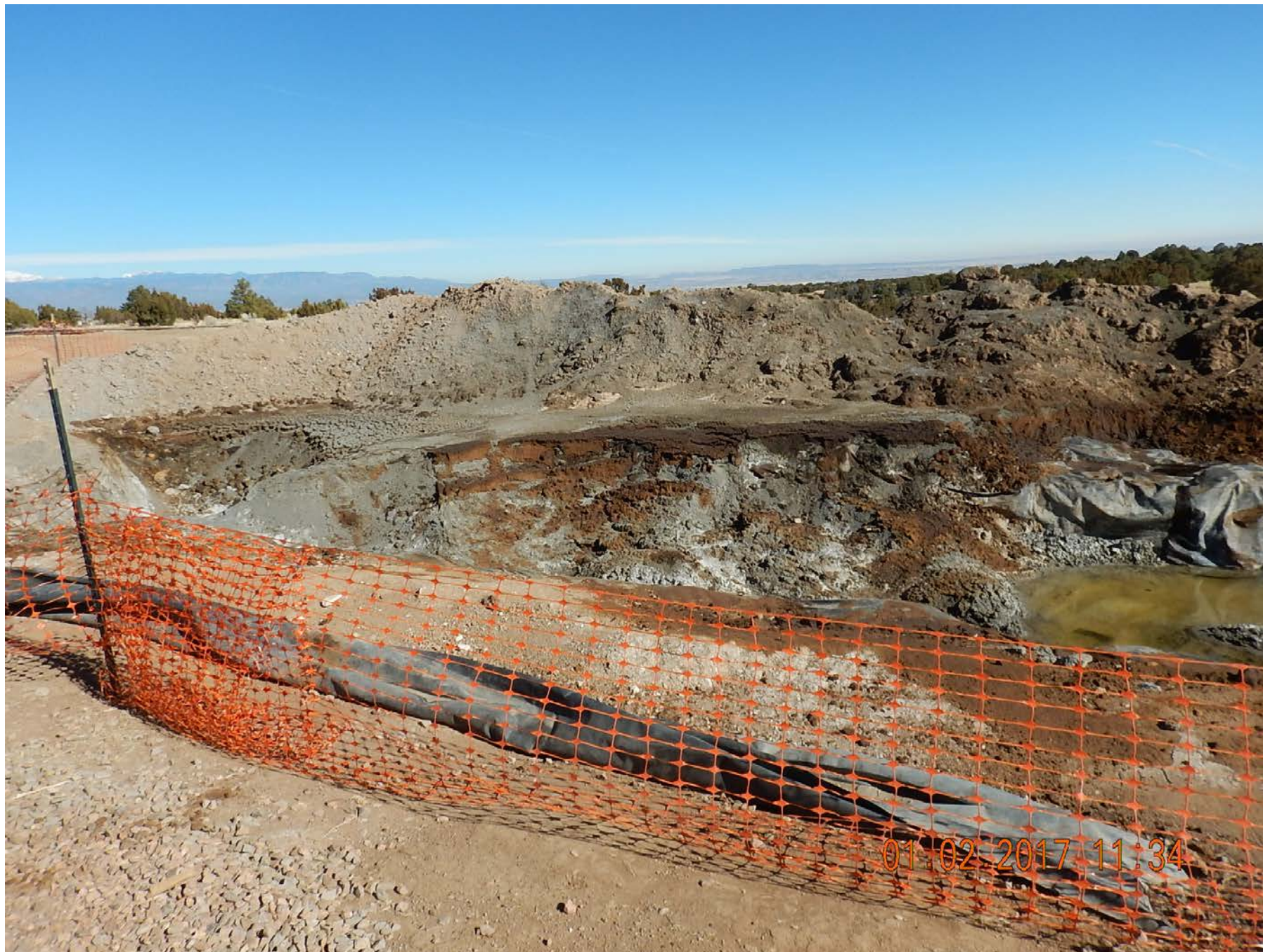
Drill pit cuttings. Fluid appeared to be precipitation and only de minimus amounts of oily fluid was observed.
