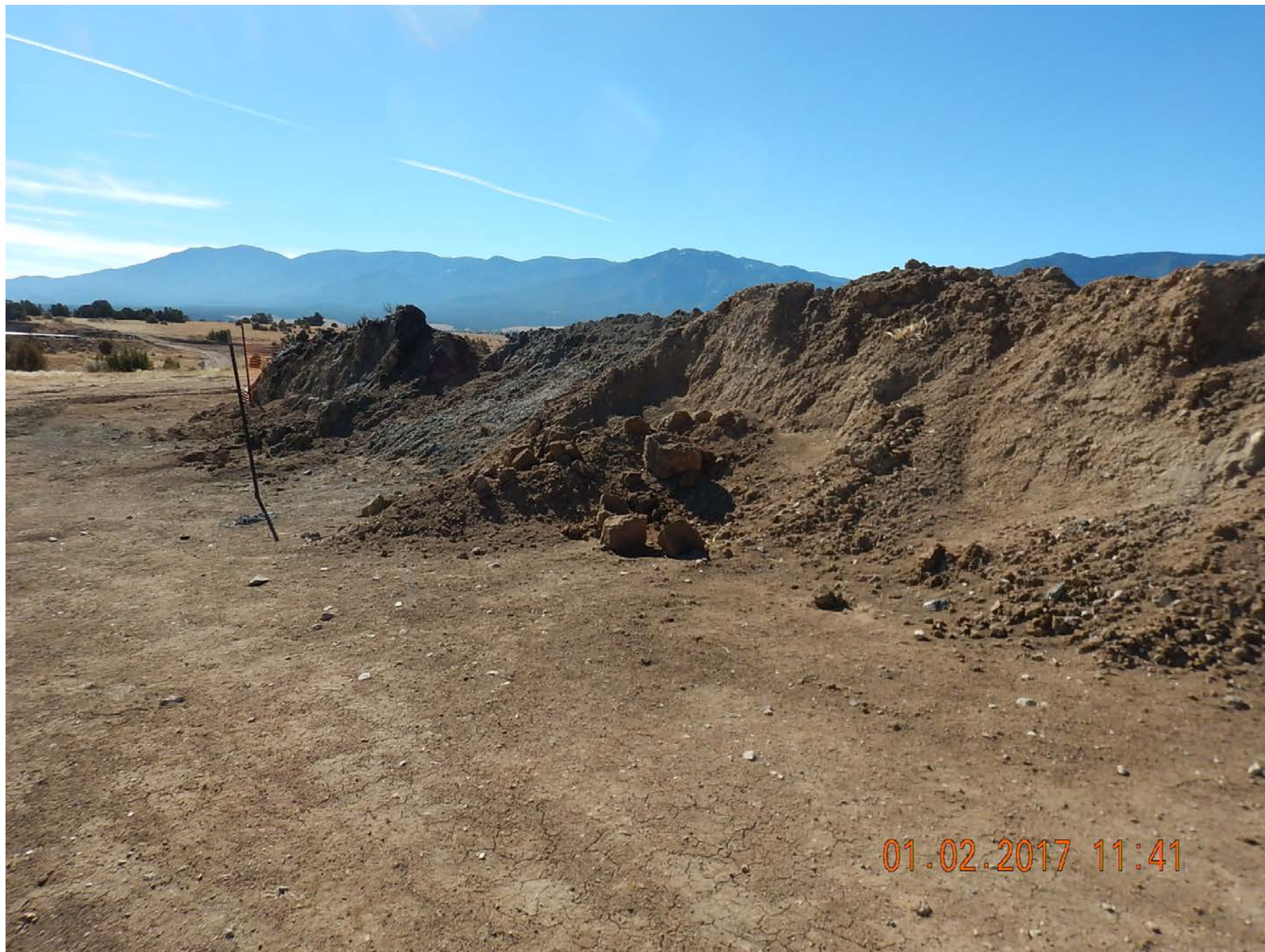
Stormwater controls have not been installed.
