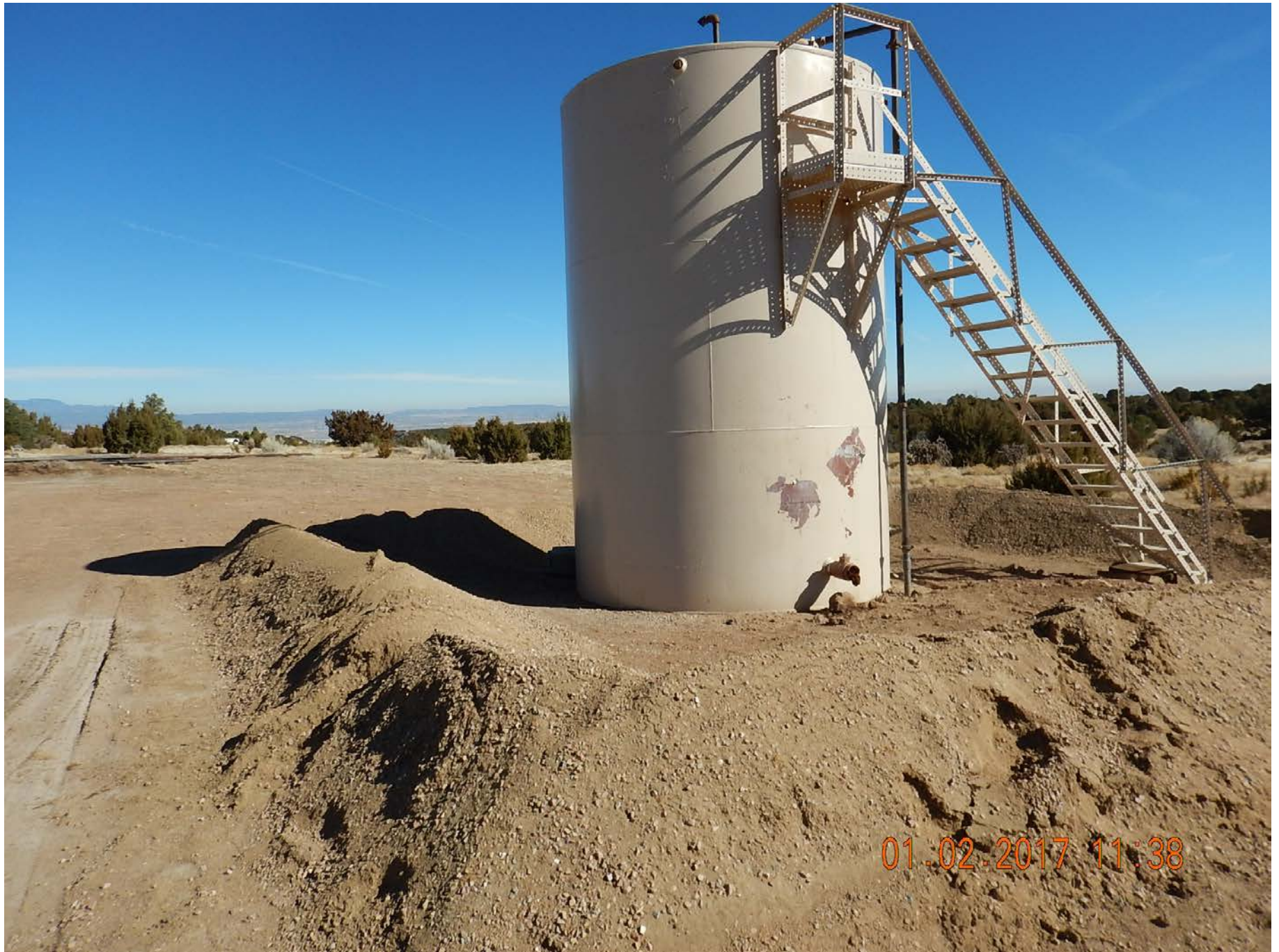
Berm around production tank.
