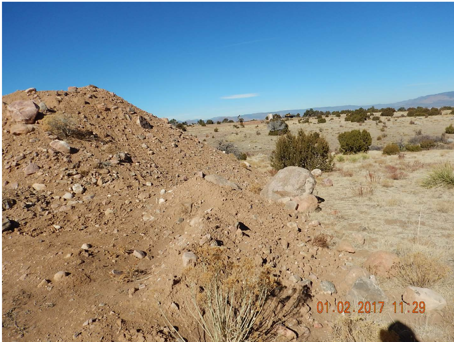
Soil pile lacks sediment control.
