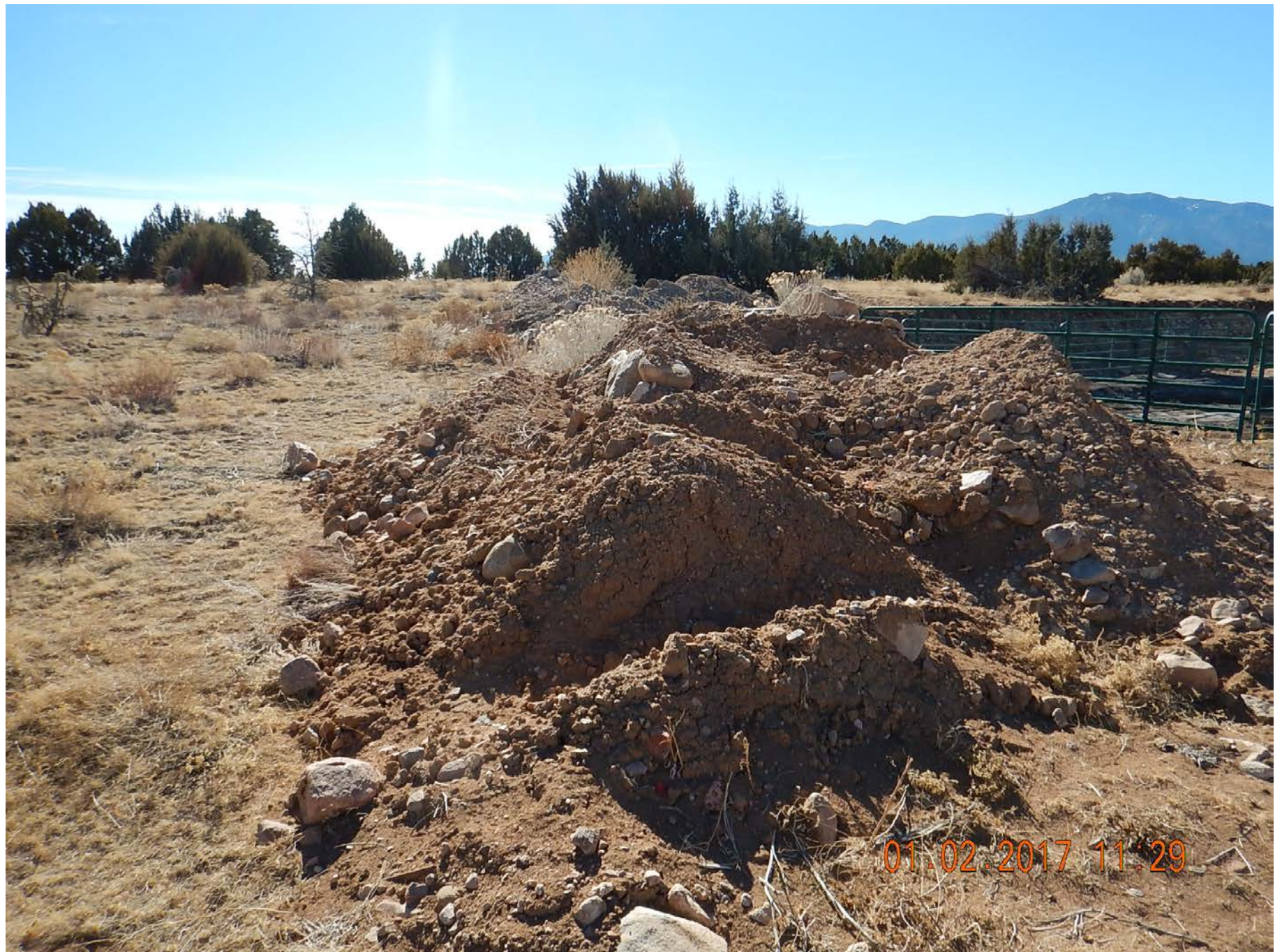
Soil pile lacks sediment control.
