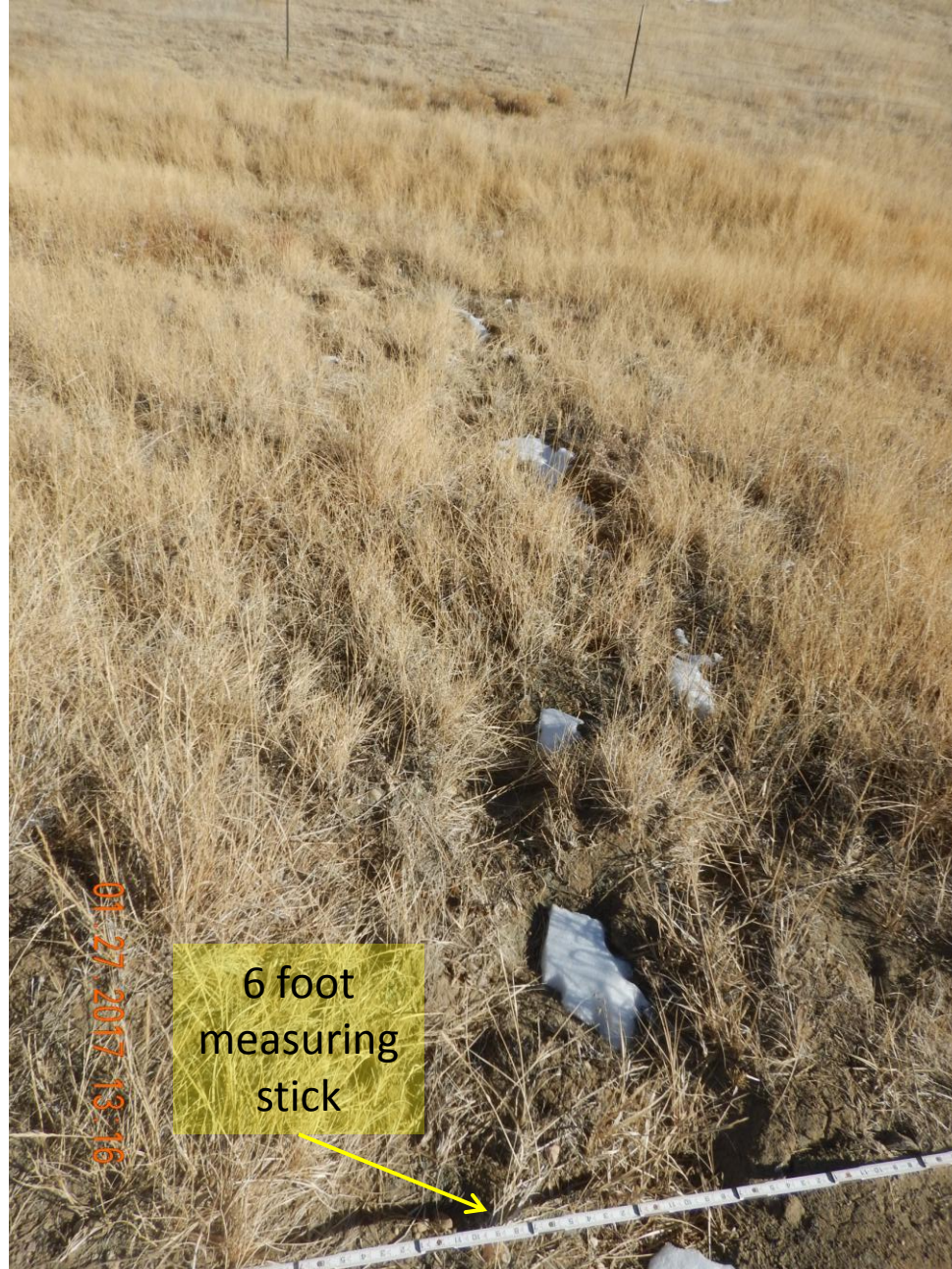
Figure 18: Photo taken from the east end of the project area, facing east. Photo shows a small gully forming due to stormwater erosion degrading the project and interim area. Erosion will need to be repaired and stabilized. Stormwater and sediment control BMPs will need to be installed. 6 foot measuring stick used for reference.
