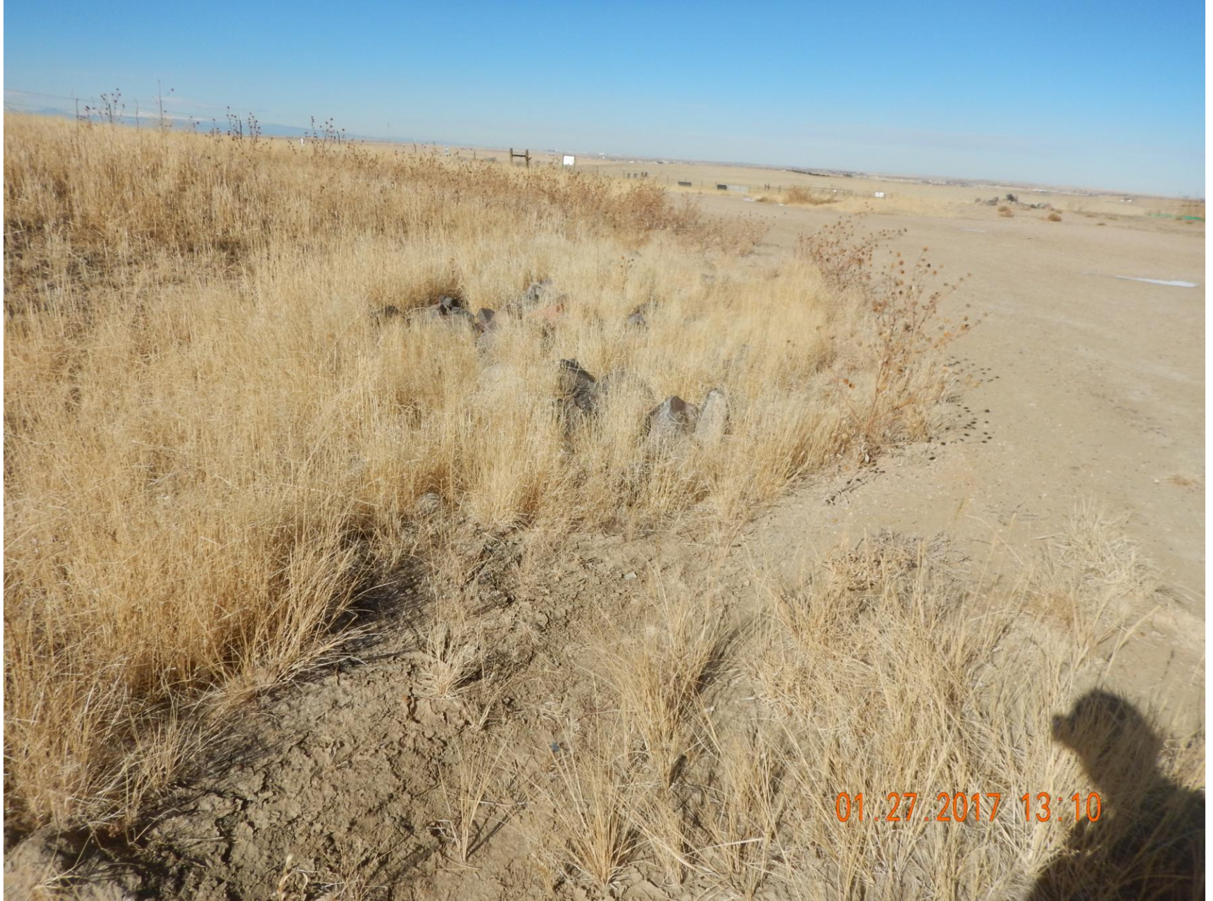
Figure 5: Photo taken from the west end of the project area, facing north. Photo shows sediment trap composed of various sized rock.
