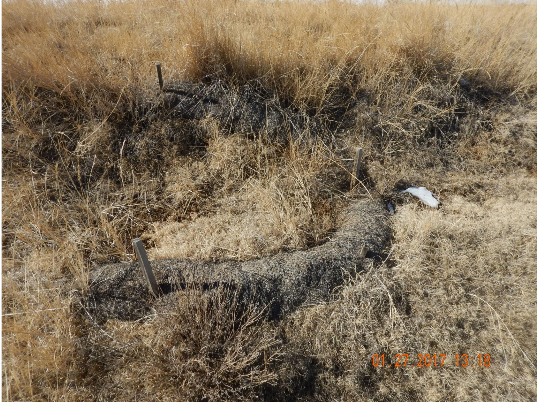
Figure 21: Photo taken from the southeast corner of the location,. Photo shows wattle used as a stormwater and sediment control BMP.
