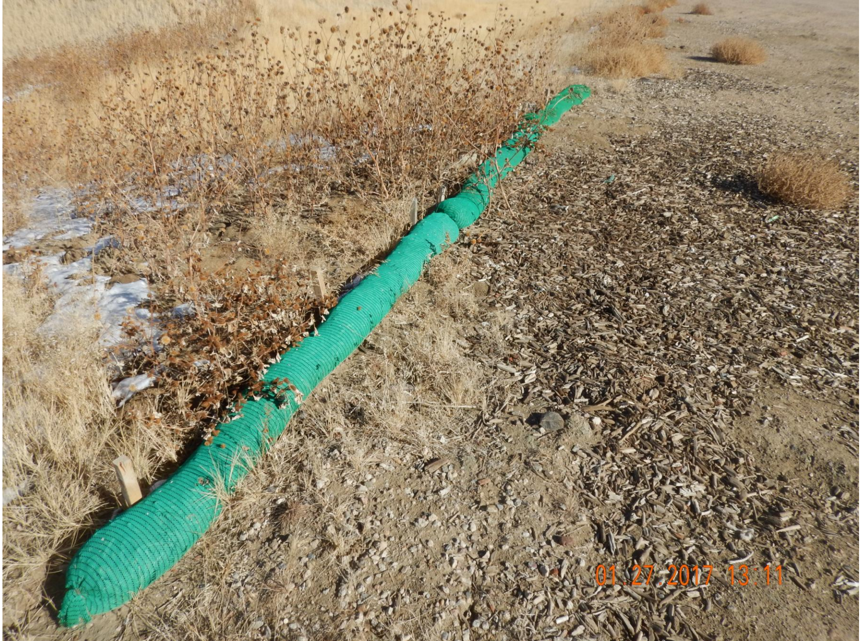
Figure 7: Photo taken from the north end of the location. Photo shows wattle used as a stormwater and sediment control BMP.
