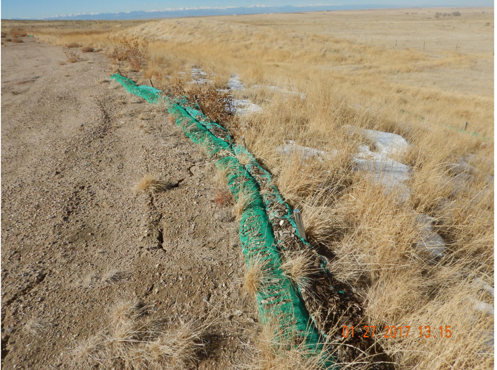
Figure 16: Photo taken from the northeast corner of the location, facing west. Photo shows wattles used as a stormwater and sediment control BMP in disrepair.
