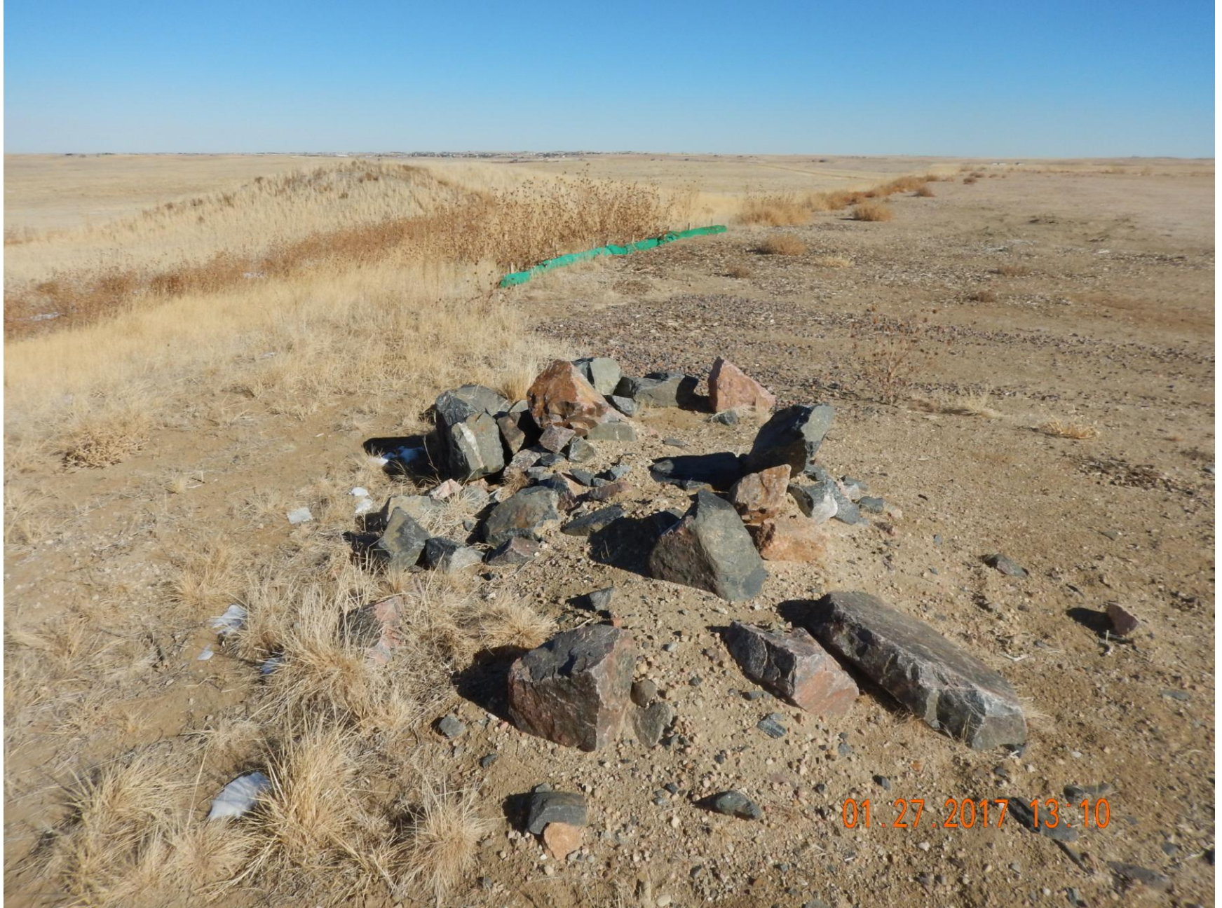
Figure 6: Photo taken from the northwest corner of the project area, facing northeast. Photo rock pile on the location, and wattle used as a stormwater and sediment control BMP.
