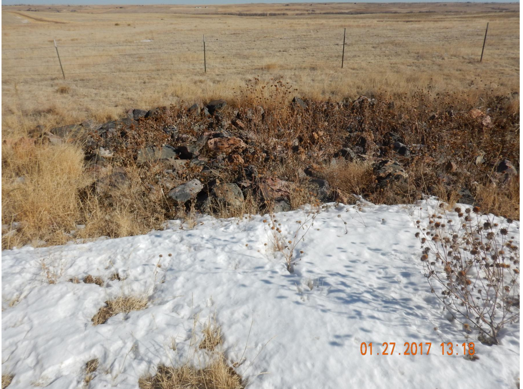
Figure 20: Photo taken from the southeast corner of the location, facing east. Photo shows sediment trapped used as a stormwater and sediment control BMP.
