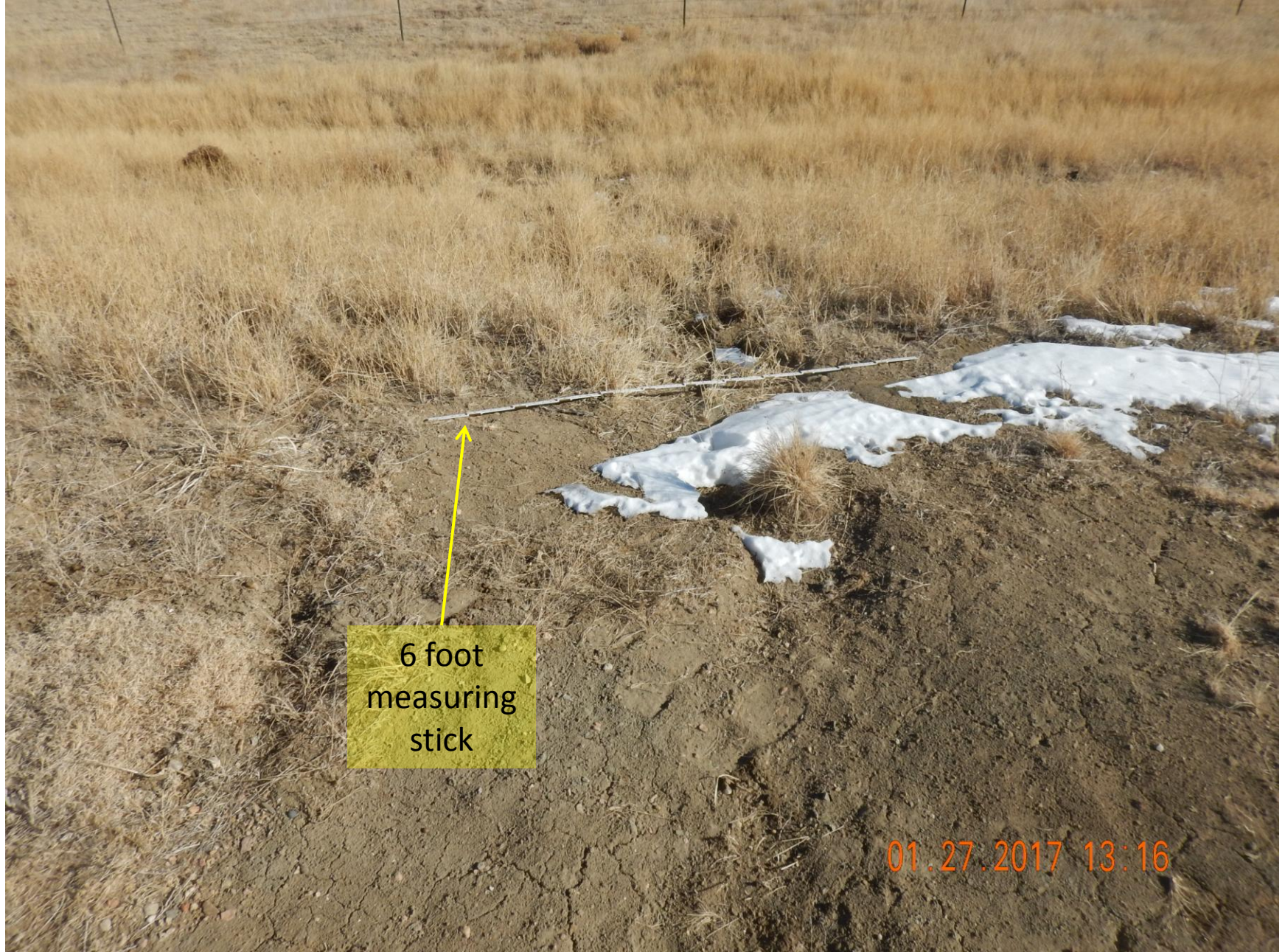
Figure 17: Photo taken from the east end of the project area, facing east. Photo shows a small gulley forming due to stormwater erosion degrading the project and interim area. Erosion will need to be repaired and stabilized. Stormwater and sediment control BMPs will need to be installed. 6 foot measuring stick used for reference.
