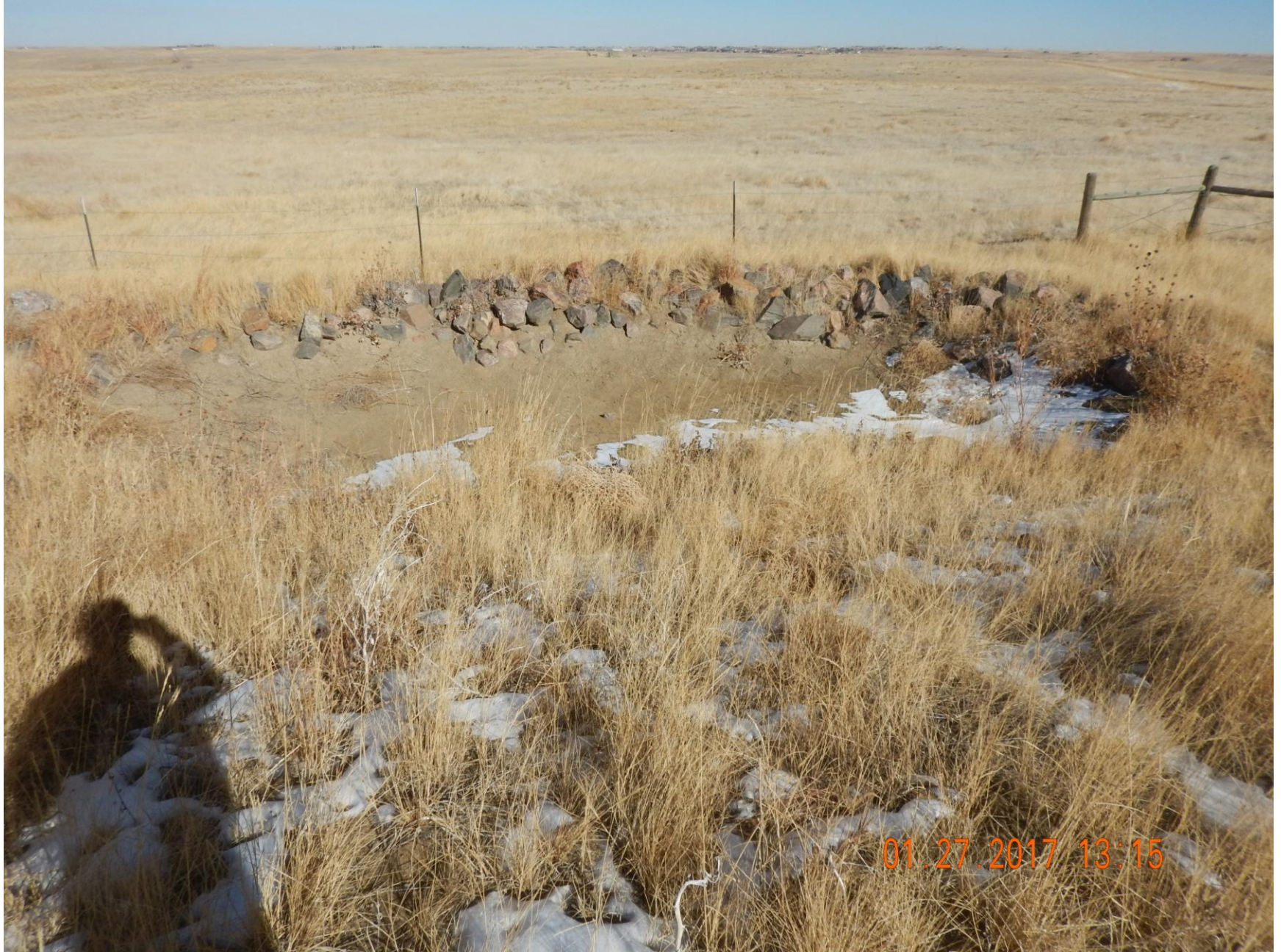
Figure 13: Photo taken from the northeast corner of the current interim area, facing north. Photo shows a sediment trap used as a stormwater and sediment control BMP.
