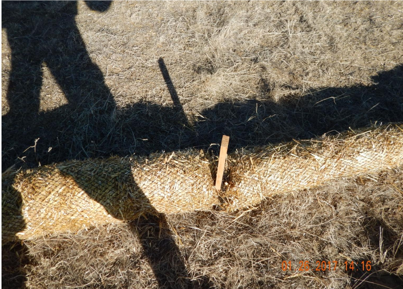
Photo 4. Photo taken from the northwest location. Wattle BMP has not been properly installed by trenching and backfilling the wattle, and wattles have not been overlapped at joints.
