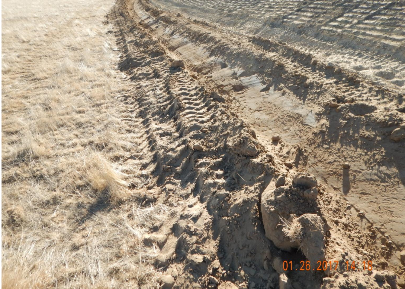
Photo 9. Photo taken from the eastern location, facing South. Berm BMP insufficient and berm not compacted.
