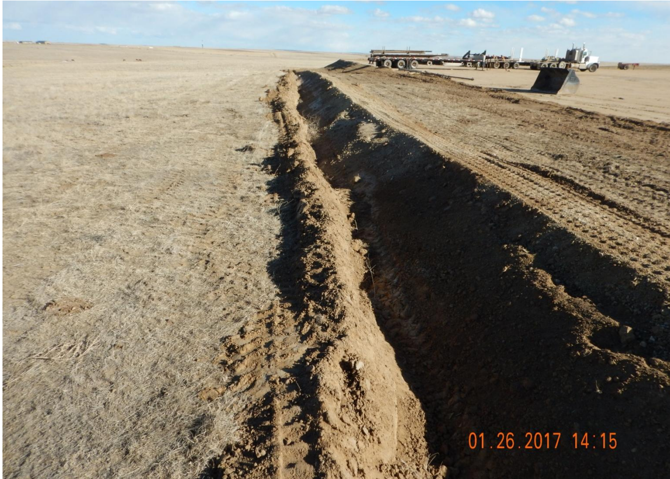
Photo 1. Photo taken from the northwest location, facing East. Berm BMP insufficient and berm not compacted.
