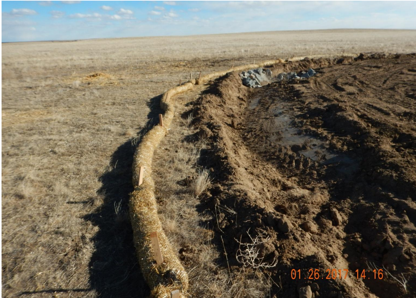
Photo 3. Photo taken from the northwest location, facing East. Berm BMP insufficient and berm not compacted. Wattle BMP has not been properly installed by trenching and backfilling the wattle, and wattles have not been overlapped at joints.
