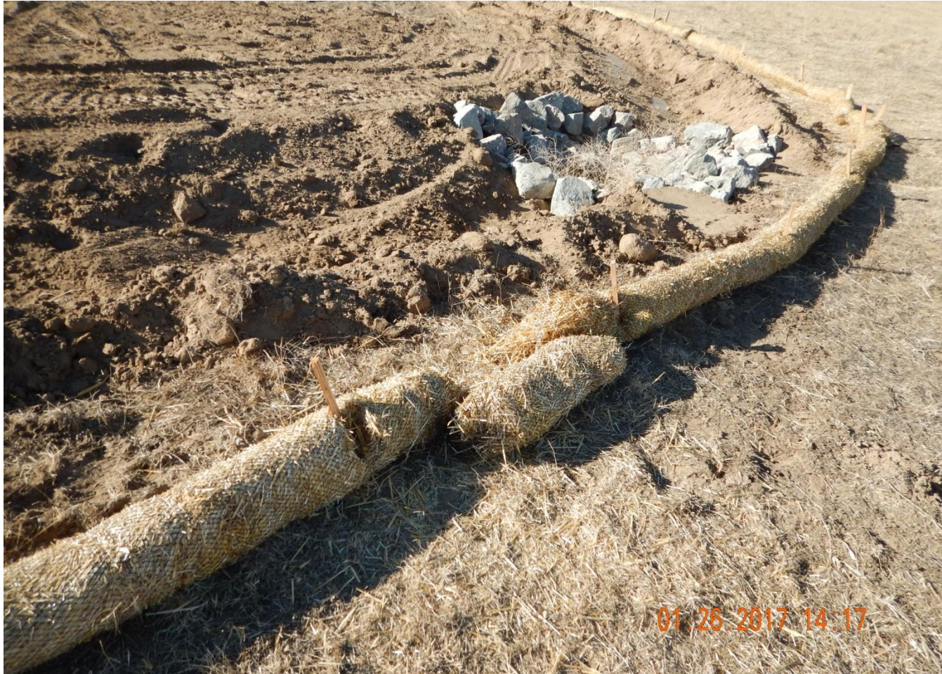
Photo 7. Photo taken from the northwest location, facing West. Wattle BMP has not been properly installed by trenching and backfilling the wattle, and wattles have not been overlapped at joints. A section of wattle is not staked.
