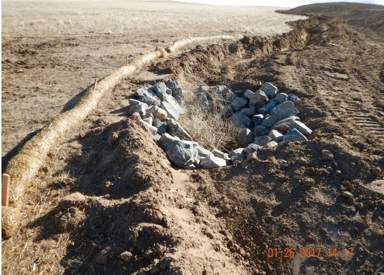
Photo 6. Photo taken from the northwest location, facing towards the sediment trap. Berm BMP insufficient and berm not compacted. Wattle BMP has not been properly installed by trenching and backfilling the wattle, and wattles have not been overlapped at joints.
