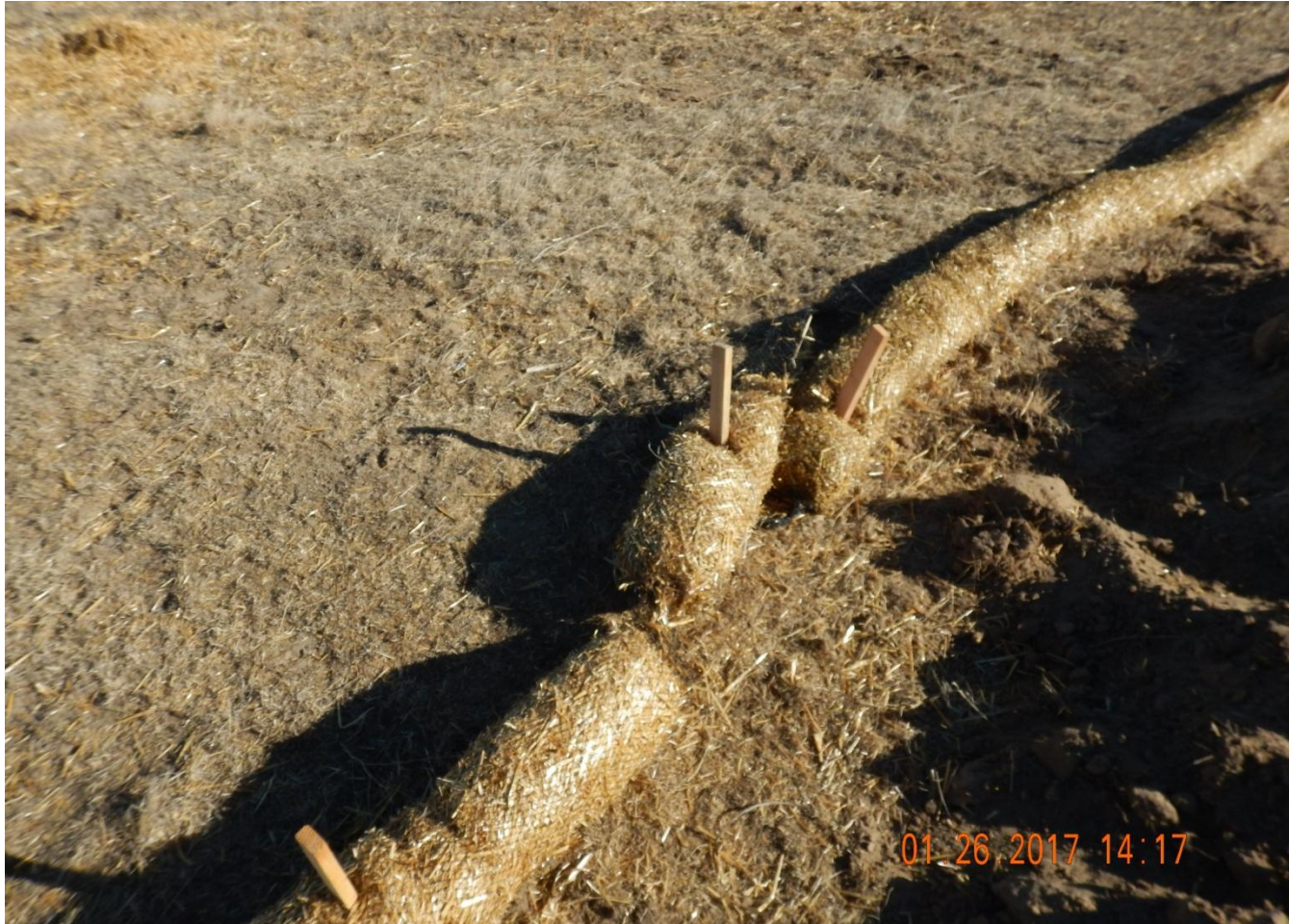
Photo 5. Photo taken from the northwest location. Wattle BMP has not been properly installed by trenching and backfilling the wattle, and wattles have not been overlapped at joints.
