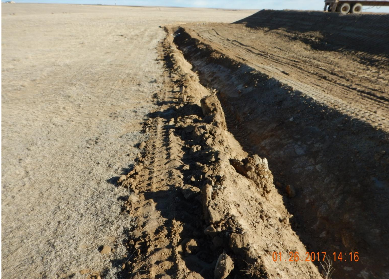
Photo 2. Photo taken from the northern location, facing East. Berm BMP insufficient along perimeter of location and berm not compacted.
