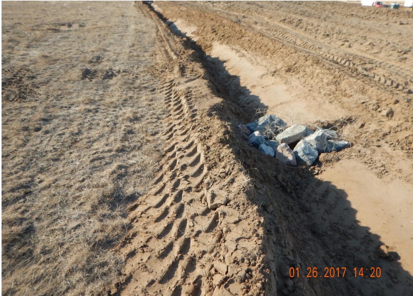
Photo 10. Photo taken from the southern location, facing West. Berm BMP insufficient and berm not compacted. Check dam BMP installed along portions of the perimeter. Appears more rock material could be added to capture sediment.
