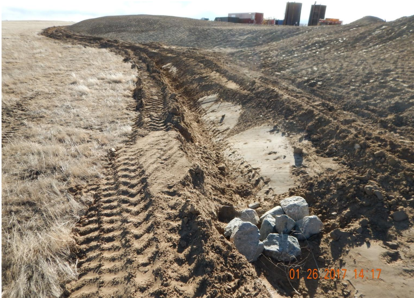
Photo 8. Photo taken from the northwest location, facing South. Berm BMP insufficient and berm not compacted. Check dam BMP installed along portions of the perimeter. Appears more rock material could be added to capture sediment.
