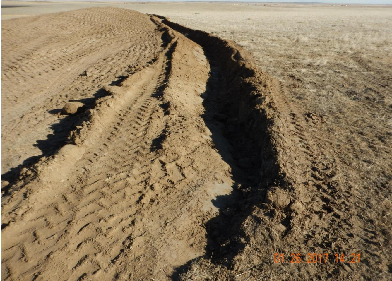
Photo 11. Photo taken from the southwest location, facing East. Berm BMP insufficient and berm not compacted.
