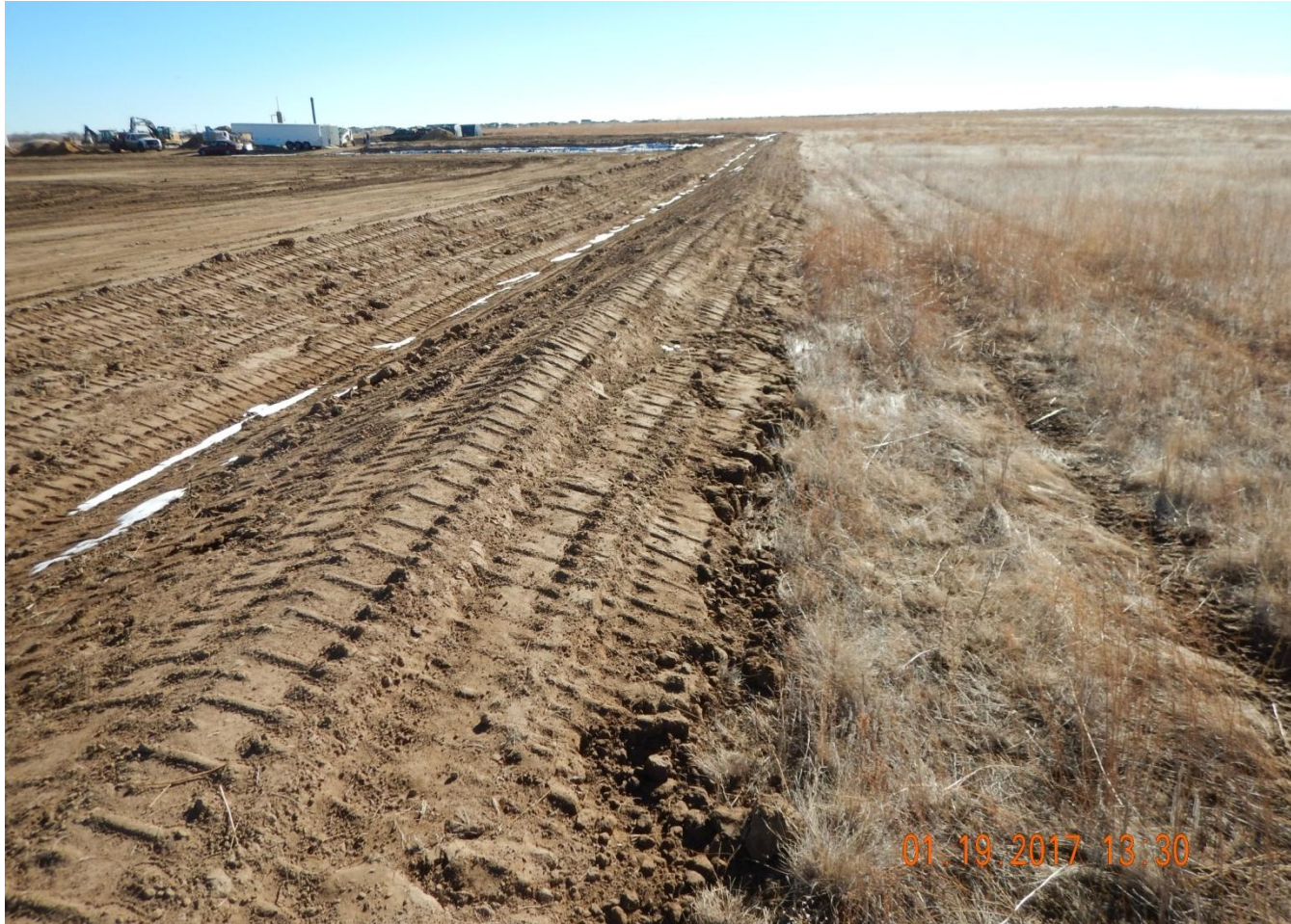
Photo 4. Photo taken from the western location, facing South. Ditch and berm BMP installed around the entire perimeter of the location.
