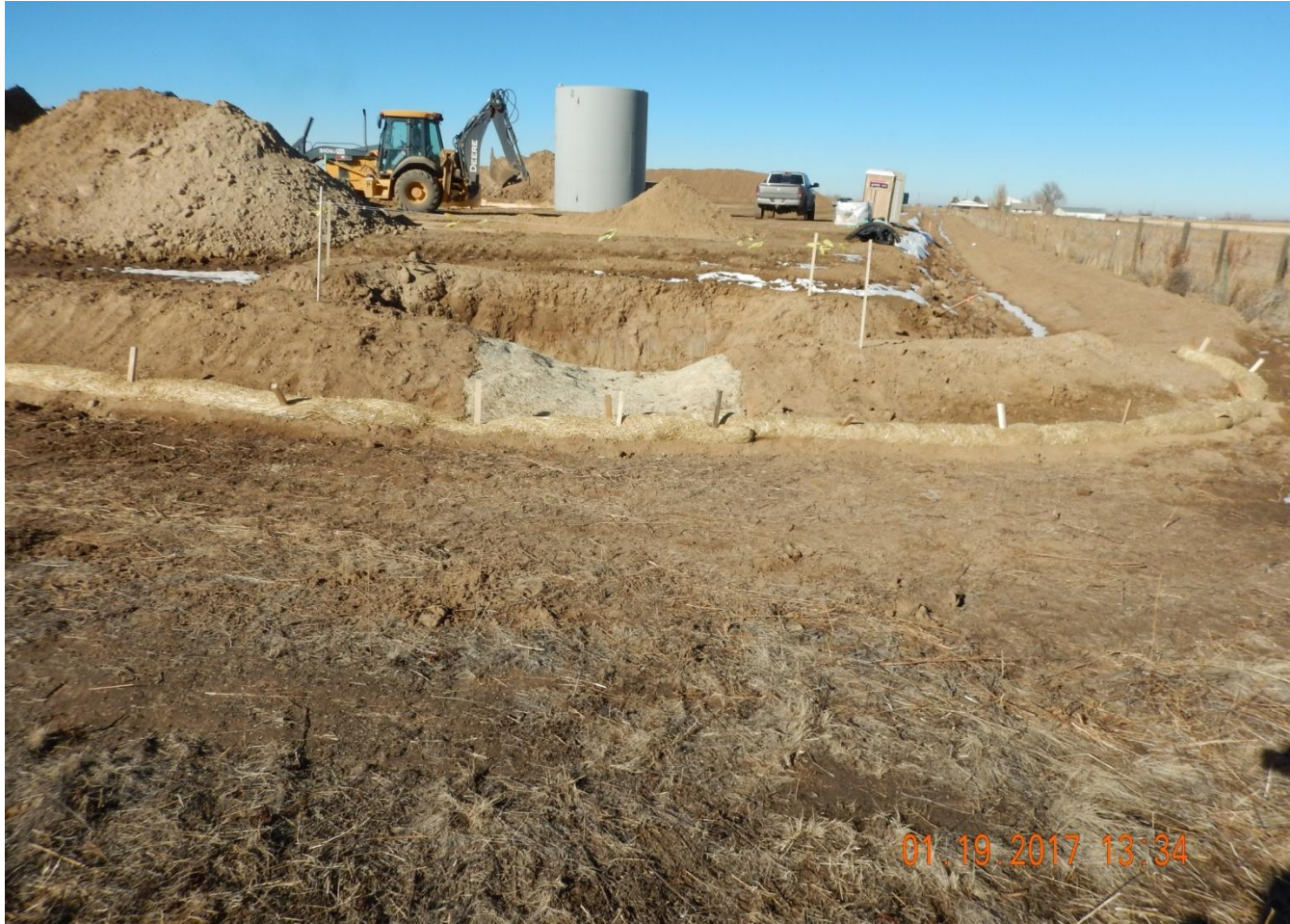
Photo 6. Photo taken from the southeast location, facing North. Ditch and berm BMP installed around the entire perimeter of the location. Sediment trap has been installed with a stabilized outlet.
