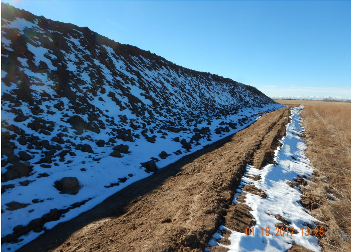
Photo 3. Photo taken from the northern location, facing West, towards the topsoil stockpile. Topsoil stockpile appears steep on the north-facing side and would be difficult for perennial vegetative growth to establish for stabilization. May consider re-contouring when conditions are suitable (i.e., after winter).
