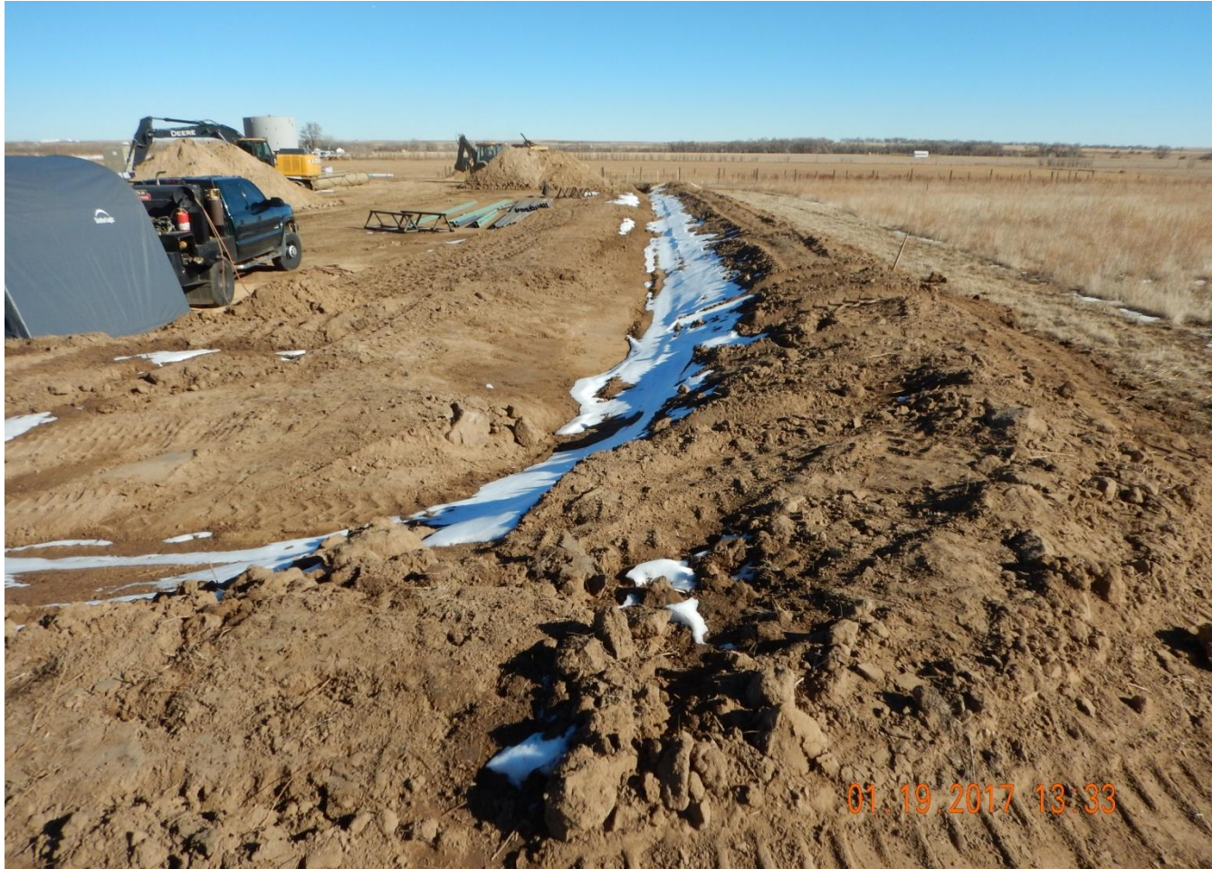
Photo 5. Photo taken from the southwest location, facing East. Ditch and berm BMP installed around the entire perimeter of the location.
