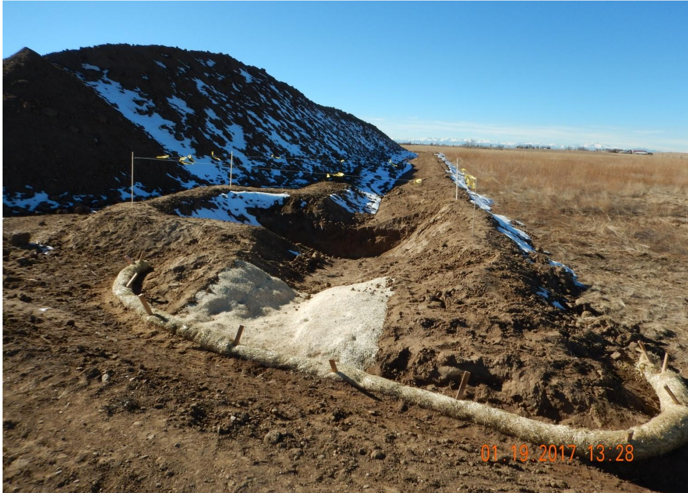
Photo 2. Photo taken from the entrance of location on the westside of the access road, facing West. Ditch and berm BMP installed around the entire perimeter of the location. Sediment trap has been installed with a stabilized outlet.
