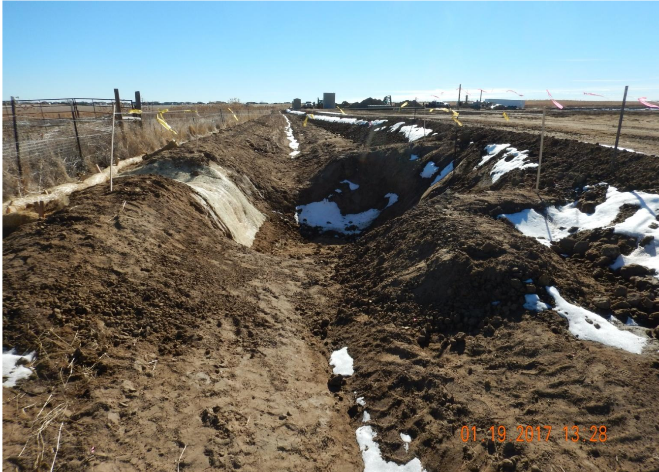
Photo 1. Photo taken from the entrance of location on the eastside of the access road, facing South. Ditch and berm BMP installed around the entire perimeter of the location. Sediment trap has been installed with a stabilized outlet.
