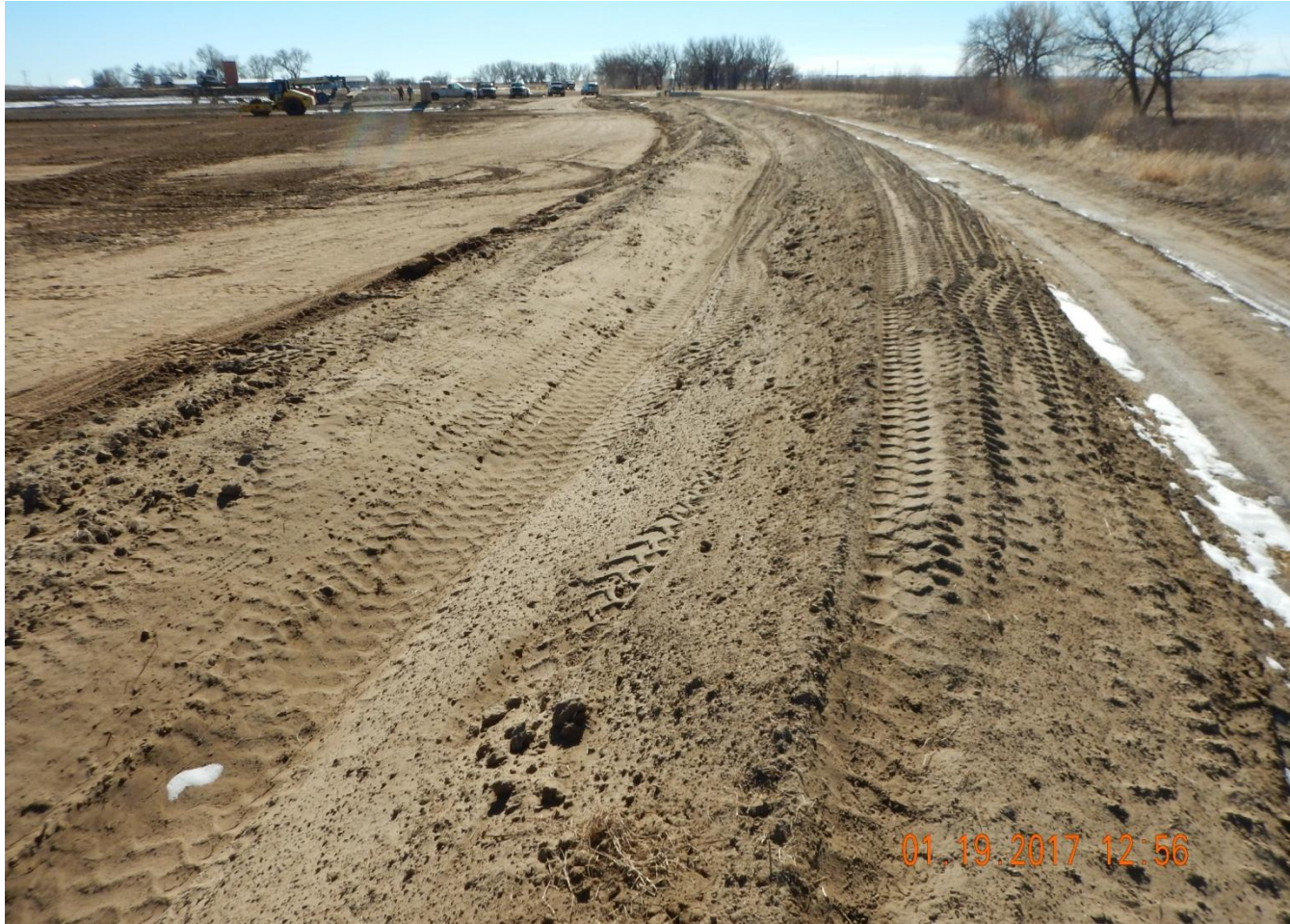
Photo 7. Photo taken from the northwest location, facing South. Ditch and berm BMP installed around the entire perimeter of the location.
