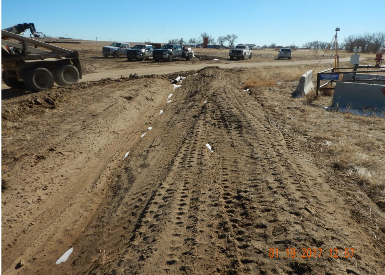
Photo 8. Photo taken from the entrance of location, facing South. Ditch and berm BMP installed around the entire perimeter of the location. Culvert installed in conjunction with ditch.
