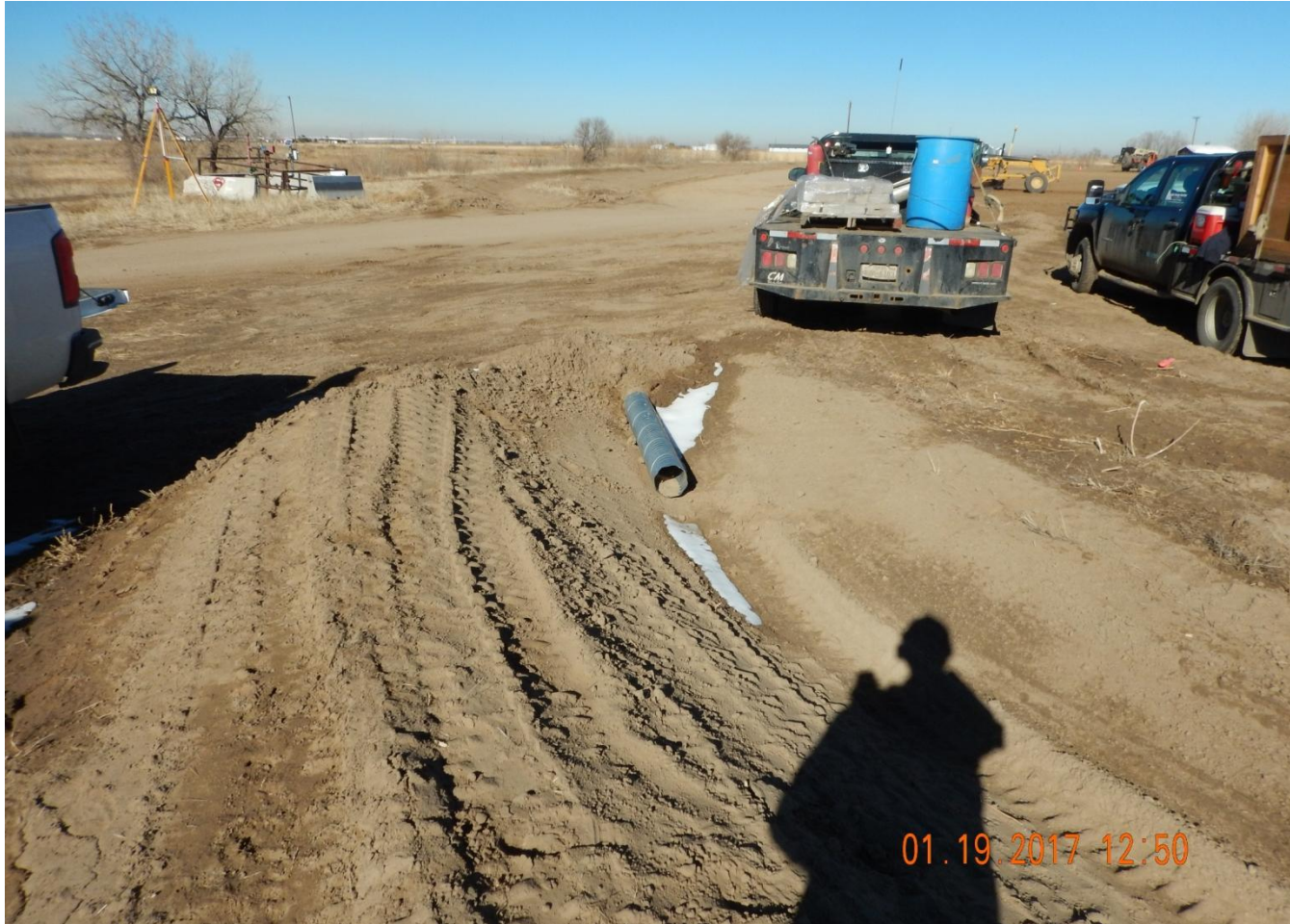
Photo 1. Photo taken from the entrance of location, facing North. Ditch and berm BMP installed around the entire perimeter of the location. Culvert installed in conjunction with ditch.
