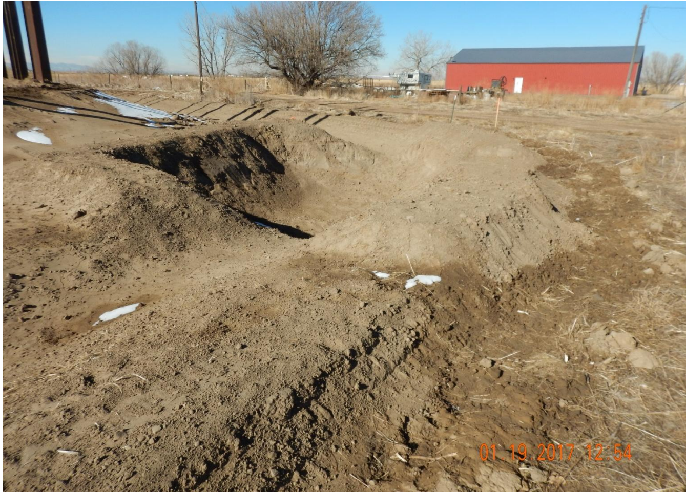
Photo 5. Photo taken from the northeast location, facing North. Sediment trap IN-PROCESS of being constructed.
