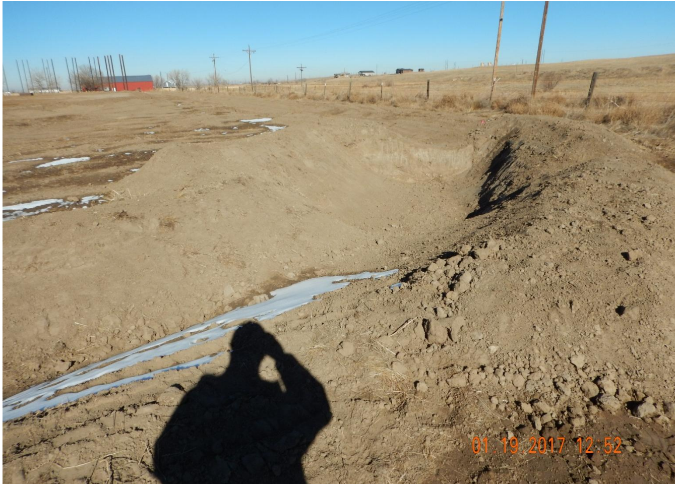
Photo 3. Photo taken from the southeast location, facing North. Sediment trap IN-PROCESS of being constructed.
