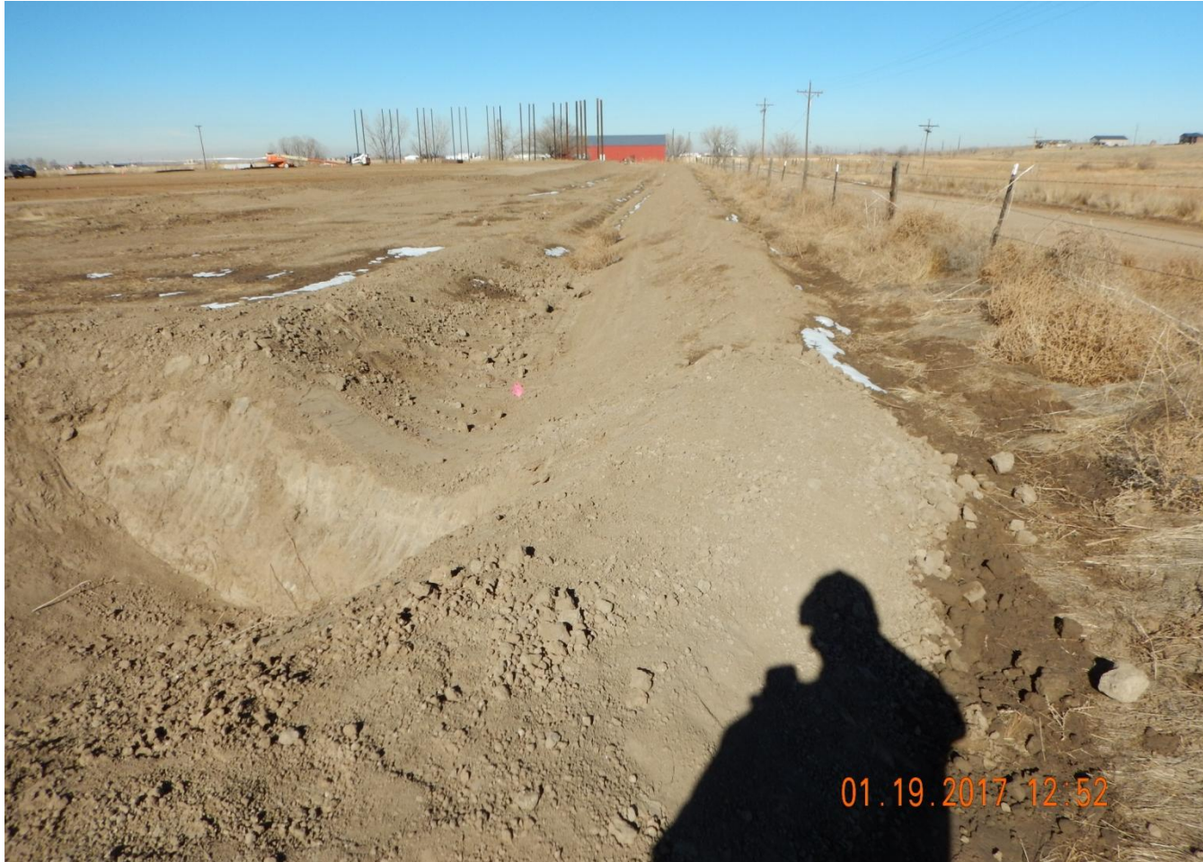
Photo 4. Photo taken from the southeast location, facing North. Ditch and berm BMP installed around the entire perimeter of the location.
