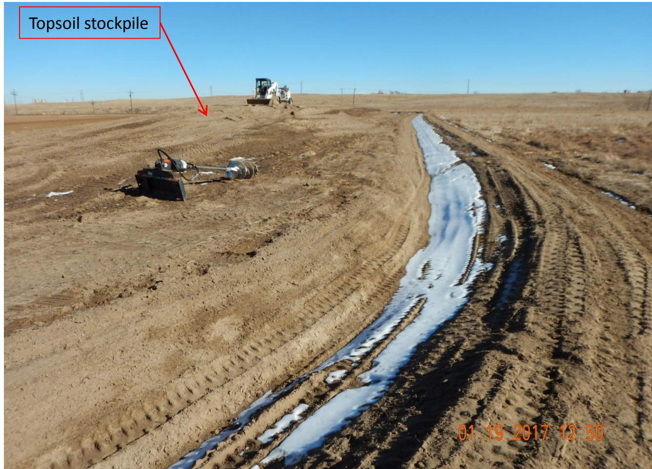
Photo 2. Photo taken from the southwest location, facing East. Ditch and berm BMP installed around the entire perimeter of the location. Topsoil has been salvaged, stored, and temporarily stabilized (i.e., tracked) along the southern perimeter location.
