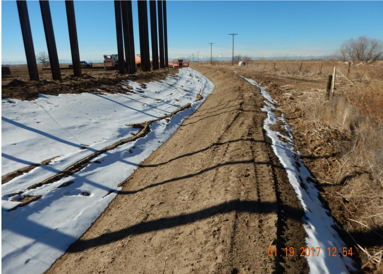
Photo 6. Photo taken from the northeast location, facing West. Ditch and berm BMP installed around the entire perimeter of the location.
