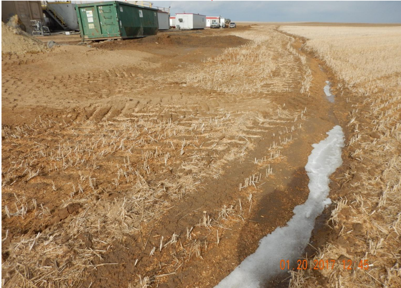
Photo 4. Photo taken from the southeast location, facing North. Insufficient BMP installed around perimeter of location (i.e., swallow ditch) with no, to minimal unconsolidated berm. BMP appears to be in the same condition as the previous inspection.
