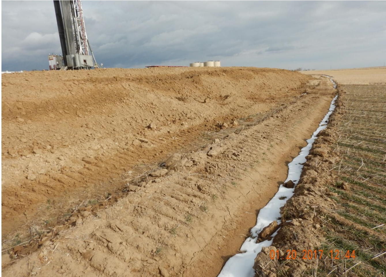
Photo 3. Photo taken from the southern location, facing East. Insufficient BMP installed around perimeter of location (i.e., swallow ditch) with no, to minimal unconsolidated berm. BMP appears to be in the same condition as the previous inspection.
