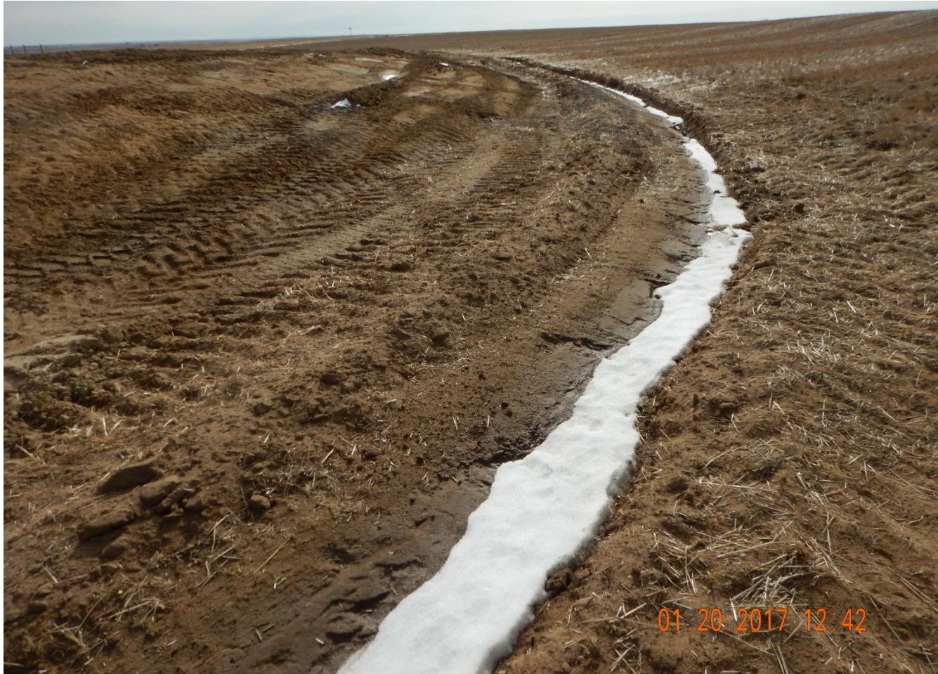
Photo 1. Photo taken from the northwest location, facing South. Insufficient BMP installed around perimeter of location (i.e., swallow ditch) with no, to minimal unconsolidated berm. BMP appears to be in the same condition as the previous inspection.
