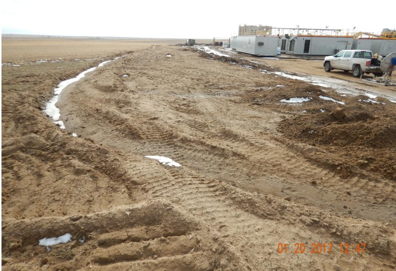
Photo 5. Photo taken from the northeast location, facing South. Insufficient BMP installed around perimeter of location (i.e., swallow ditch) with no, to minimal unconsolidated berm. BMP appears to be in the same condition as the previous inspection.
