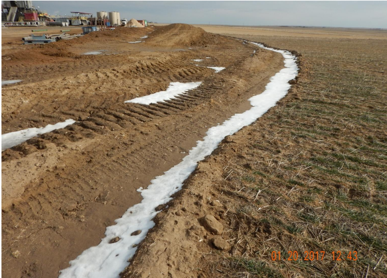
Photo 2. Photo taken from the southwest location, facing East. Insufficient BMP installed around perimeter of location (i.e., swallow ditch) with no, to minimal unconsolidated berm. BMP appears to be in the same condition as the previous inspection.
