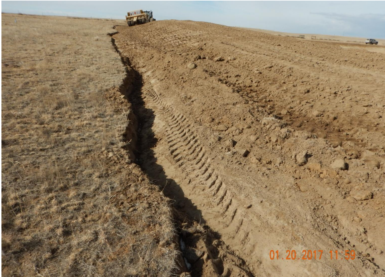
Photo 4. Photo taken from the northern location, facing West. Insufficient BMP installed around perimeter of location. Topsoil stockpile has been tracked and stabilized but that alone is not sufficient to control potential erosion.
