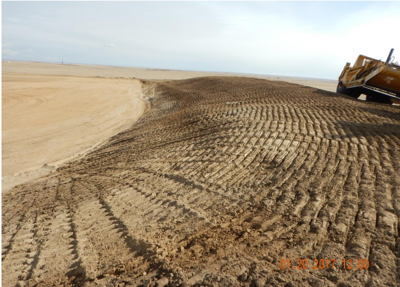
Photo 6. Photo taken from the southwest location, facing East. Topsoil stockpile has been salvaged and stored along the southern perimeter of location. May suggest marking spoil and topsoil stockpiles to aid in identifying stockpiles for future reference.
