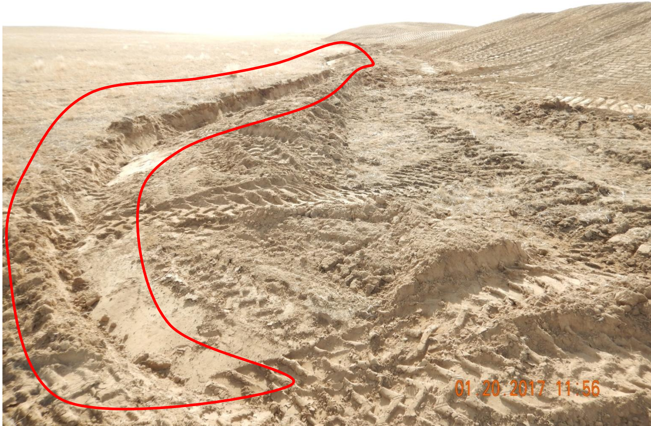
Photo 2. Photo taken from the northeast location, facing South. Insufficient BMP installed around perimeter of location (i.e., swallow ditch). Equipment traffic should be kept off BMPs to ensure they function properly.
