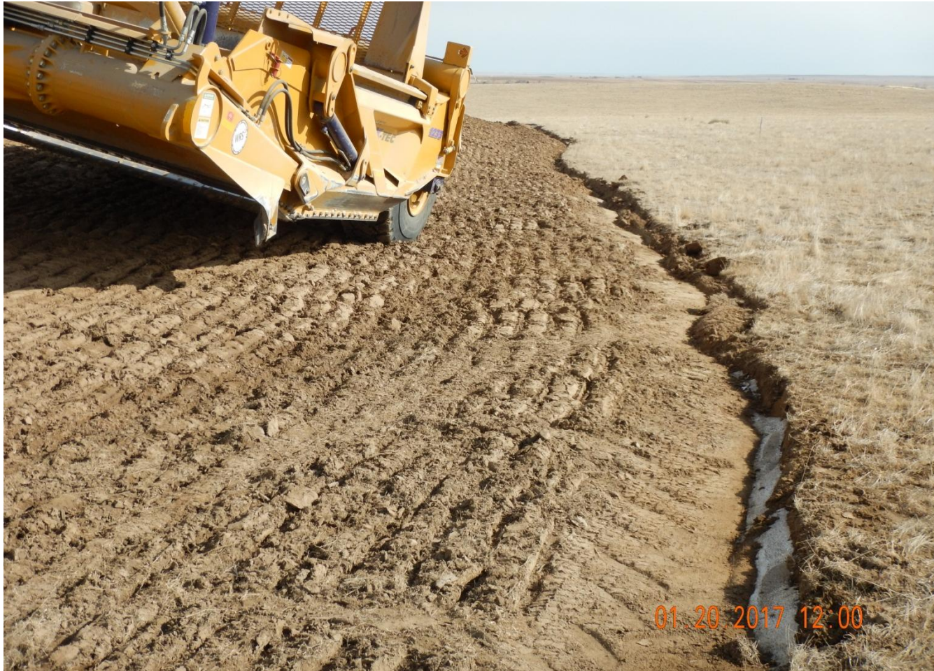
Photo 5. Photo taken from the southwest location, facing East. Insufficient BMP installed around perimeter of location. Topsoil stockpile has been tracked and stabilized but that alone is not sufficient to control potential erosion.
