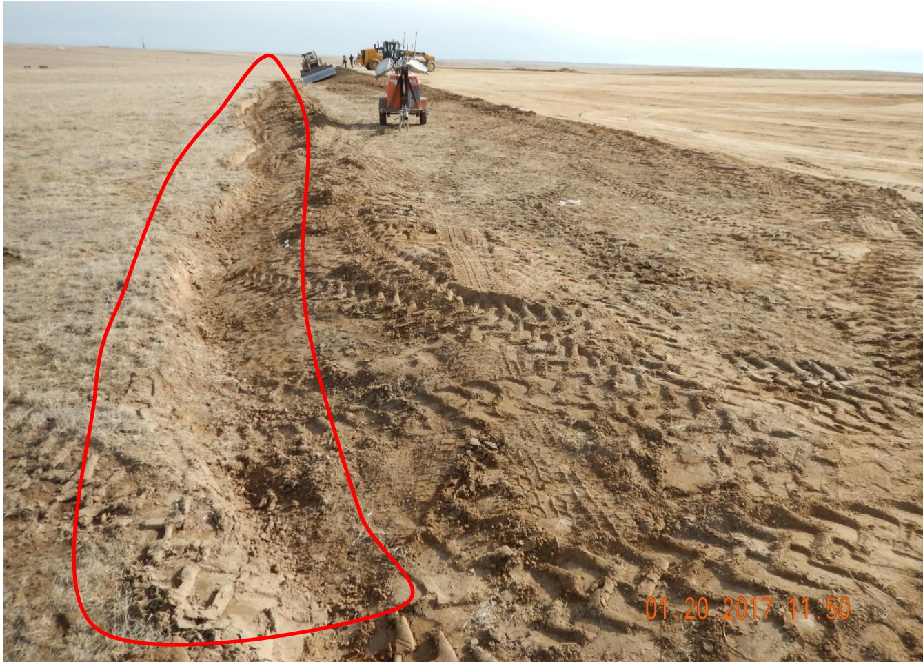
Photo 1. Photo taken from the northwest location, facing East. Insufficient BMP installed around perimeter of location (i.e., swallow ditch) and equipment traffic should be kept off BMPs to ensure they function properly.
