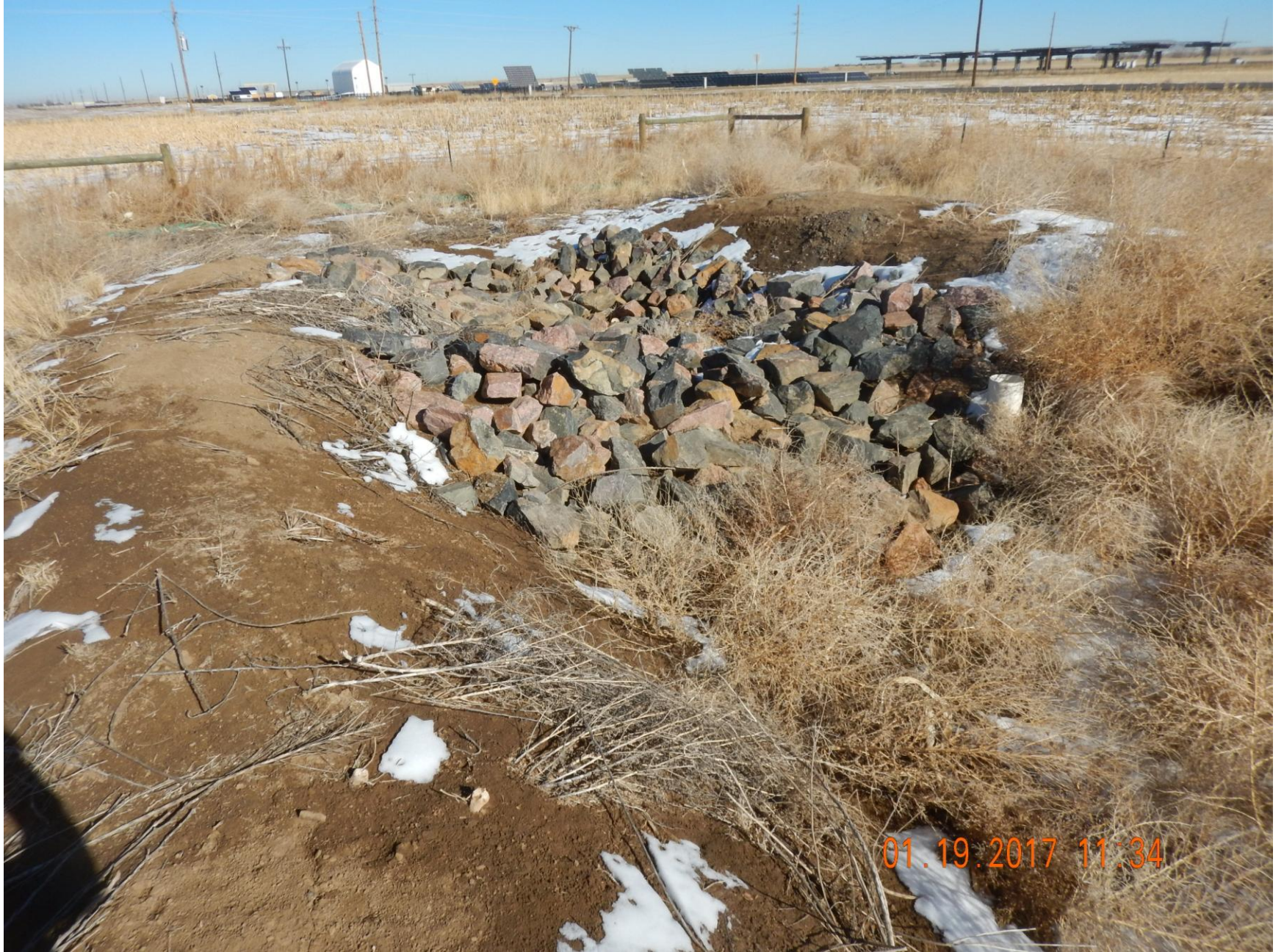
Figure 13: Photo taken from the northeast end of the location, facing northeast. Photo shows sediment trap.
