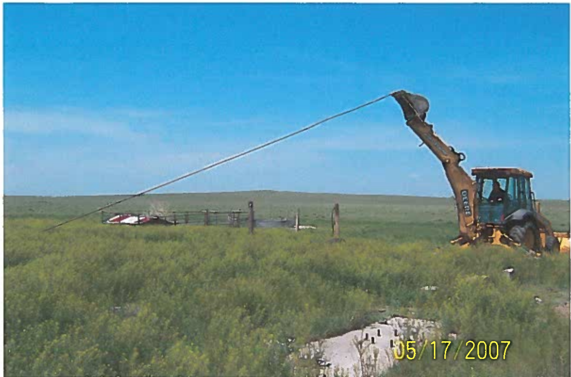
Photo 5: Some piping was shallow enough that the whole line was removed.
