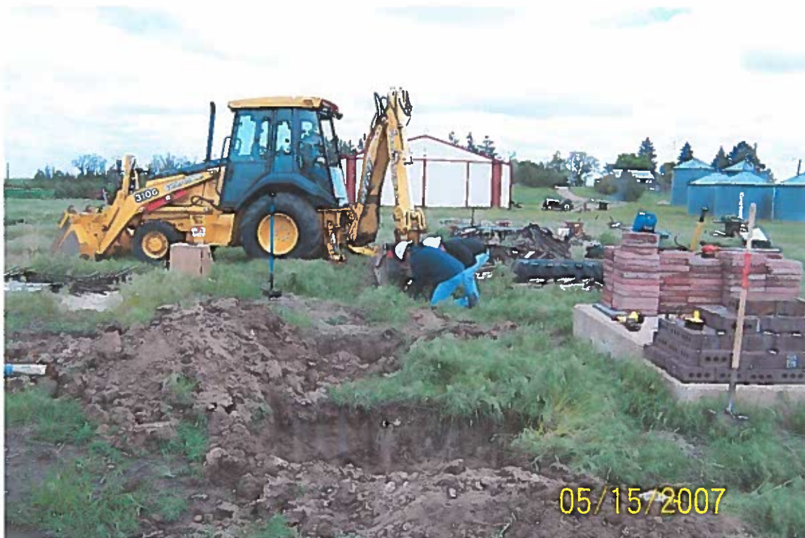
Photo 1: Exposed risers were dug up for removal.
