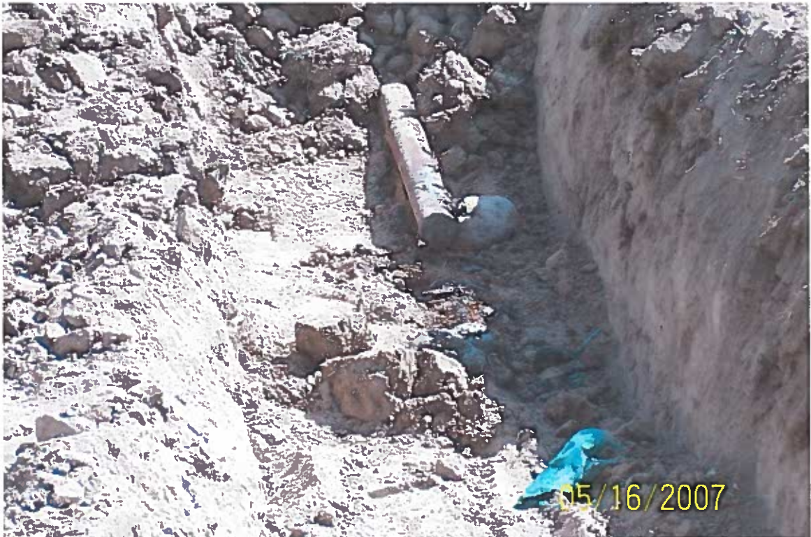
Photo 3: Remaining pipe ends were sealed with non-shrinking grout.
