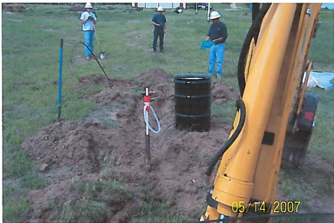
Photo 4: The product was pumped into a 55-gallon drum.
