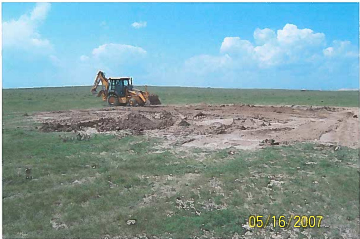
Photo 4: Dirt pit was backfilled after pipe removal.
