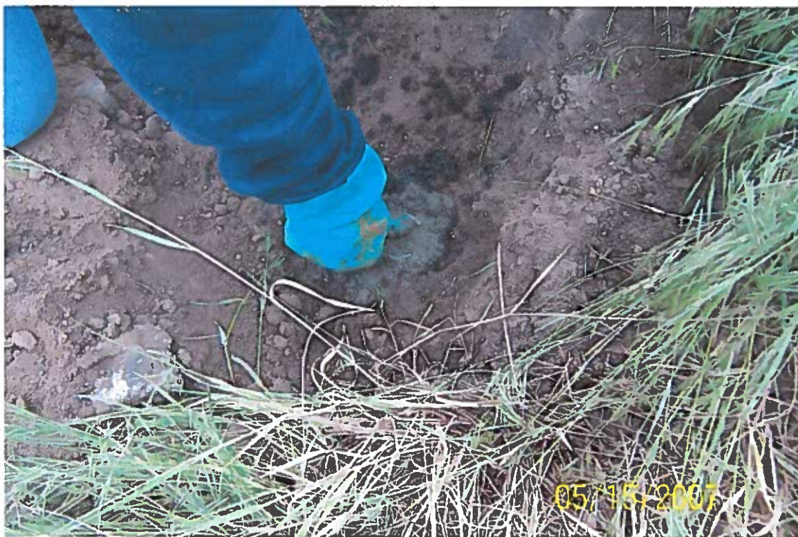
Photo 2: Remaining piping was sealed with non-shrinking grout.
