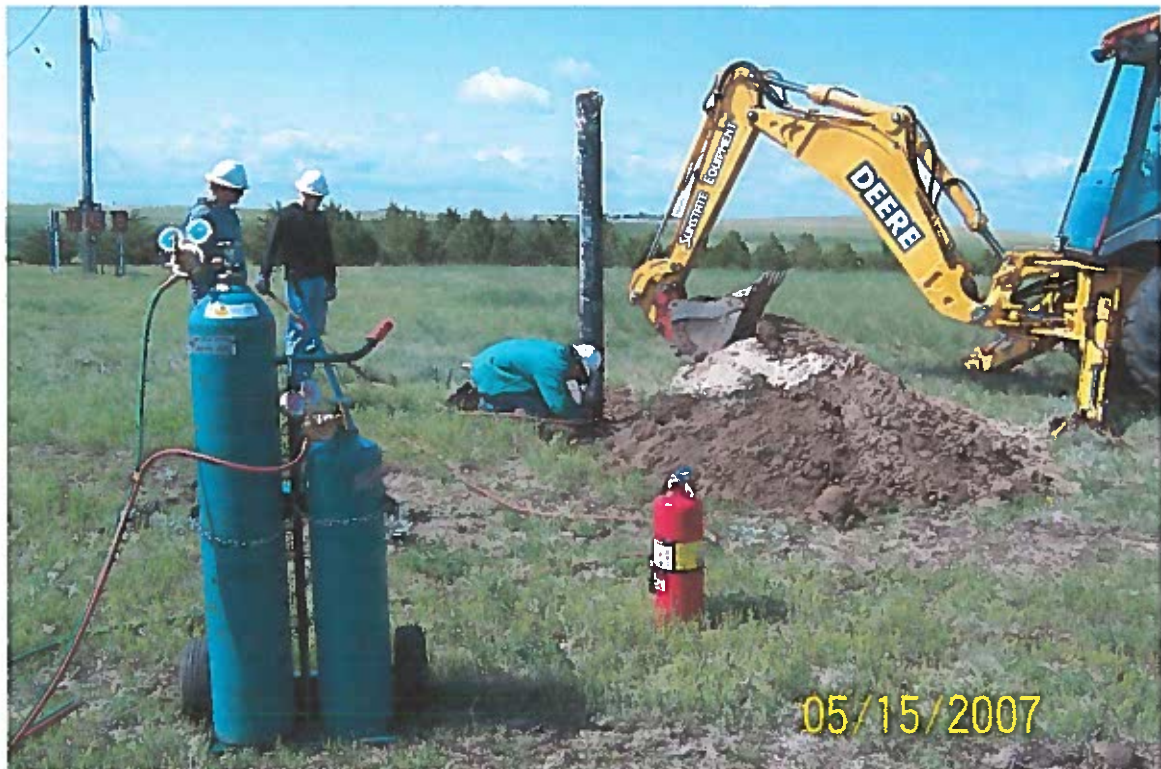
Photo 5: Cutting torch was used to cut off tie down anchors.
