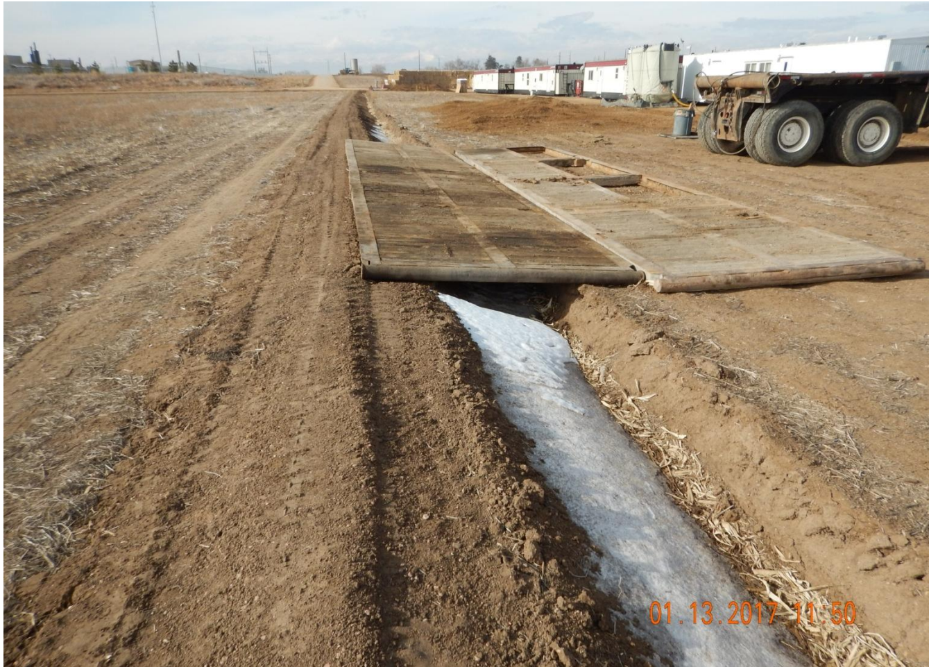
Photo 6. Photo taken from the southern location, facing West. Operator using ramps to access location with equipment to mitigate impacts to stormwater BMPs.
