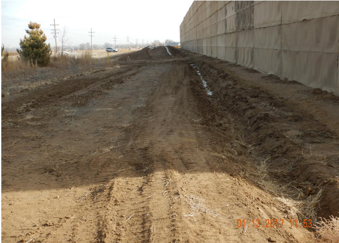
Photo 8. Photo taken from the northwest location, facing East. Ditch and berm installed around the entire perimeter of the location.
