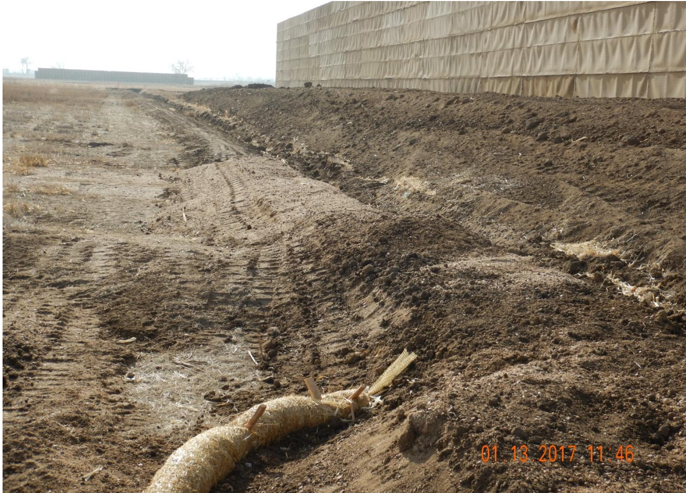
Photo 3. Photo taken from the northeast location, facing South. Ditch and berm installed around the entire perimeter of the location. Also, topsoil stockpile stored along eastern and northern perimeter of location.
