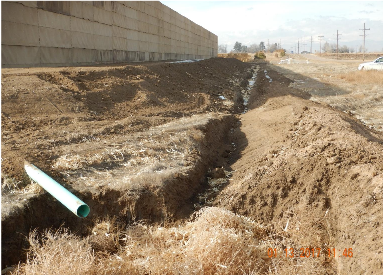
Photo 2. Photo taken from the northeast location, facing West. Ditch and berm installed around the entire perimeter of the location. Also, topsoil stockpile stored along northern and eastern perimeter of location.
