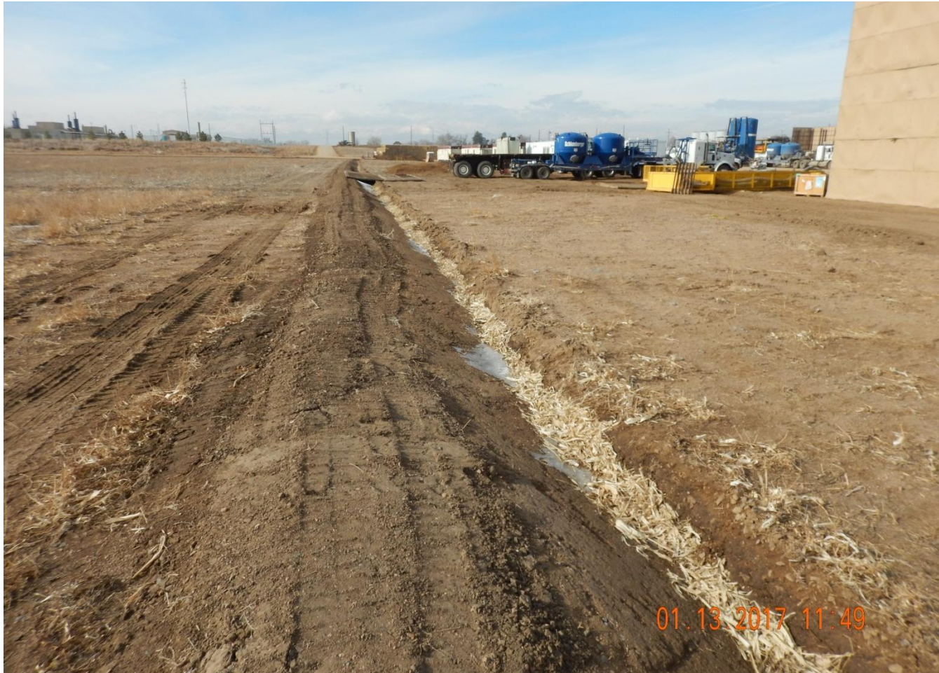
Photo 5. Photo taken from the southeast location, facing West. Ditch and berm installed around the entire perimeter of the location.
