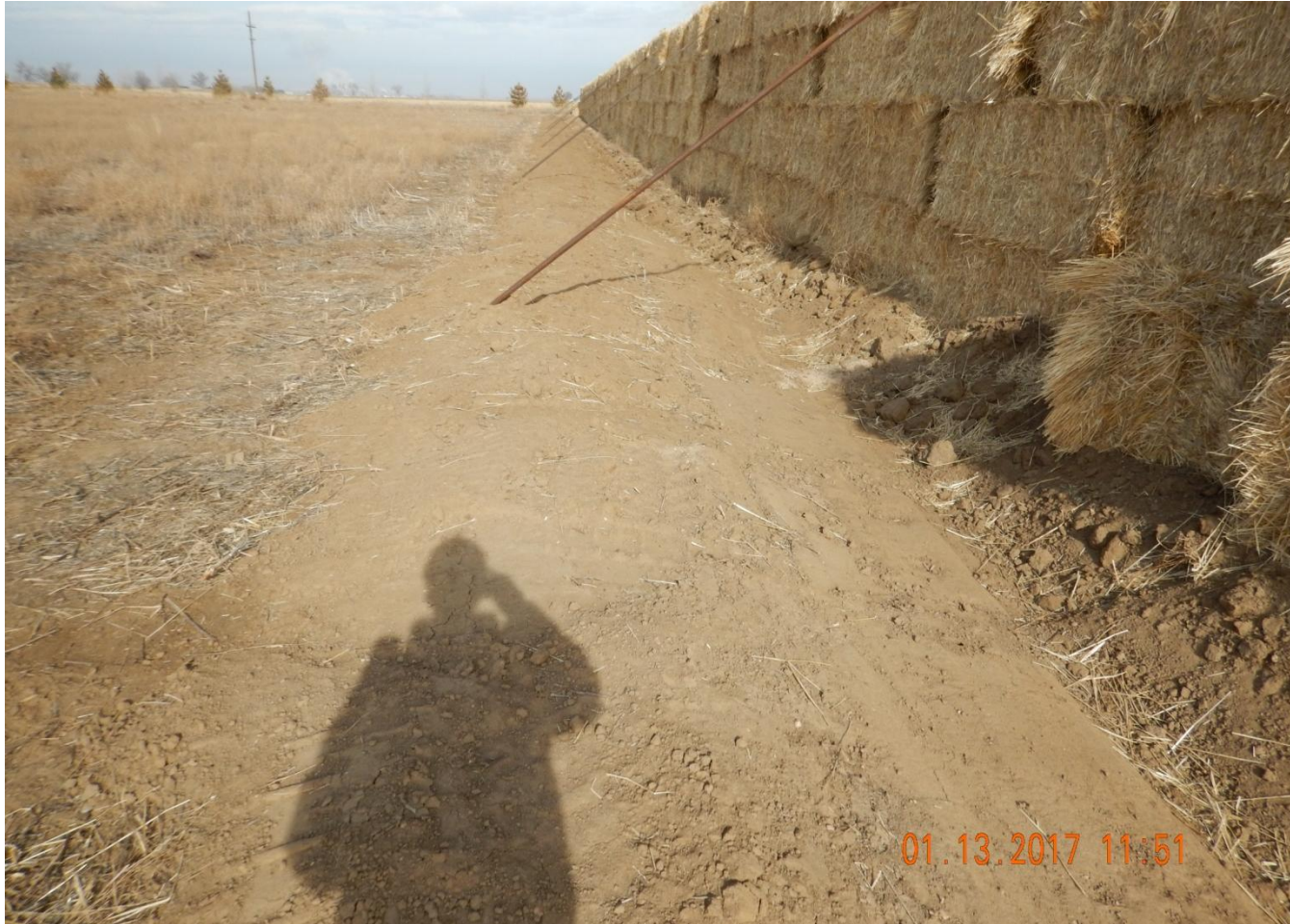
Photo 7. Photo taken from the southwest location, facing North. Ditch and berm installed around the entire perimeter of the location.
