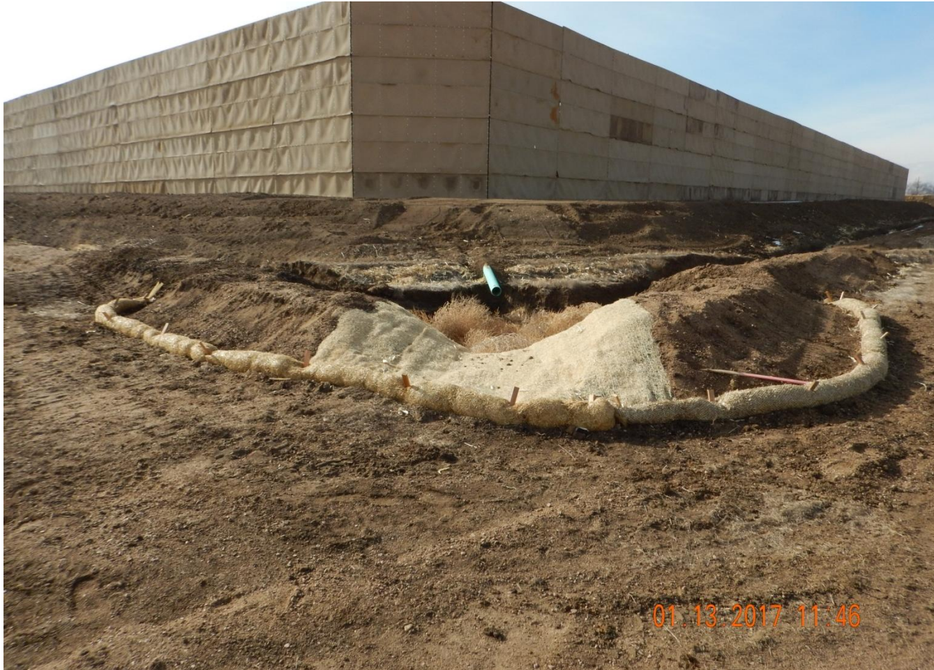
Photo 1. Photo taken from the northeast location, facing Southwest, towards the sediment trap.
