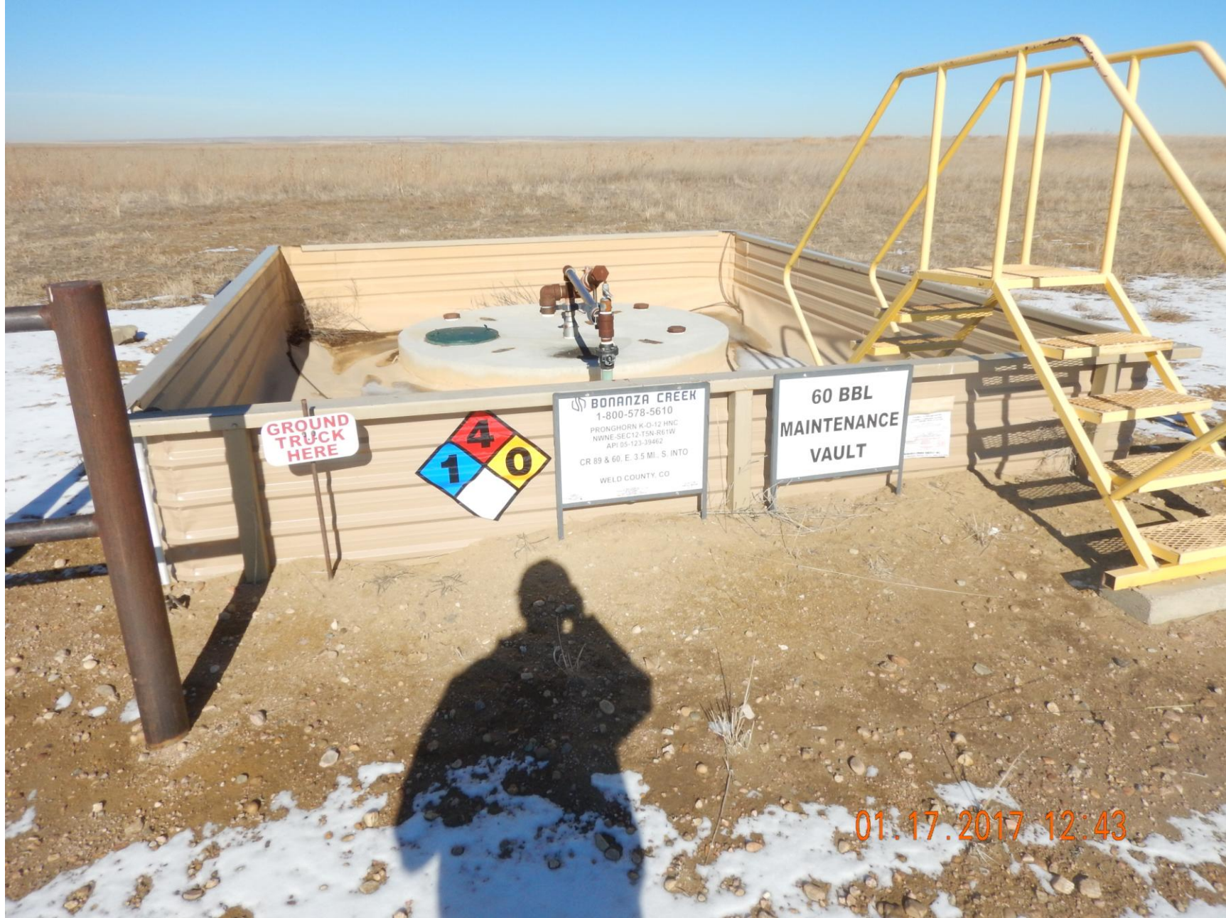
Figure 2: Photo taken from the north end of the location, facing north. Photo shows below ground 60 bbl “maintenance vault”
