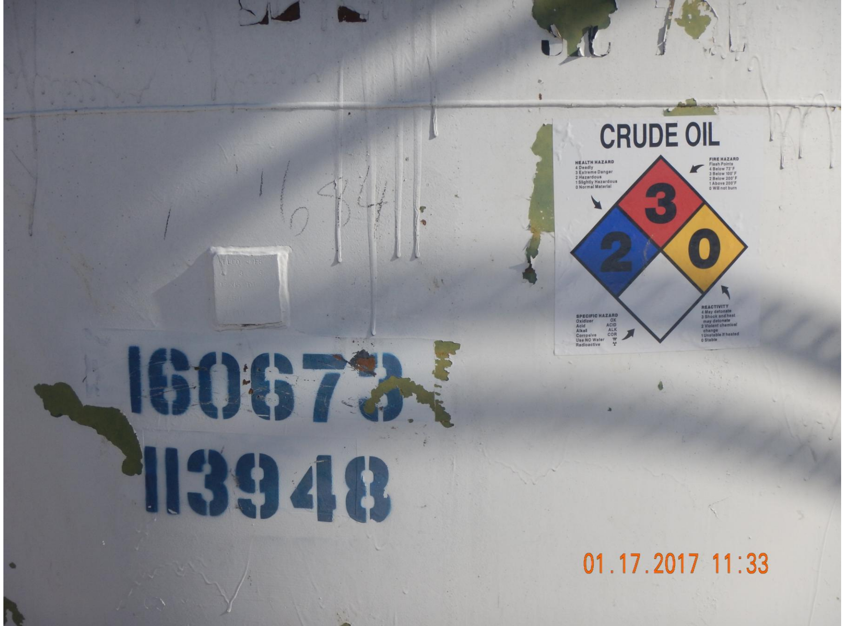
Figure 21: Photo taken from the northern tank. Photo shows a placard has been placed on the tank since inspection doc. #684901990. However tank missing 1) Name of operator, 2) Operator's emergency contact number and 3) Tank capacity.
