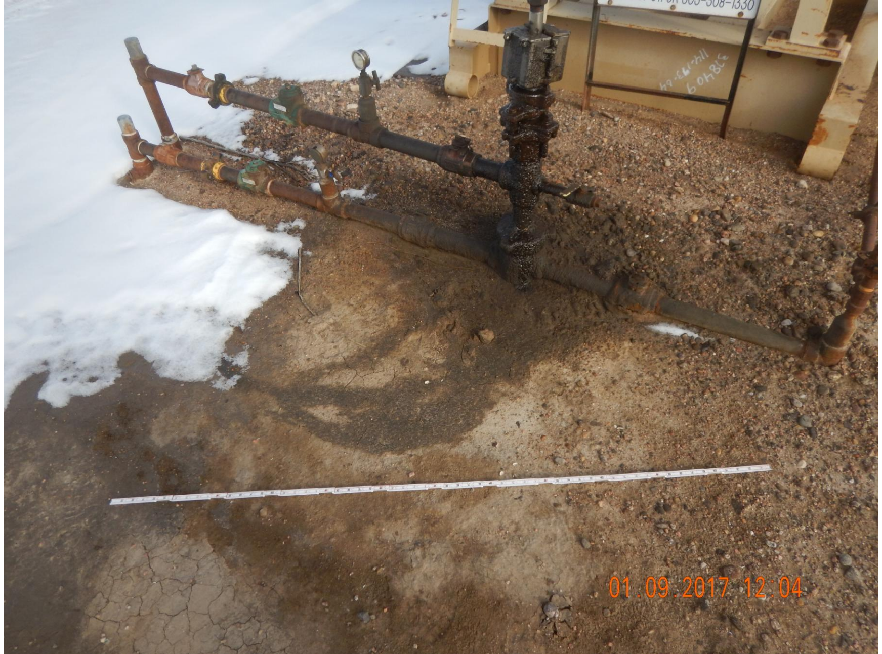
Figure 15: Photo taken at the well head. Photo shows discolored soil. Discolored soil appears to be being transported away from well via stormwater. Soil will need to be cleaned. 6 foot measuring stick for reference.
