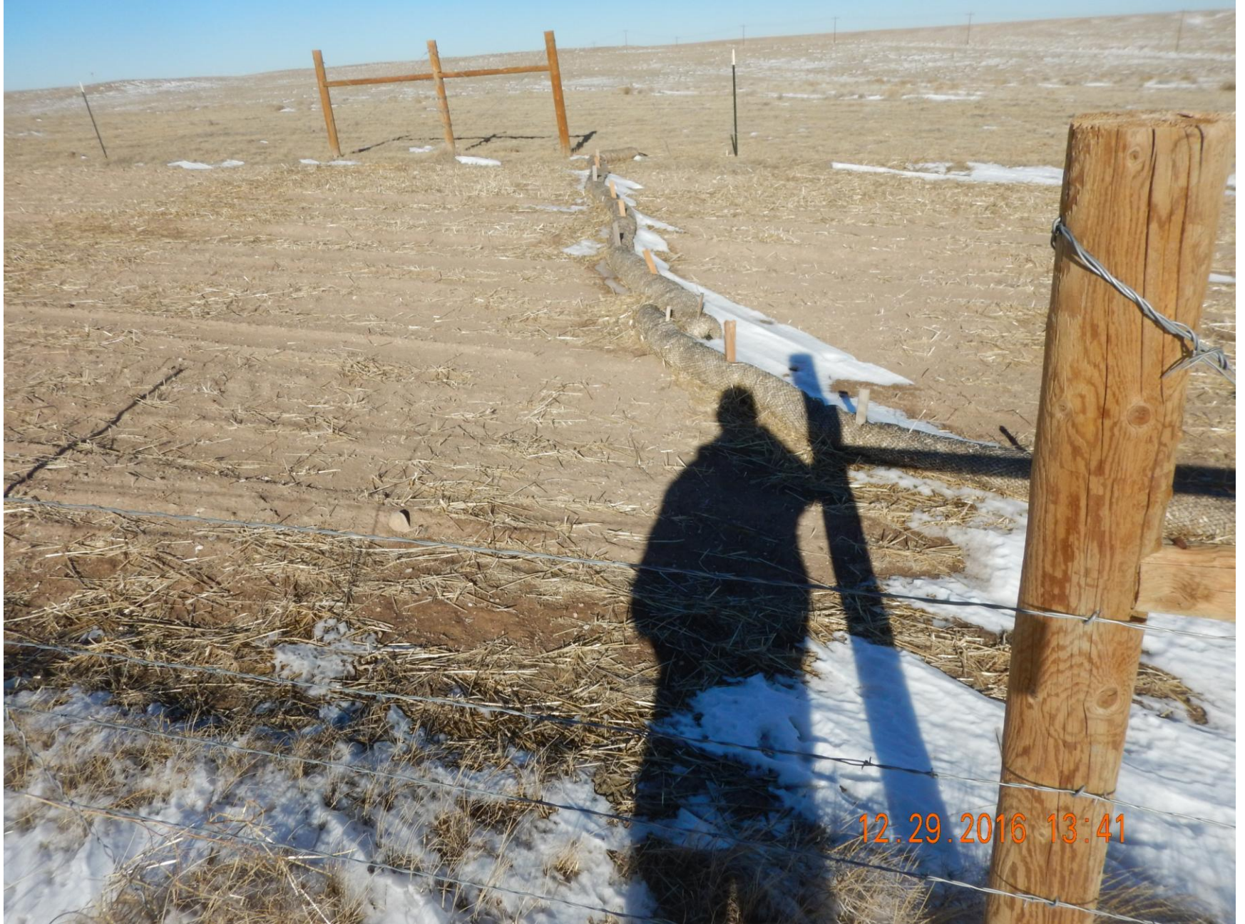
Figure 3: Photo taken from the access road, south of the location, facing east. Photo shows straw wattles used as a stormwater and sediment control BMP.
