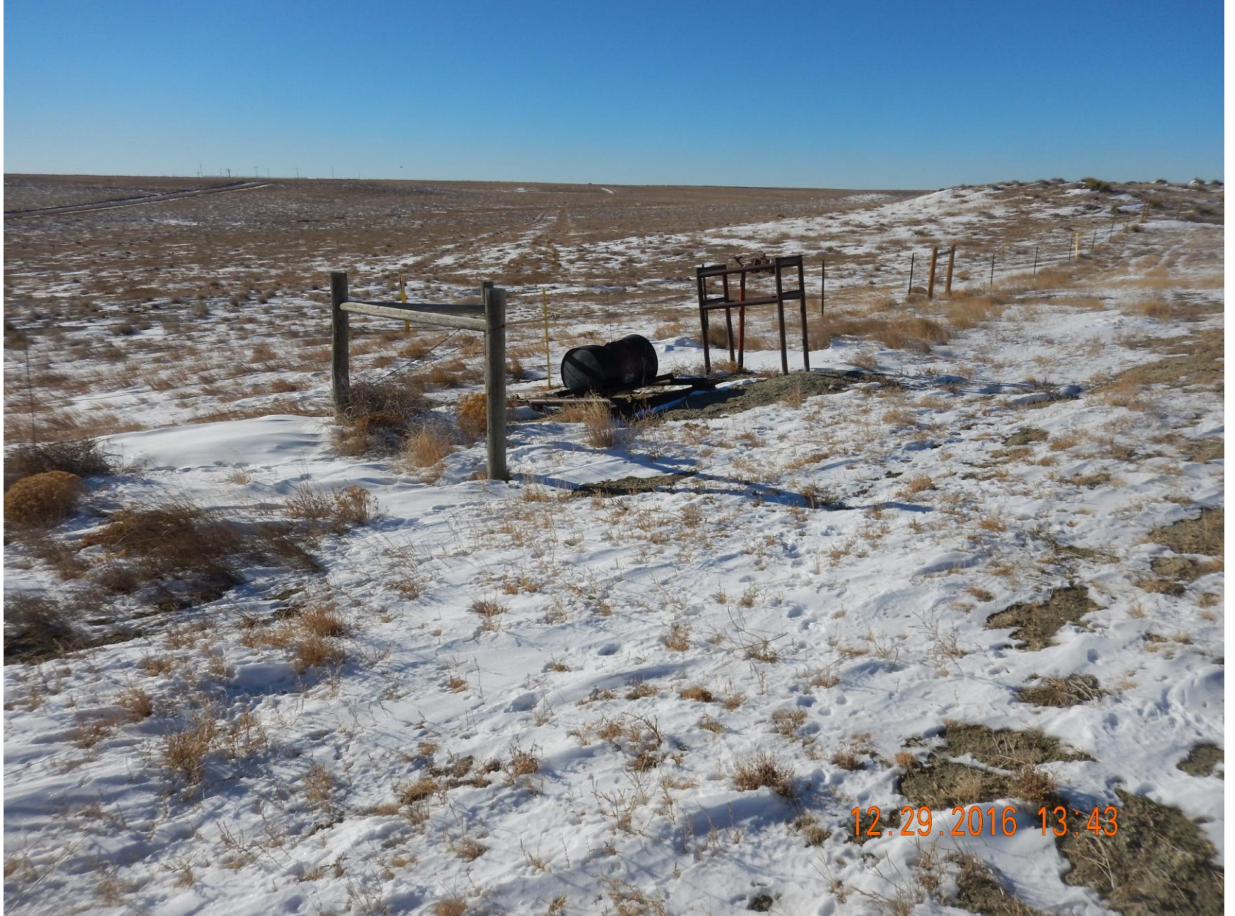
Figure 7: Photo taken from the south end of the location, facing west. Photo shows pipe riser equipment and trash (barrel) remain on location. Insp. Doc. # 682500503 required operator to remove this equipment and trash.
