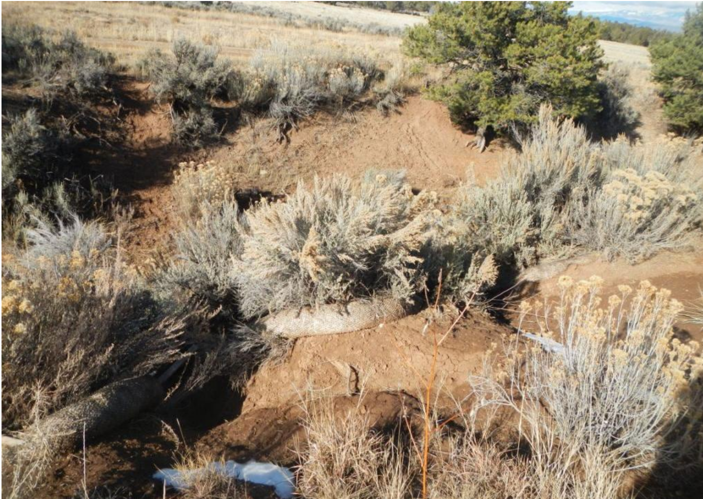
Photo 7. View of area along the western edge of the project area where wattles have failed and additional stormwater controls are needed.
