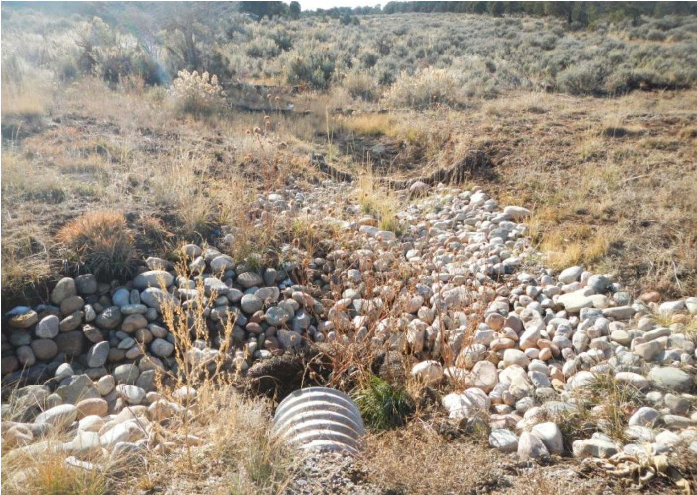
Photo 6. View of cobble armouring installed around the culvert near the entrance of the project area.
