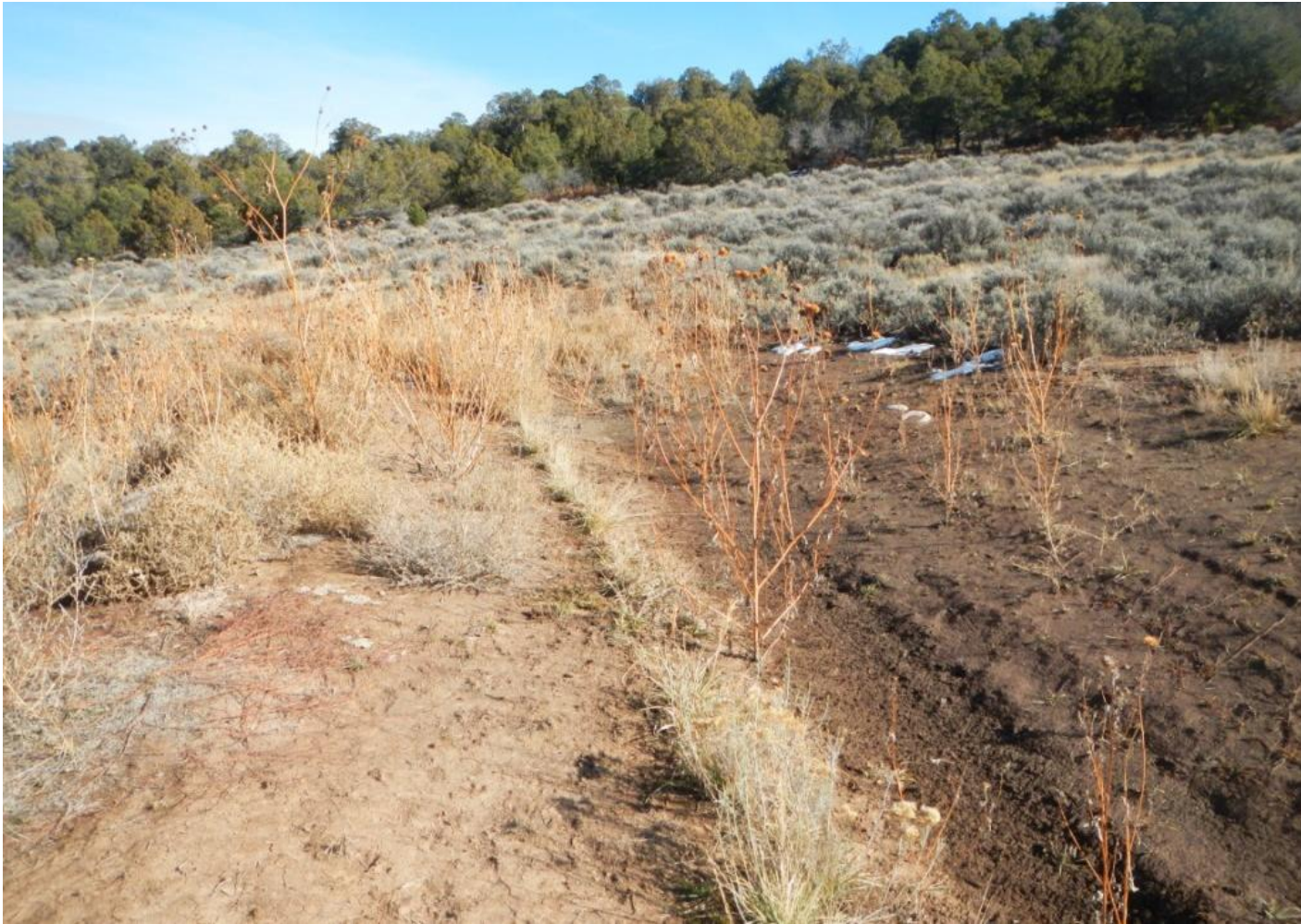
Photo 4. View of area in the southeastern portion of the project area where erosional channels and tunneling have been repaired.
