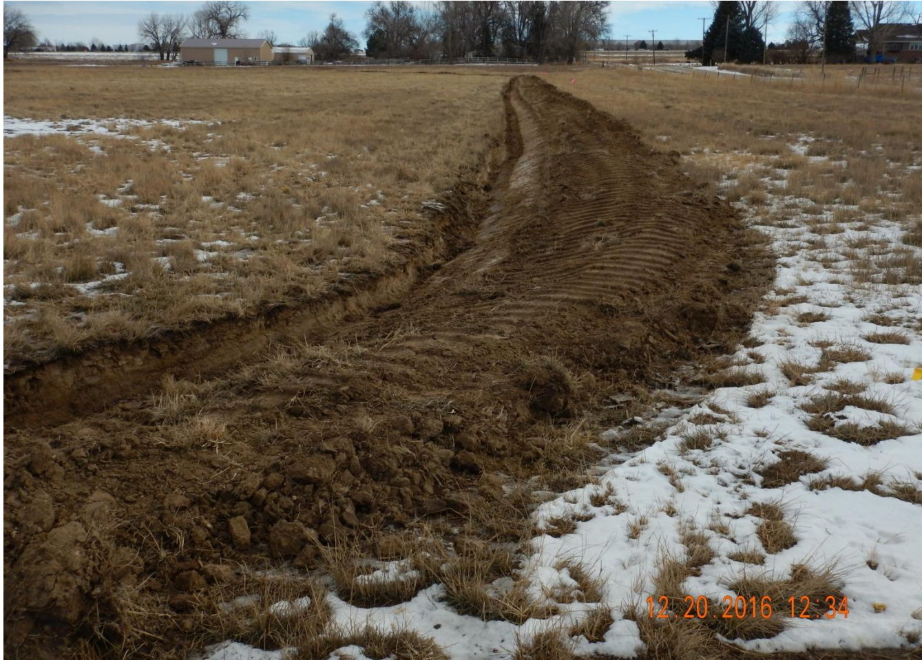
Photo 1. Photo taken from the southwest location, facing East. Ditch and berm installed around the entire perimeter of the location. Operator said berms will be further compacted.
