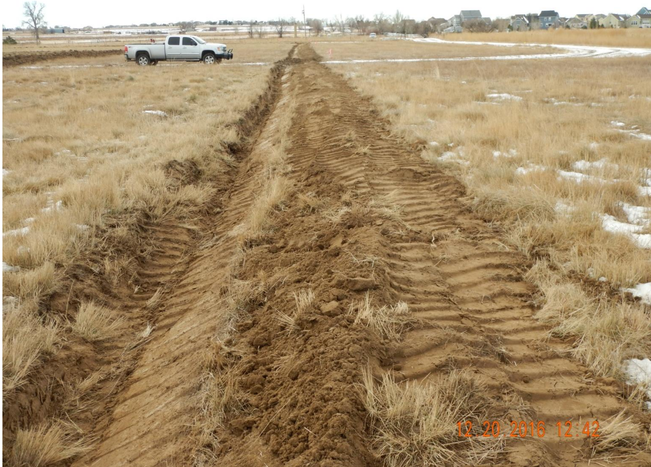
Photo 5. Photo taken from the northwest location, facing South. Ditch and berm installed around the entire perimeter of the location. Operator said berms will be further compacted.
