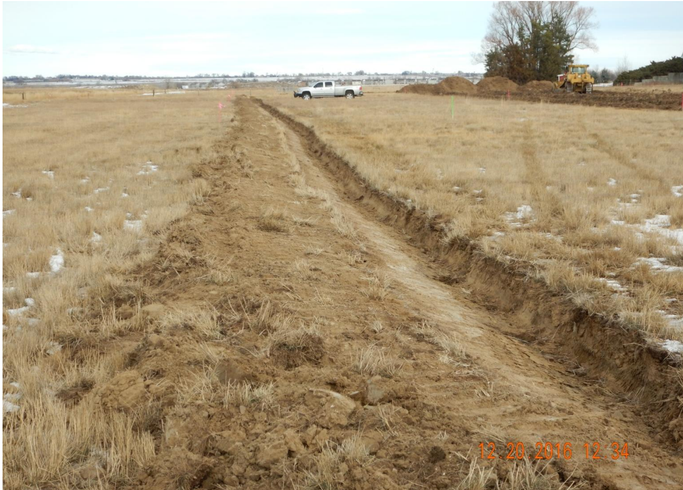
Photo 2. Photo taken from the southwest location, facing North. Ditch and berm installed around the entire perimeter of the location. Operator said berms will be further compacted.
