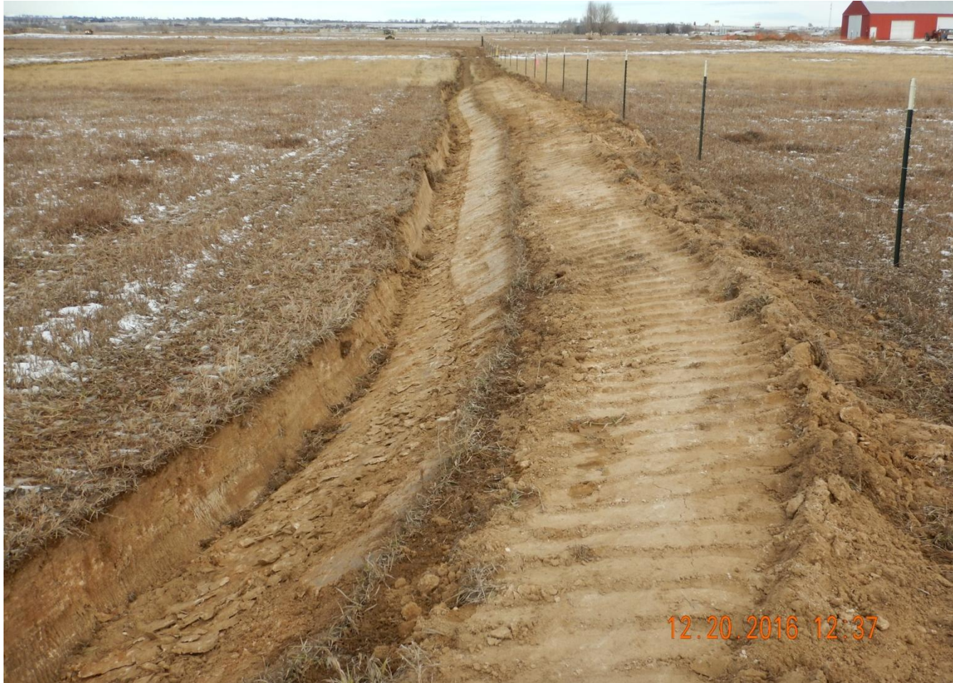
Photo 3. Photo taken from the southeast location, facing North. Ditch and berm installed around the entire perimeter of the location. Operator said berms will be further compacted.
