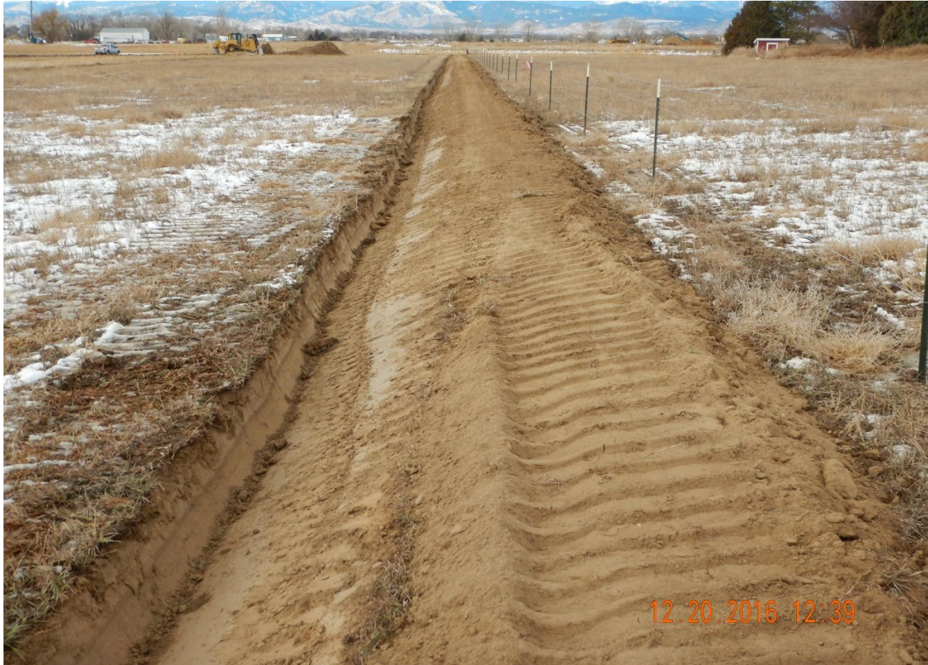
Photo 4. Photo taken from the northeast location, facing West. Ditch and berm installed around the entire perimeter of the location. Operator said berms will be further compacted.
