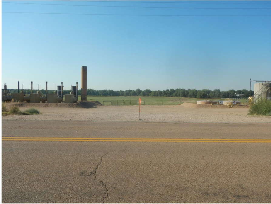
PHOTOGRAPH OF AG 26-32 ACCESS ROAD - CAMERA ANGLE SOUTH
