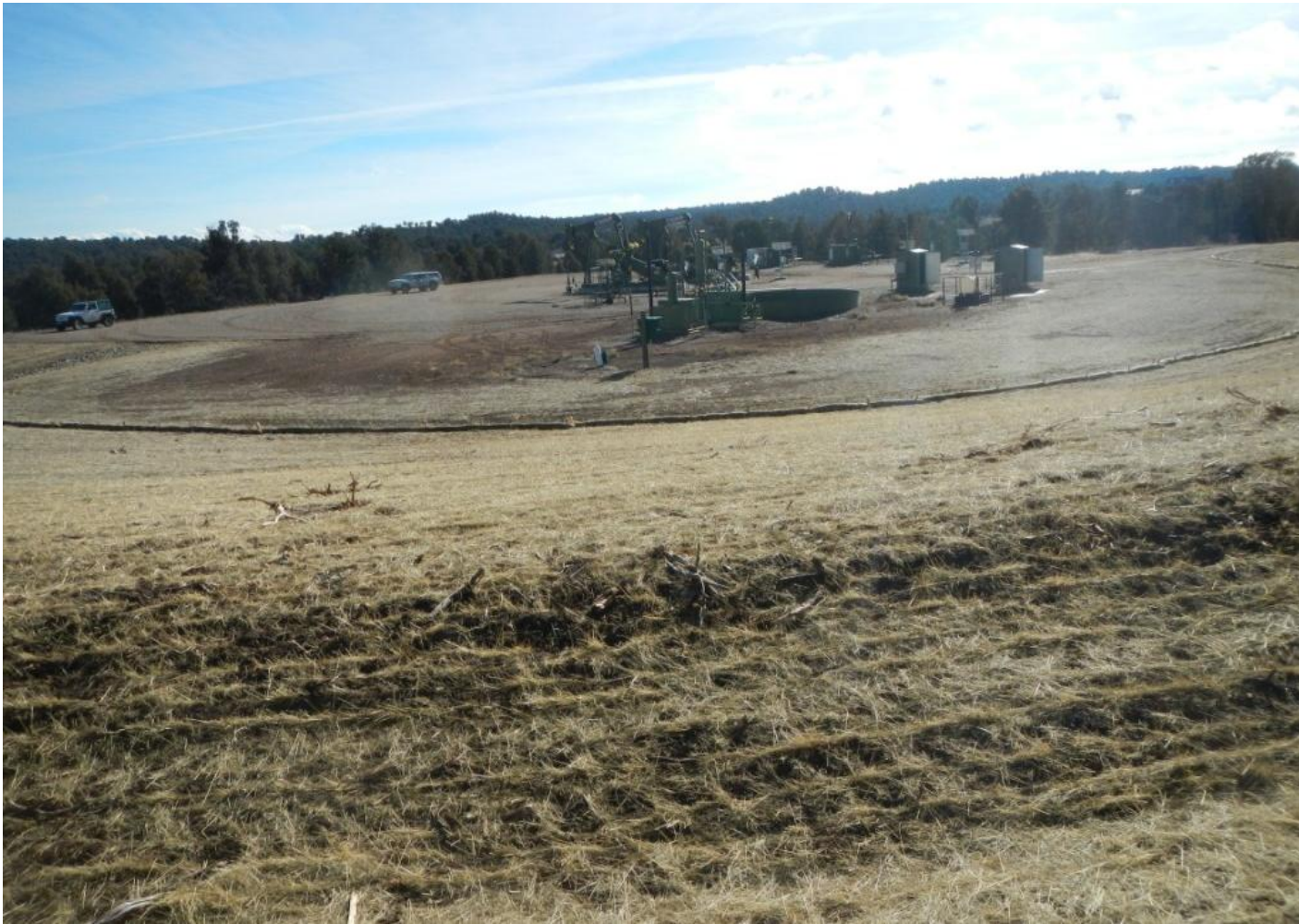
Photo 1. View of the project area from the northwestern corner facing center. Slopes and well pad are straw mulched, recontoured, and stormwater controls installed.
