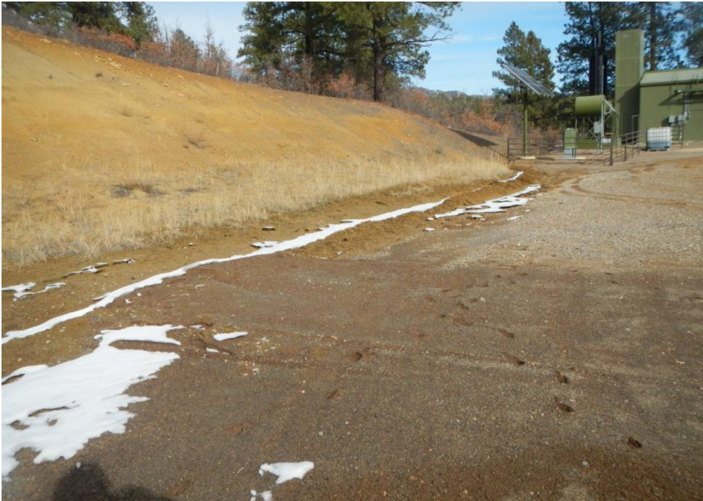
Photo 4. View of the northern portion of the project area from the northwestern edge facing eastward. Vegetation on northern cut-slope is sparse and may need to be revegetated if it is not increasing.
