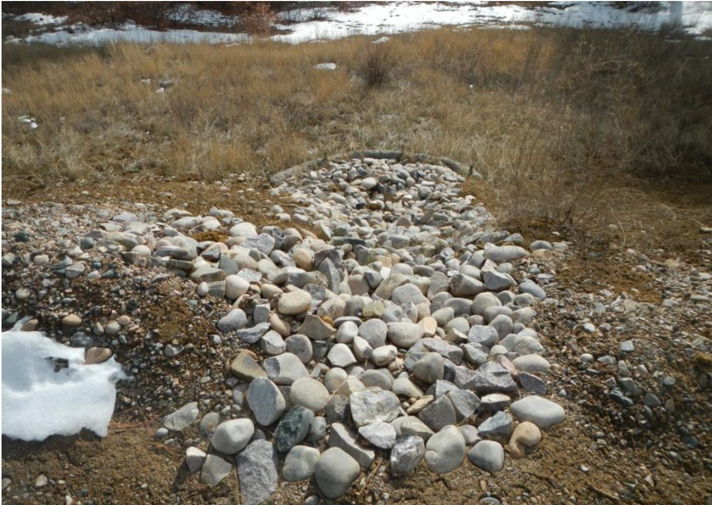
Photo 6. View of cobble run-down in the southwestern portion of the project area.
