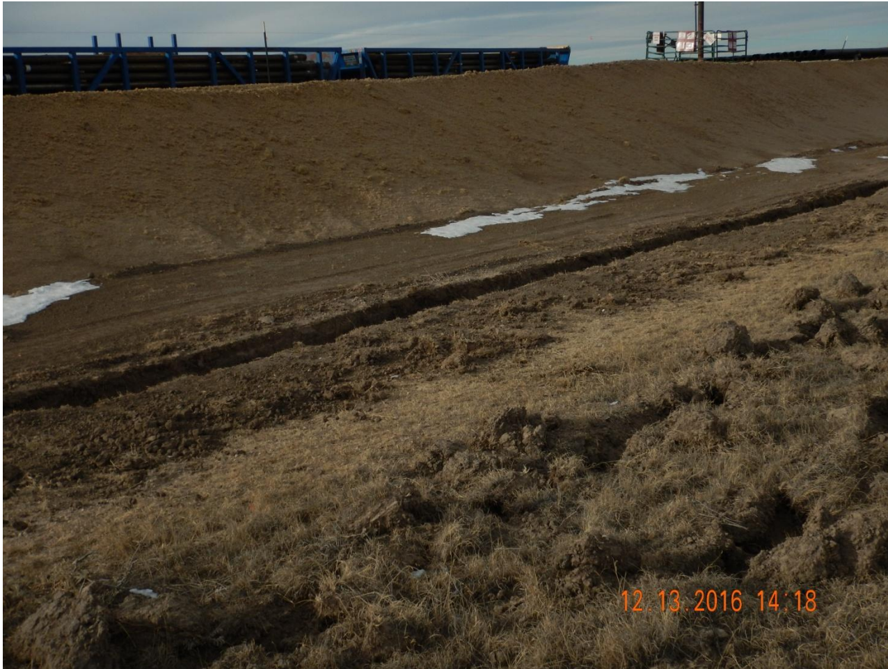
Photo 8. Photo taken from eastern location, facing West. Tackifier applied to fill slope.
