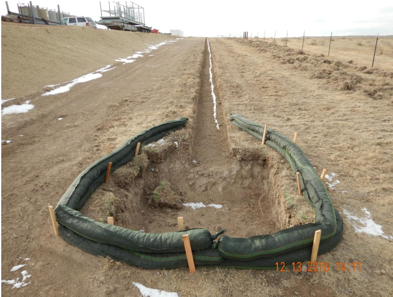
Photo 2. Photo taken from the northeast sediment trap, facing West. Sediment trap approximately 4'x4'x3' with rock socks. Trench approximately 18"x12" (width xdepth) installed along the northern perimeter of location.
