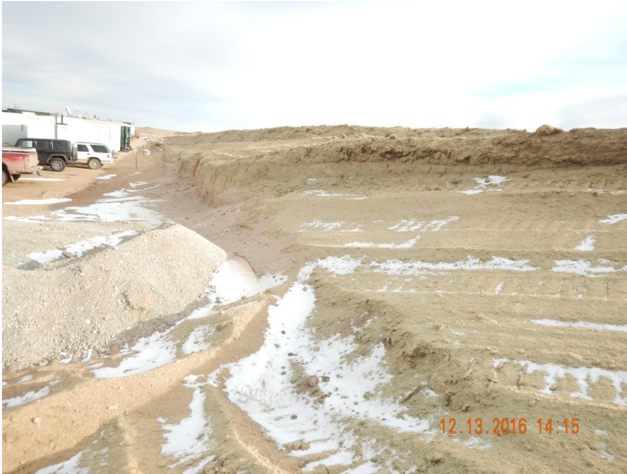
Photo 5. Photo taken from the southwest pad location, facing East. Tackifier has been applied to cut slope but may need additional stabilization with a 1:1 slope.
