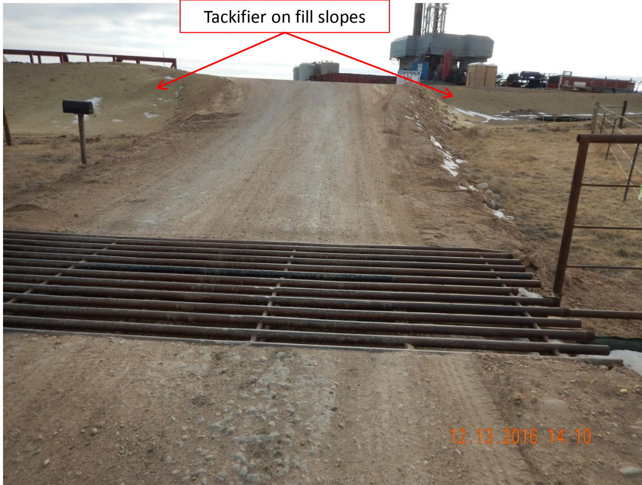
Photo 1. Photo taken from the entrance of the location, facing South. Tackifier has been applied to all fill and cut slopes on location.
