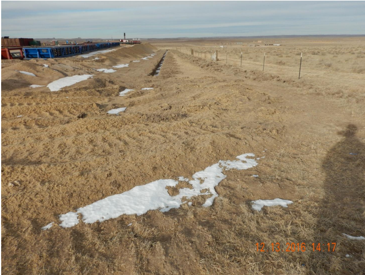
Photo 6. Photo taken from the southeast location, facing North. Surface roughening BMP installed along eastern location with 5'-6' vegetated area between trench and BMP. A sediment trap approximately 4'x4'x3' with filter socks is installed at the northeast corner of location.
