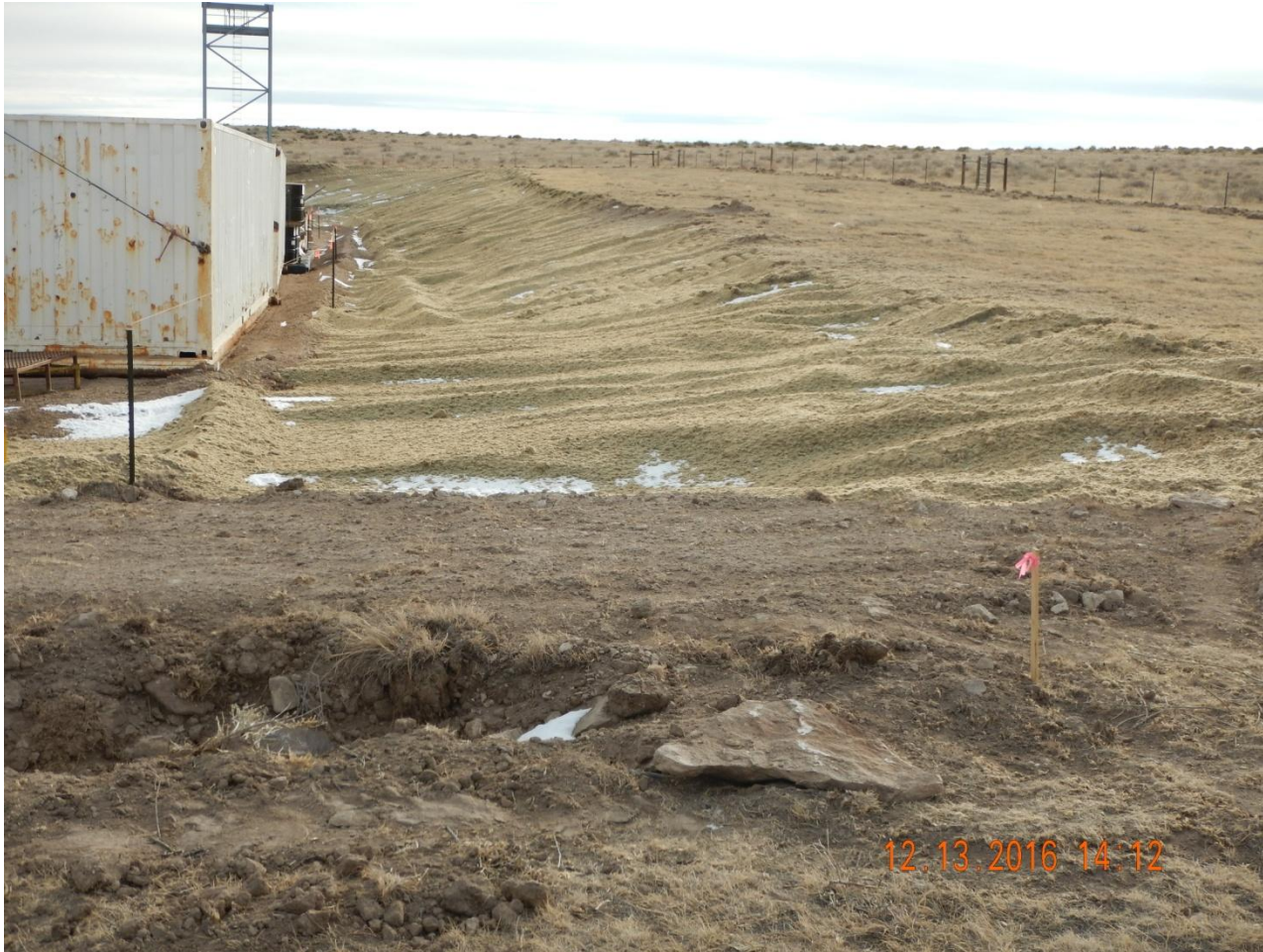
Photo 3. Photo taken from the northwest location, facing South. Cut slope has been stabilized with a tackifier.
