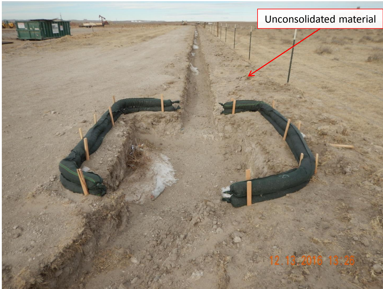
Photo 6. Photo taken from the southeast sediment trap, facing North. Sediment trap approximately 4'x4'x2.5' with filter socks. Trench approximately 18"x12" (width x depth) installed along the eastern perimeter of location. Unconsolidated soil dug out from the trench has not been stabilized.
