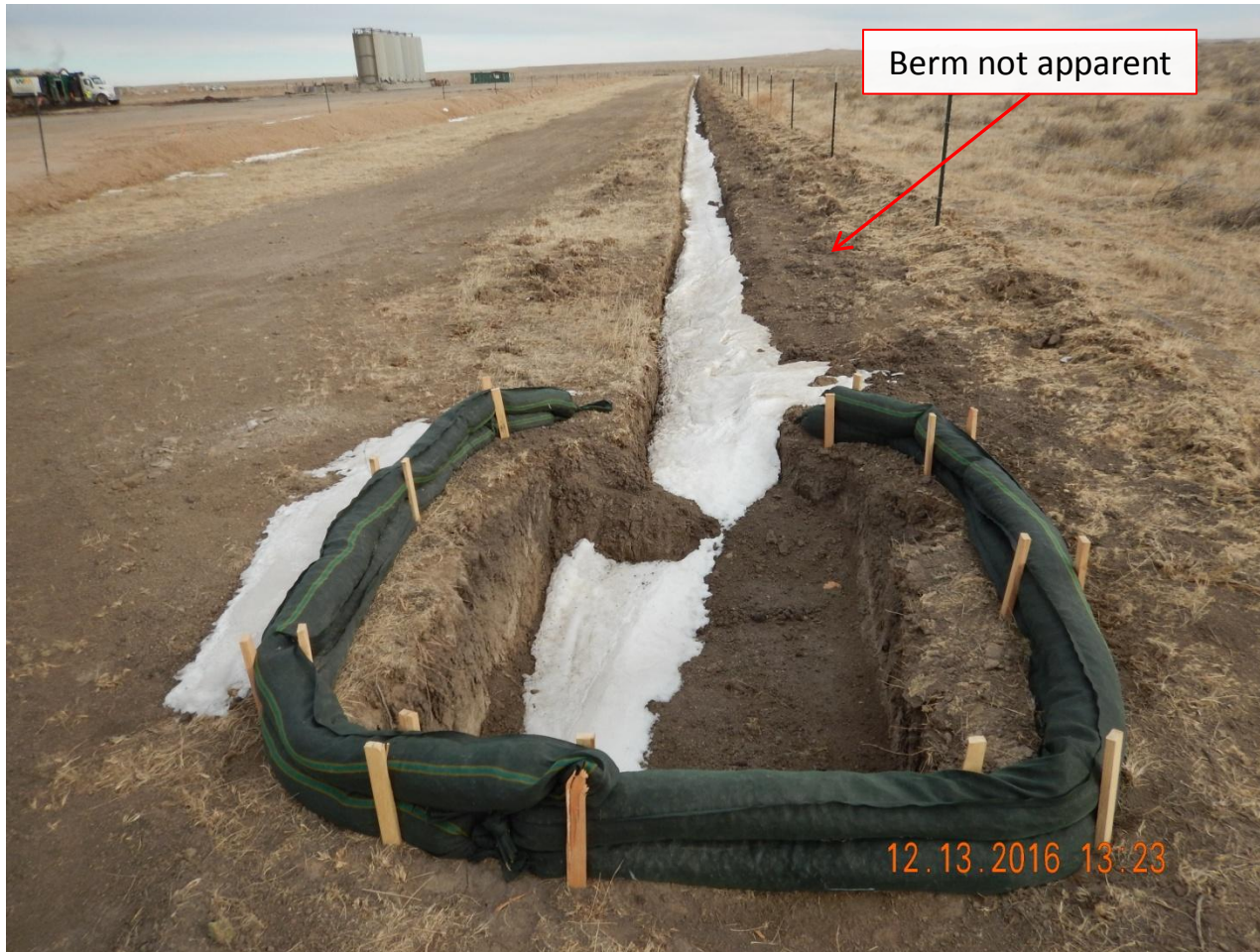
Photo 4. Photo taken from the previous sediment trap, facing East. Trench approximately 18"x12" (width x depth) installed along the southern perimeter of location. No apparent berm associated with trench.
