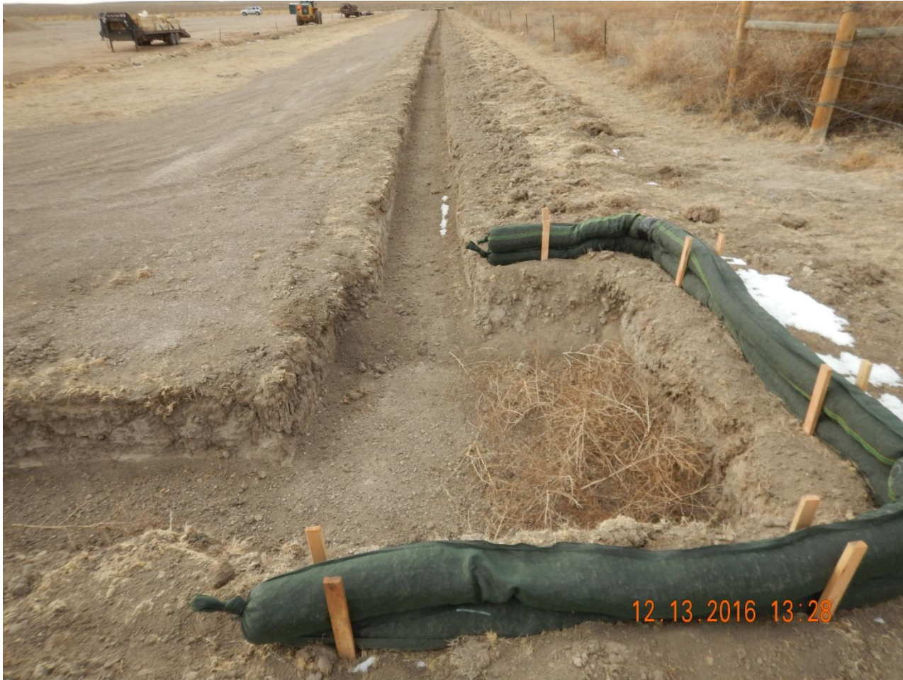
Photo 8. Photo taken from the northeast sediment trap, facing West. Sediment trap approximately 4'x3'x2' with rock socks. Trench approximately 18"x12" (width x depth) installed along the northern perimeter of location. A light application of tackifier has been applied to soil dug out from the trench. May need additional tackifier to stabilize soil.
