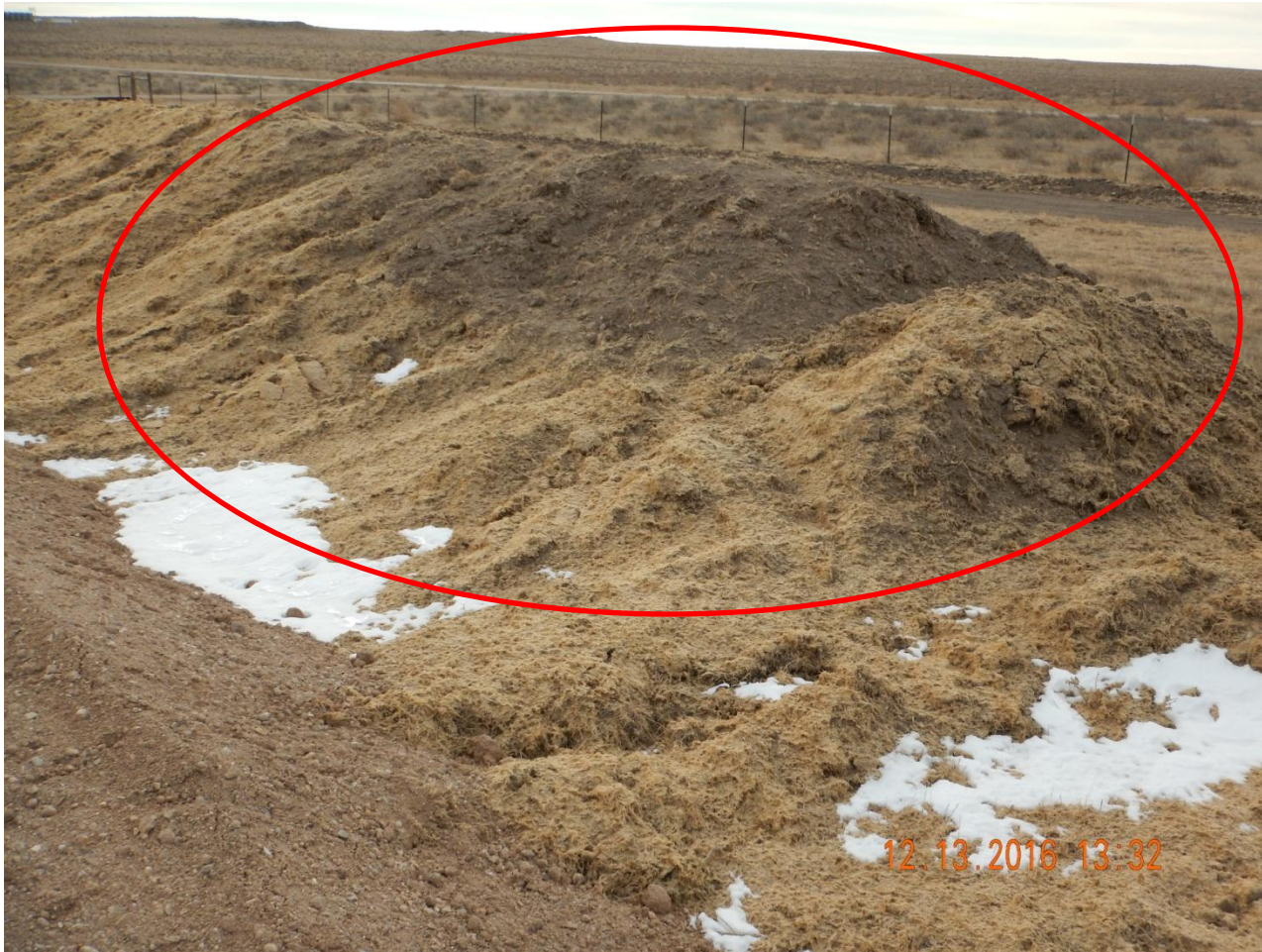
Photo 11. Photo taken from the western location, facing West, along the topsoil stockpile. May need to stabilize topsoil stockpile with additional tackifier in areas.
