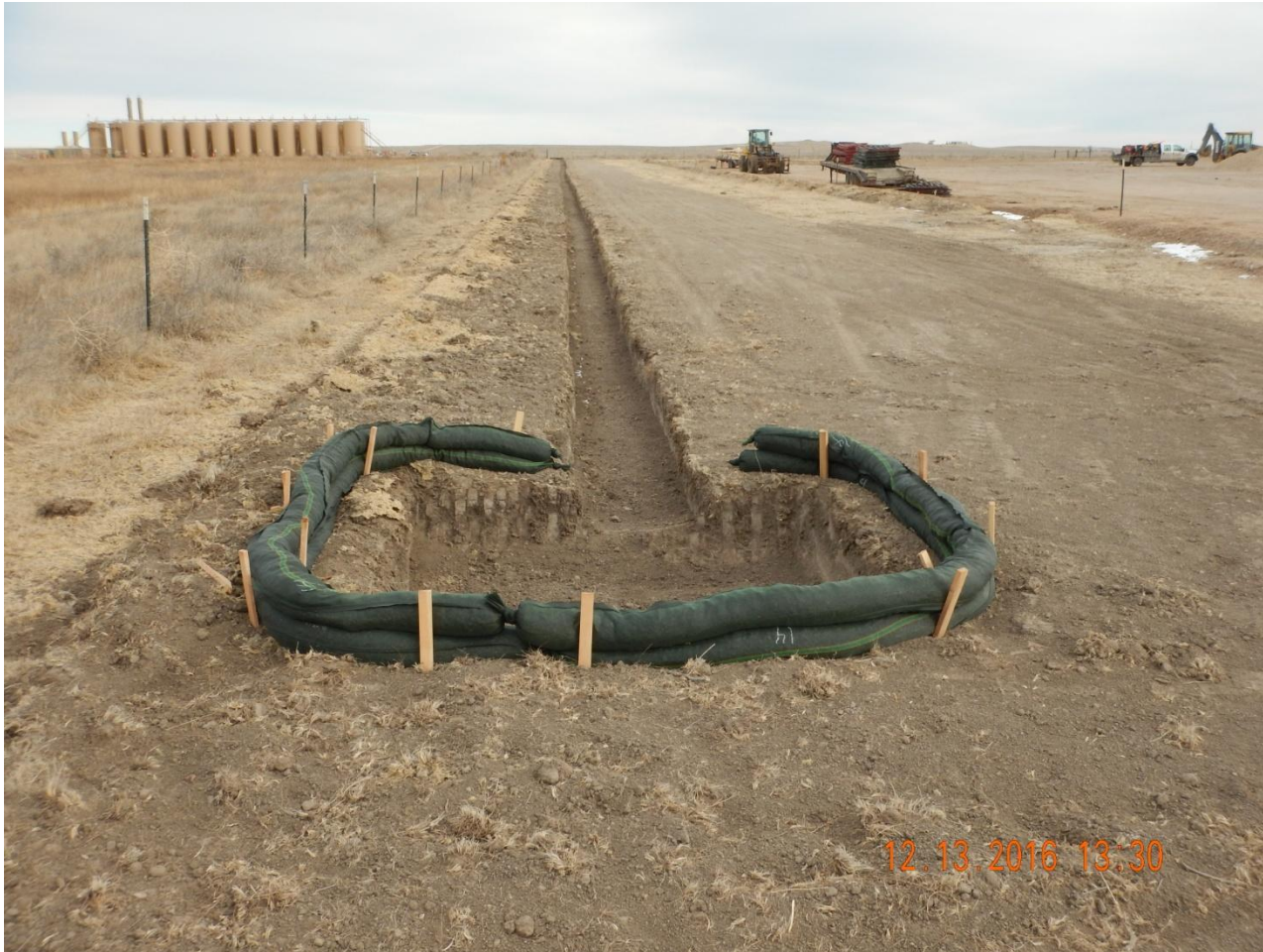
Photo 9. Photo taken from the northwest sediment trap, facing East. Sediment trap approximately 4'x3'x2' with rock socks.
