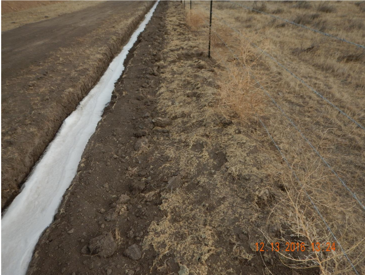
Photo 5. Photo taken from the southern location, facing East. Unconsolidated soil dug out from the trench sprayed with tackifier but may need additional tackifier because the application rate appears too low.
