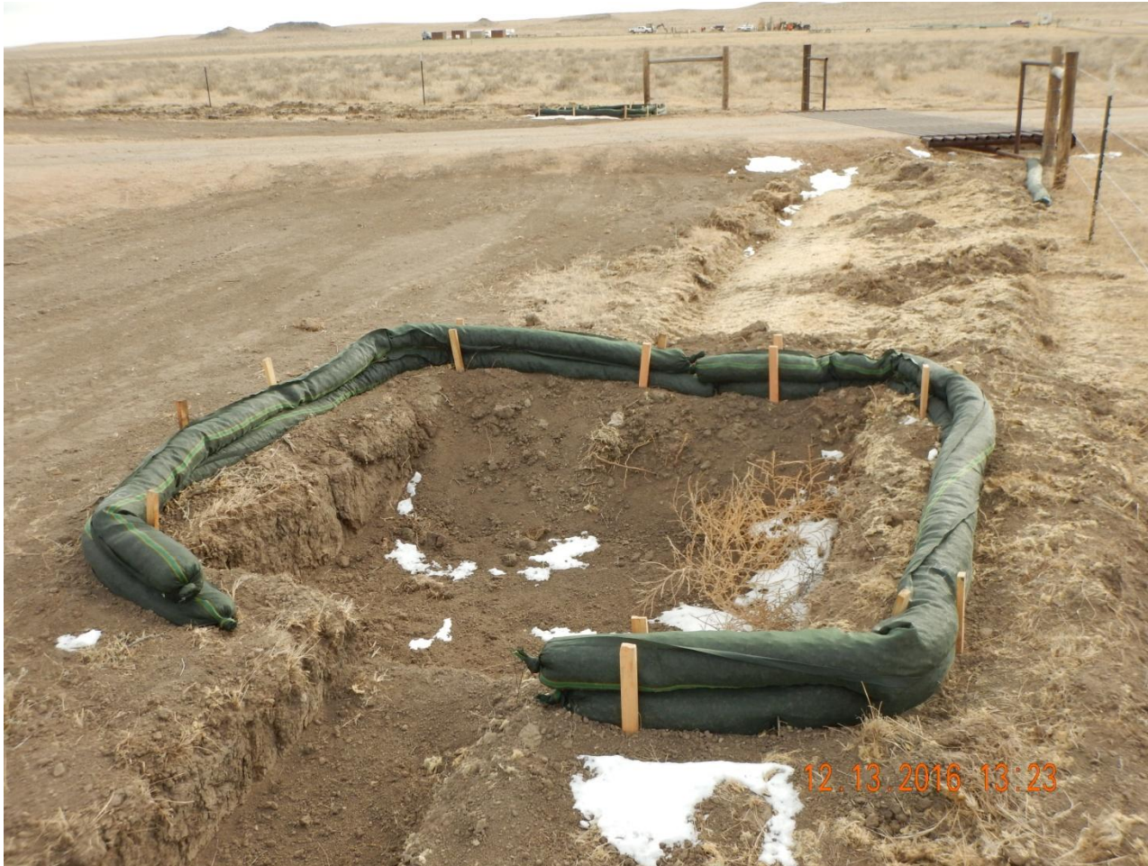
Photo 2. Photo taken from the southwest sediment trap north of the access road, facing South. Sediment trap approximately 4'x4'x2.5' with rock socks.
