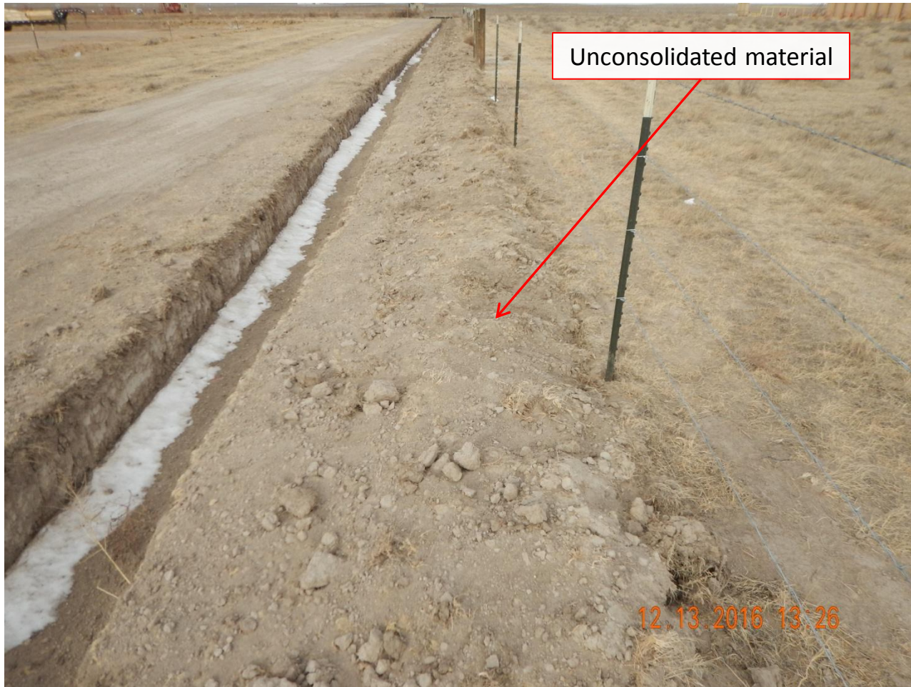
Photo 7. Photo taken from eastern location, facing North. Unconsolidated soil dug out from the trench has not been stabilized.
