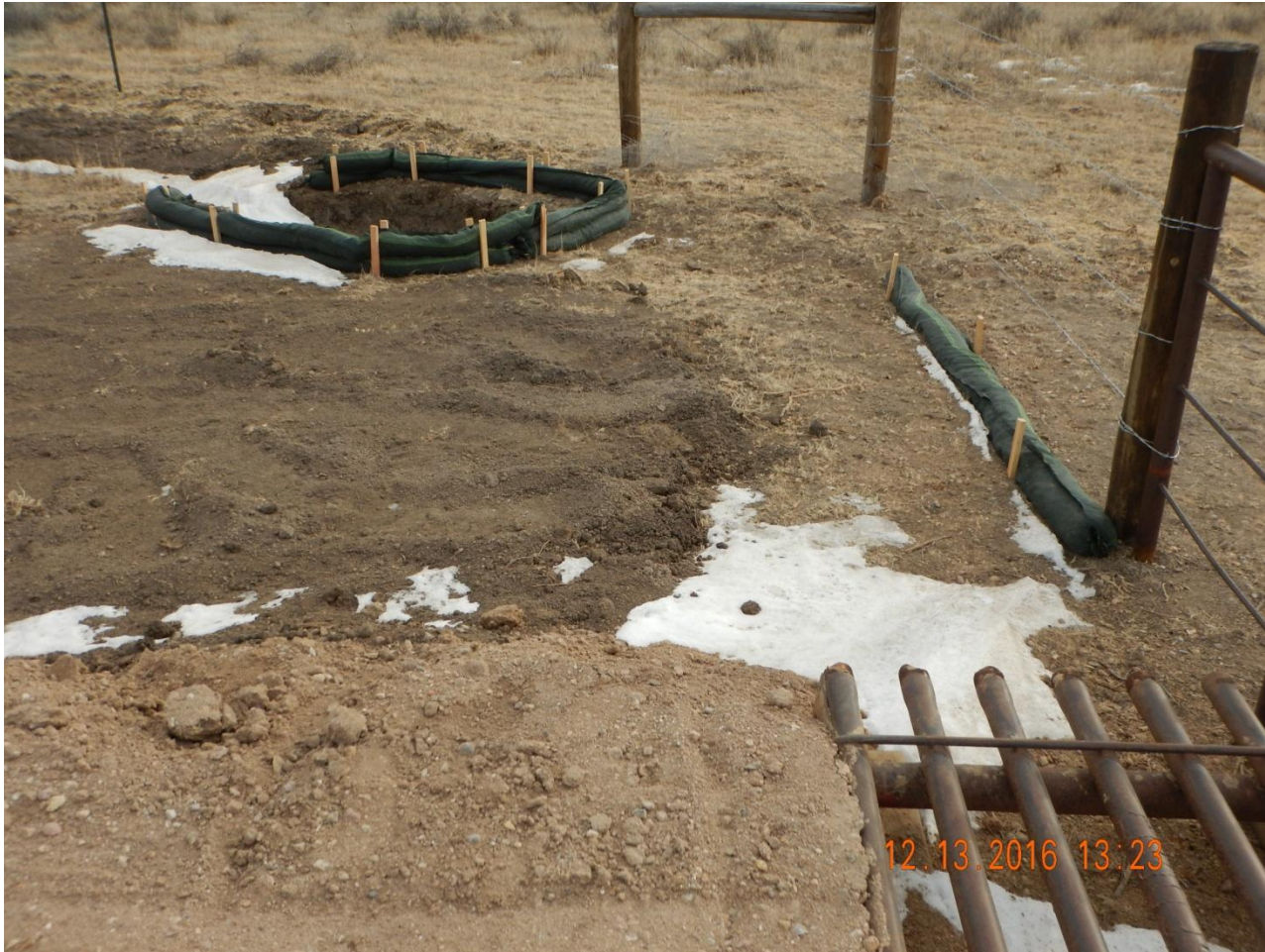
Photo 3. Photo taken from the southwest sediment trap south of the access road, facing South. Sediment trap approximately 4'x4'x2.5' with rock socks.
