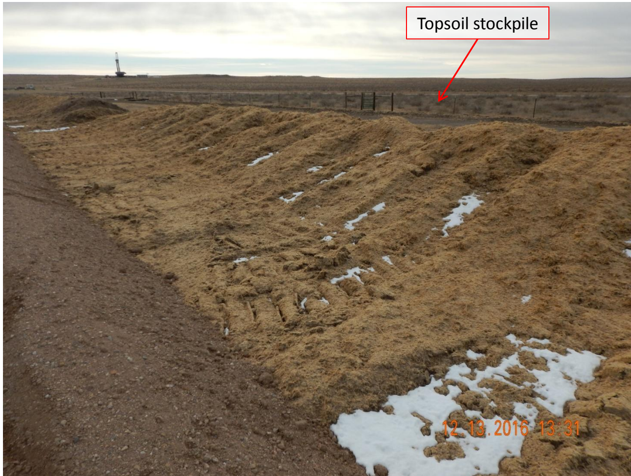
Photo 10. Photo taken from the western location, facing Southwest, along the topsoil stockpile. Tackifier applied to the topsoil stockpile. Not certain whether topsoil was seeded in addition to applying tackifier, but tackifier alone is not a long-term stabilization BMP to protect topsoil from erosion and weed establishment.
