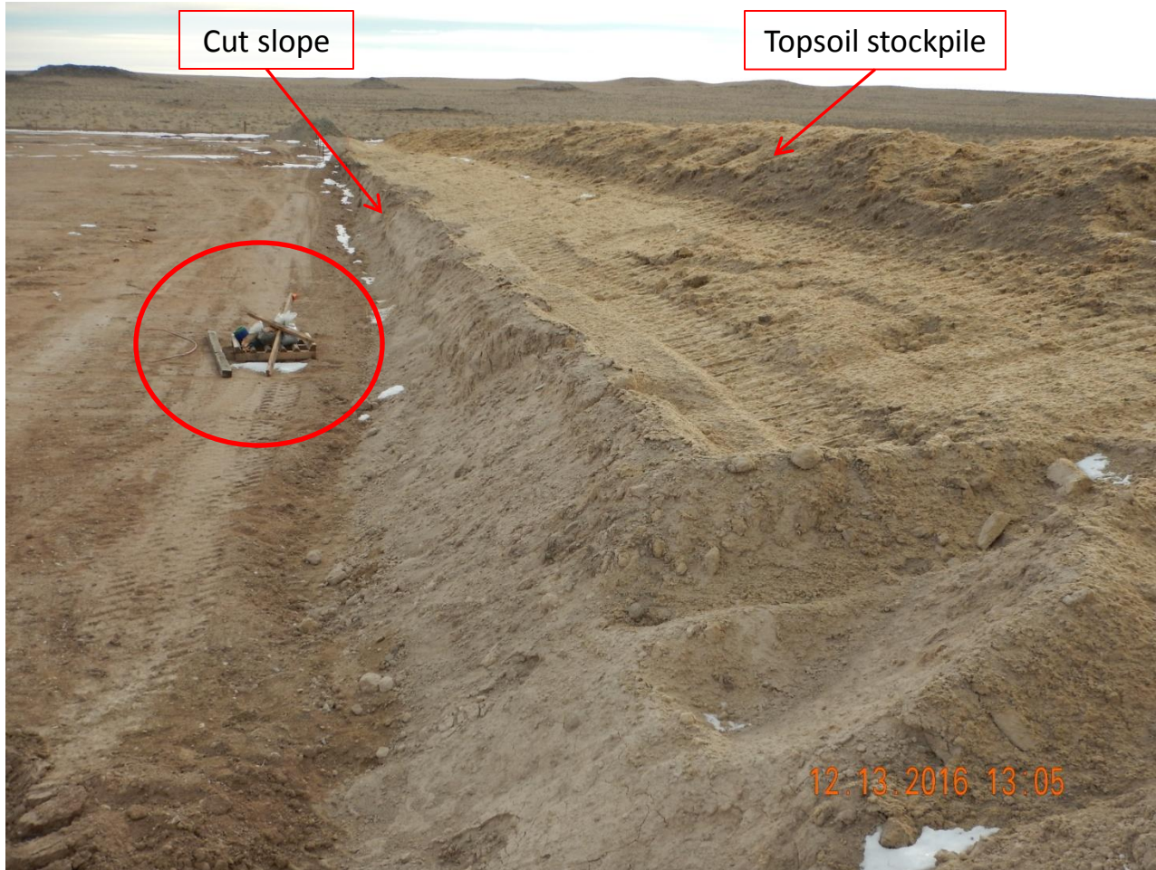
Photo 8. Photo taken from western pad cut slope, facing South. Cut slope does not appear to be stabilized (1:1 slope) and a 2:1 slope would be appropriate with additional stabilization measures. Remove waste material per Rule 603.f.
