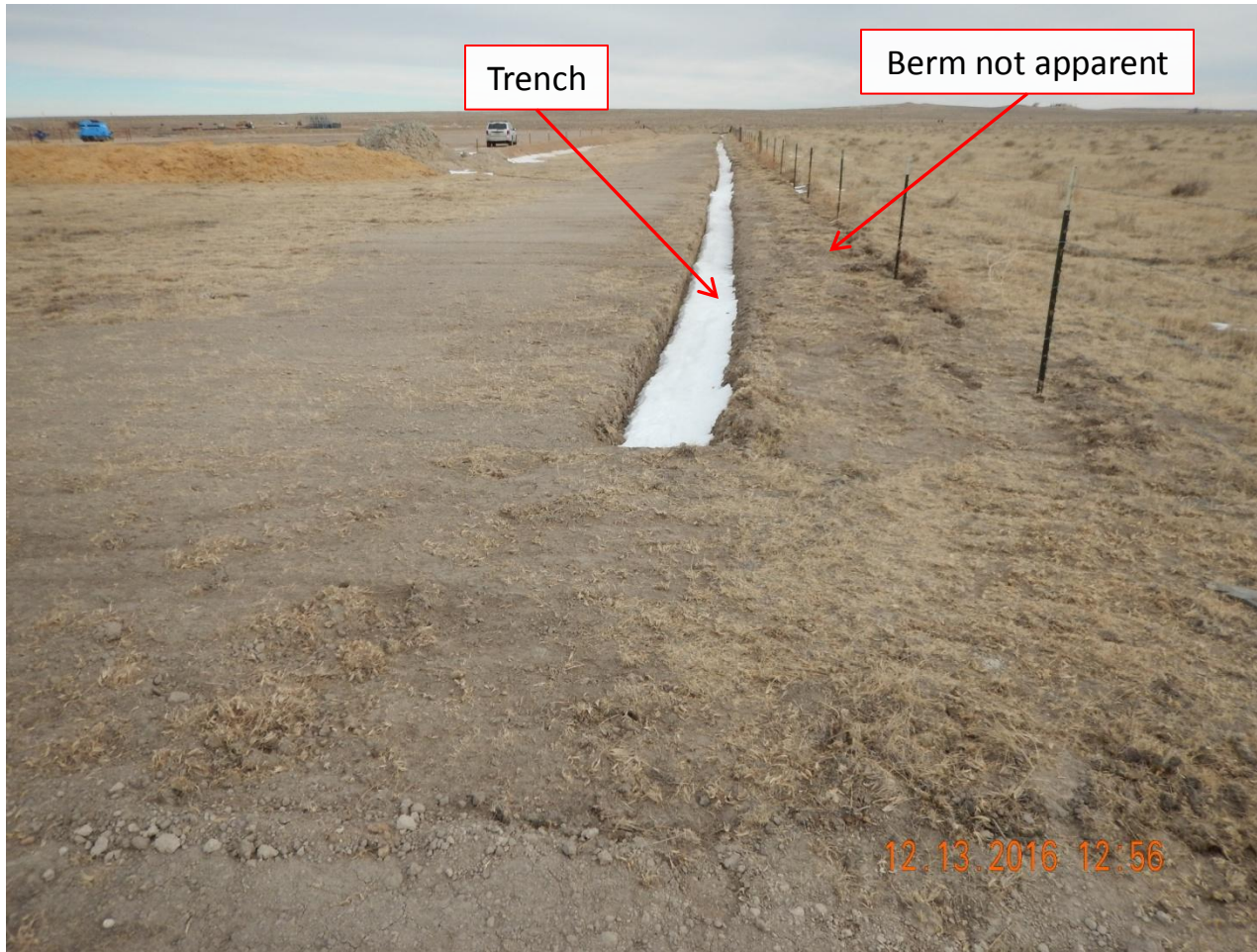
Photo 1. Photo taken from southwest location, facing East. Trench approximately 18"x12" (width x depth) installed along the southern perimeter of location. No apparent berm associated with trench.
