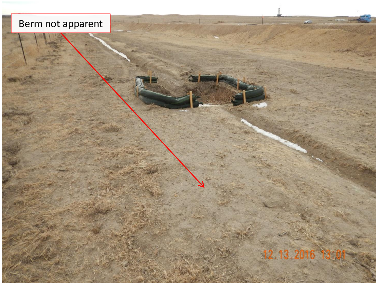
Photo 5. Photo taken from the northeast location, facing South. Sediment trap approximately 4'x4'x2.5' with filter socks.
