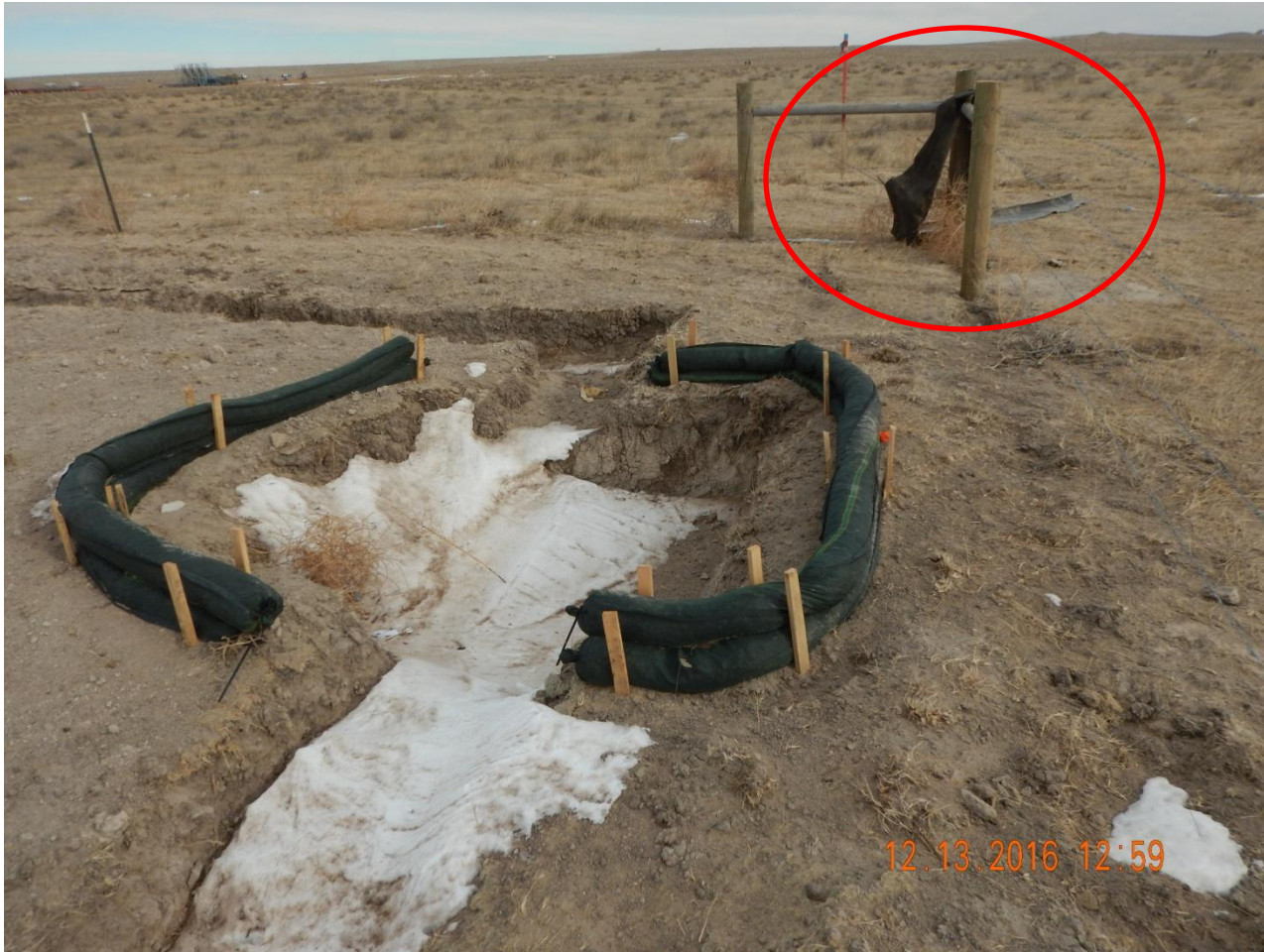
Photo 2. Photo taken from the southeast sediment trap, facing East. Sediment trap approximately 4'x4'x2.5' with rock socks. Need to remove waste material from fence per Rule 603.f.
