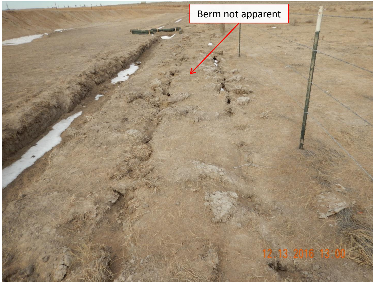
Photo 4. Photo taken from southeast location, facing North. Trench approximately 18"x12" (width x depth) installed along the eastern perimeter of location. No apparent berm associated with trench.
