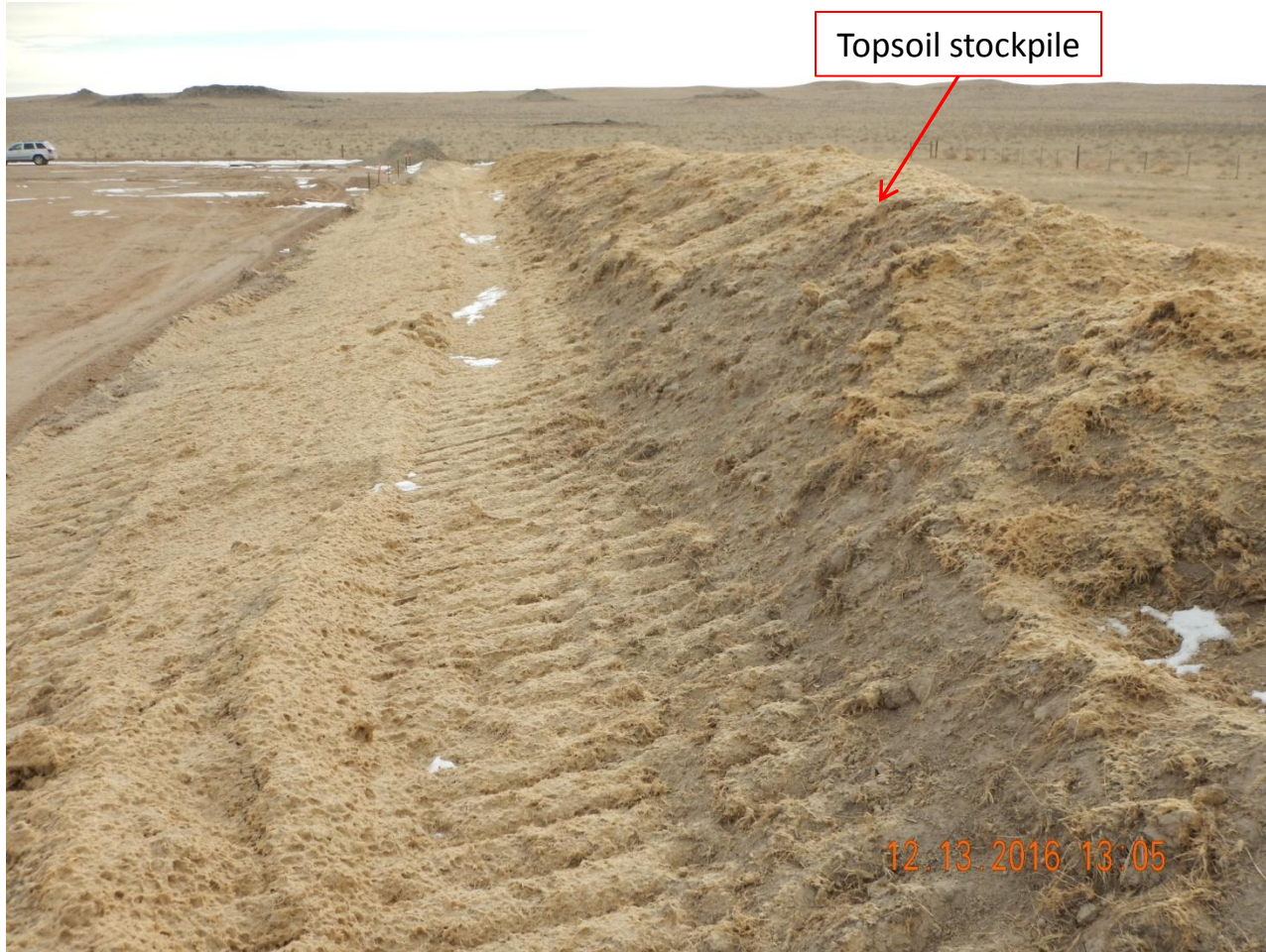
Photo 9. Photo taken from the western location, facing South, along the topsoil stockpile. Tackifier applied to the topsoil stockpile and the east-facing edge. Not certain whether topsoil was seeded in addition to applying tackifier, but tackifier alone is not a long-term stabilization BMP to protect topsoil from erosion and weed establishment.
