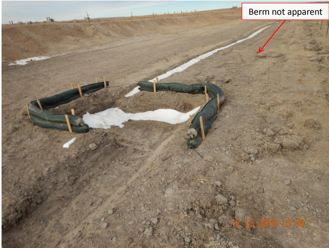
Photo 4. Photo taken from the east central sediment trap, facing North. Sediment trap approximately 4'x4'x2' with rock socks.
