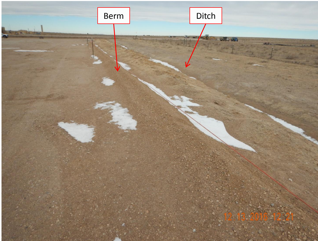
Photo 1. Photo taken from eastern location, facing North. A berm approximately 10"-12" constructed of road base installed along the east, south, and west pad perimeter. An outer perimeter ditch installed along the east, south and west pad perimeter.
