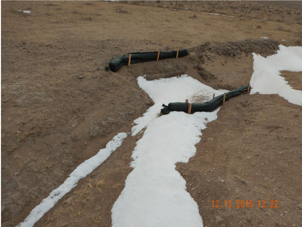
Photo 4. Photo taken from the southeast sediment trap. Sediment trap approximately 4'x4'x2.5' with filter socks. Sediment trap is about 1/3 filled in with sediment.
