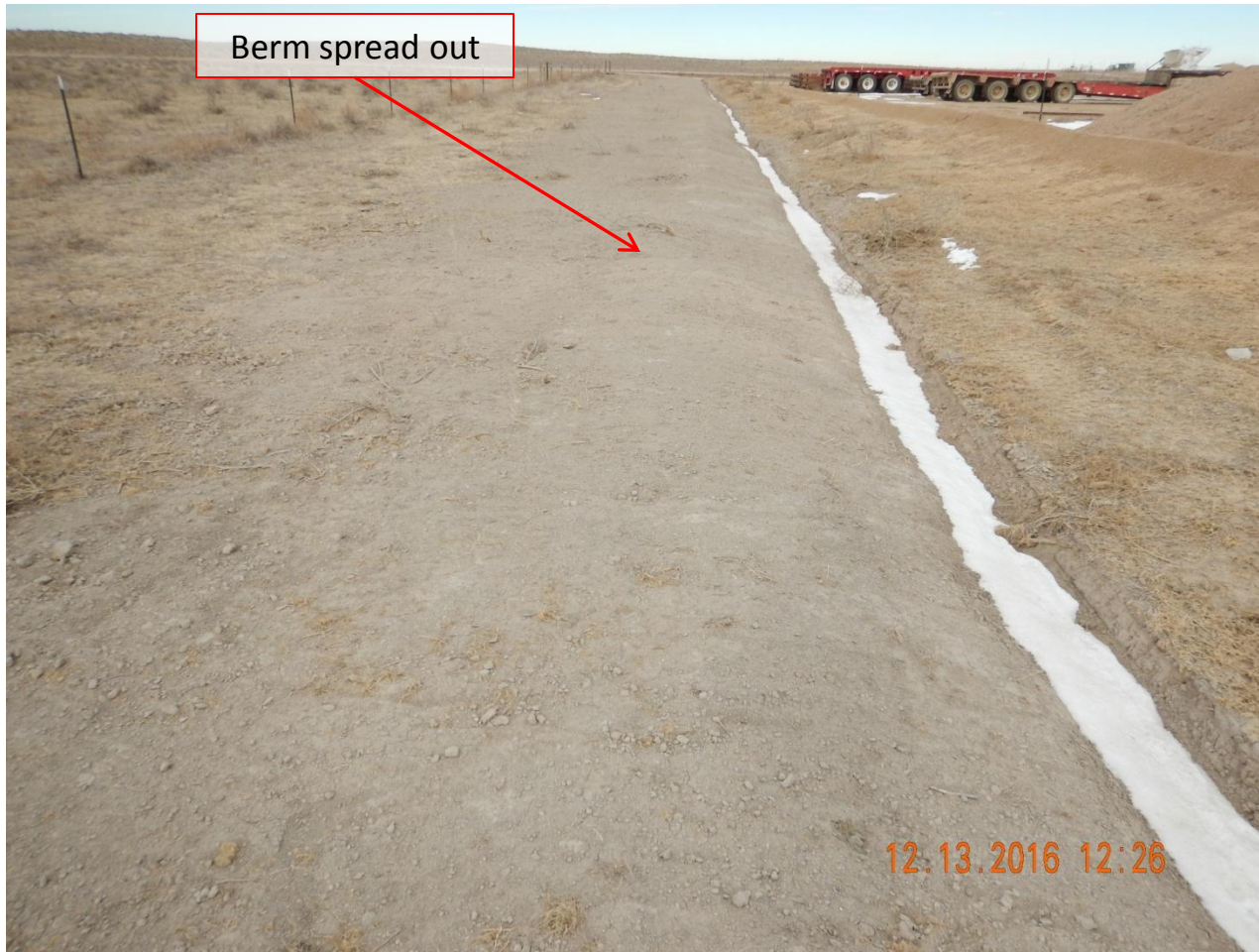
Photo 9. Photo taken from western location, facing North. Ditch approximately 8-12" in depth installed along the western perimeter. Berm appears to be spread out and not apparent along the western perimeter.
