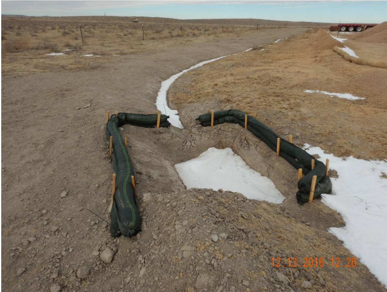
Photo 7. Photo taken from southwest location, facing North. Sediment trap approximately 3'x3'x2' with rock socks.
