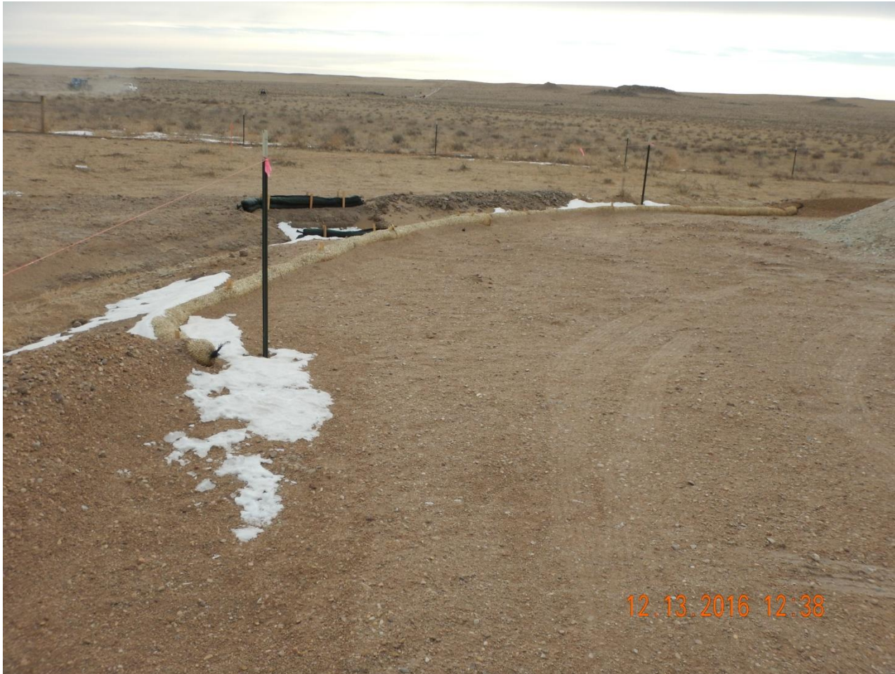
Photo 3. Photo taken from the southeast location, facing South. Wattles have been installed along the southeast pad corner with a sediment trap to the outer perimeter. Appears wattles may be used to filter storm runoff before entering the sediment trap which is not the proper use. See inspection for more details.
