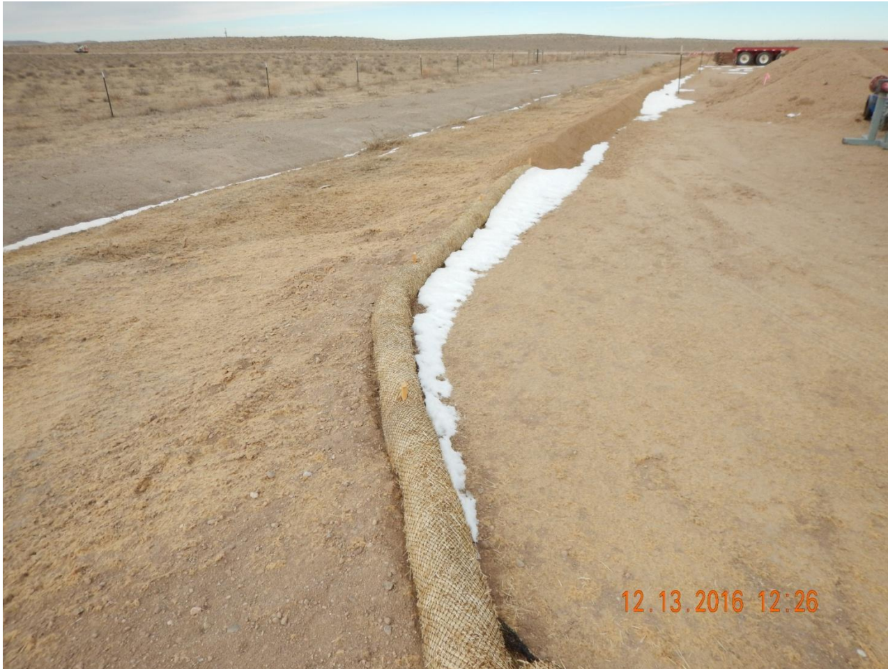
Photo 8. Photo taken from the southwest location, facing North. Wattles have been installed along the southwest pad corner in conjunction with a 12" berm along the pad perimeter. Appears wattles may be used to filter storm runoff before entering the sediment trap which is not the proper use. See inspection for more details.
