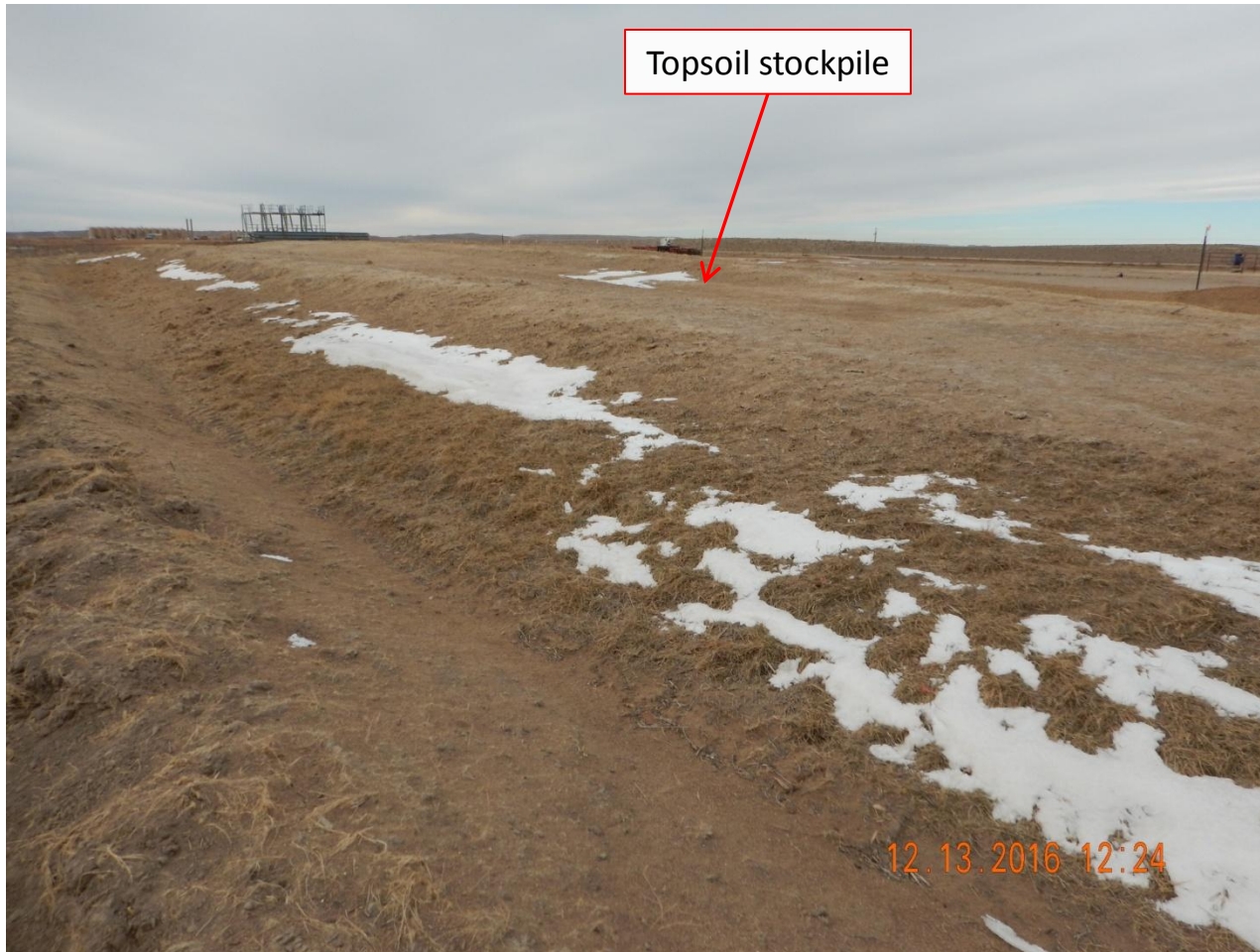
Photo 6. Photo taken from the southern location, facing North, towards the topsoil stockpile. Tackifier applied to the topsoil stockpile. May need additional stabilization on the top of the stockpile where it is susceptible to wind erosion.
