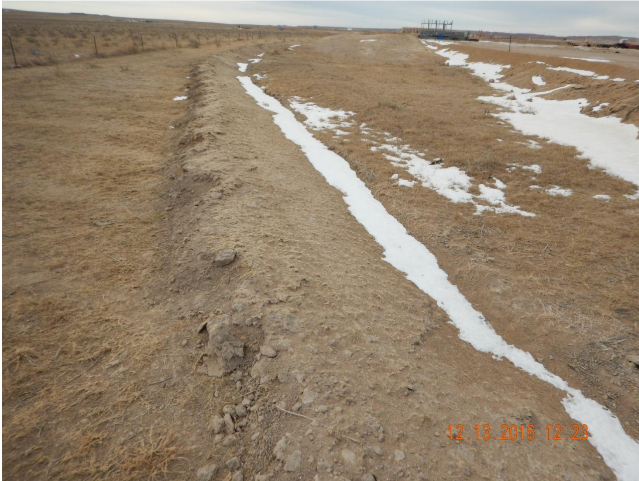
Photo 5. Photo taken from the southeast location, facing West. Ditch and berm installed along the southern location. Unconsolidated berm has been sprayed with a tackifier. May need additional stabilization along portions of the berm.
