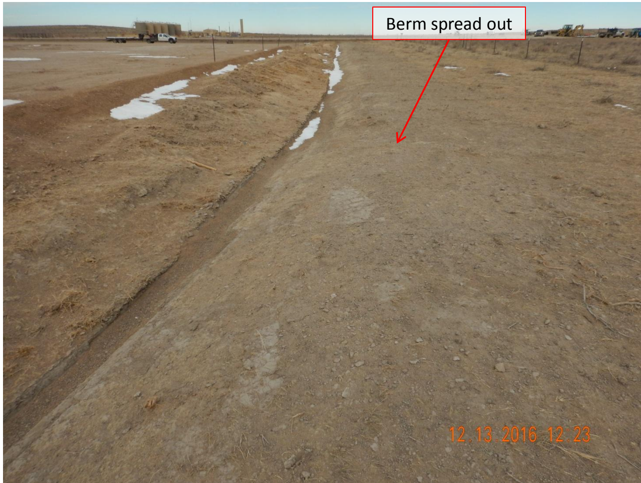
Photo 2. Photo taken from eastern location, facing North. Ditch approximately 8-12" in depth installed along the eastern perimeter is filling in with sediment. Berm appears to be spread out and not apparent along the western perimeter.
