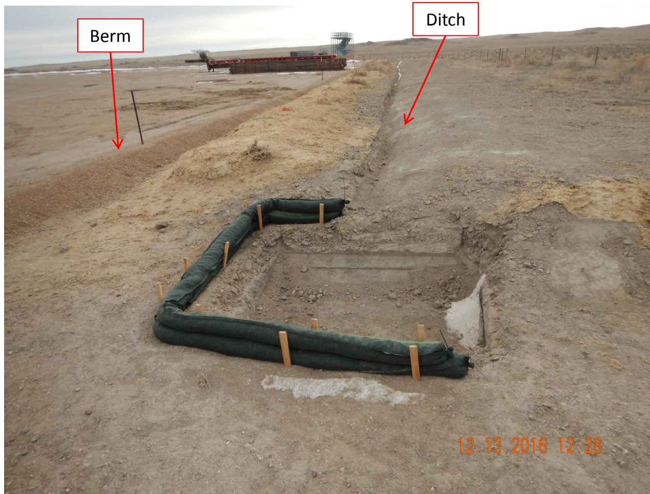
Photo 10. Photo taken from northwest location, facing South. Sediment trap approximately 4'x4'x2' with filter socks. A berm approximately 10"-12" constructed of road base installed along the west pad perimeter.
