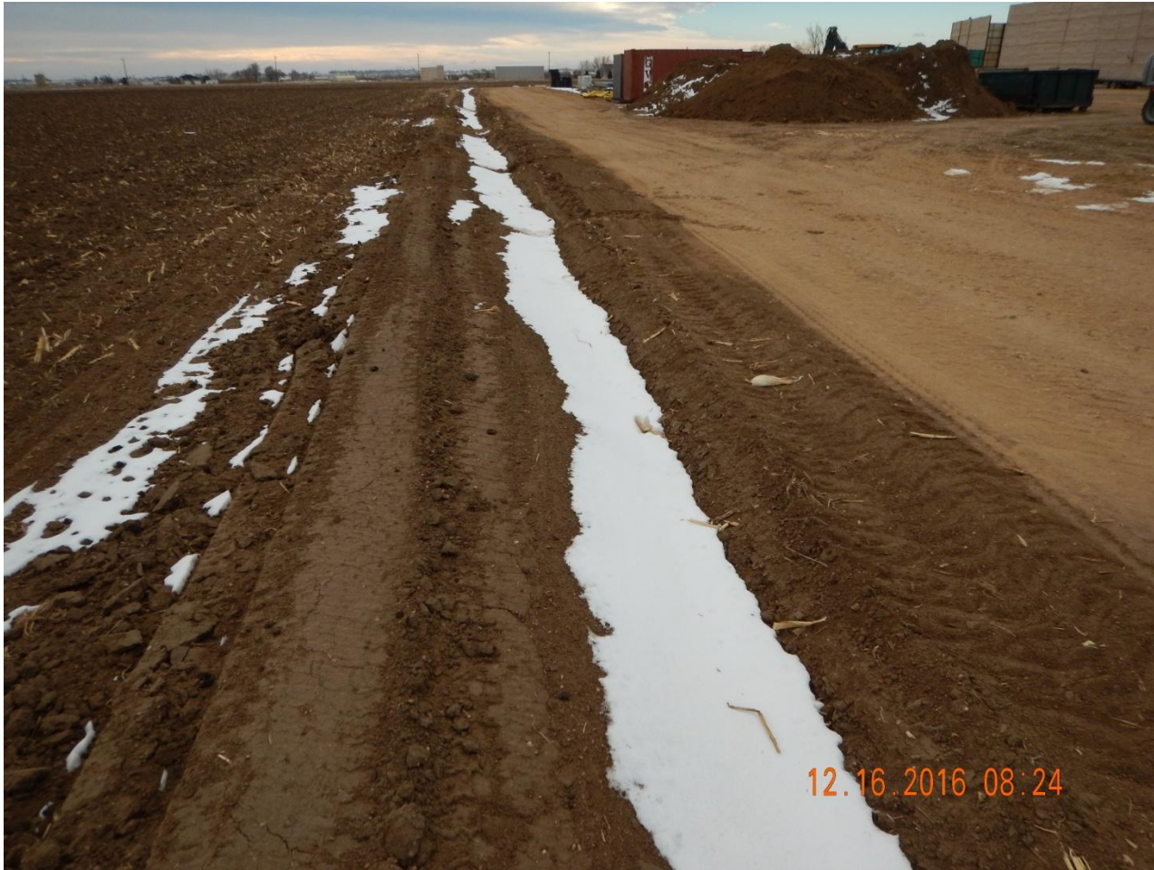
Photo 6. Photo taken from the eastern location, facing South. Ditch and berm BMP installed around the perimeter of the location.
