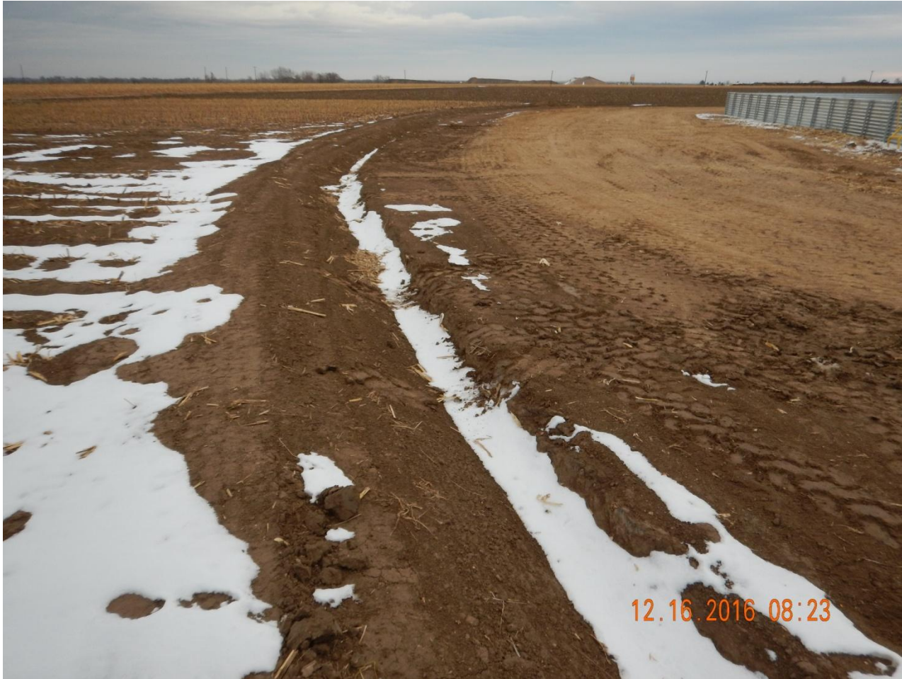
Photo 5. Photo taken from the northeastern location, facing East. Ditch and berm BMP installed around the perimeter of the location.
