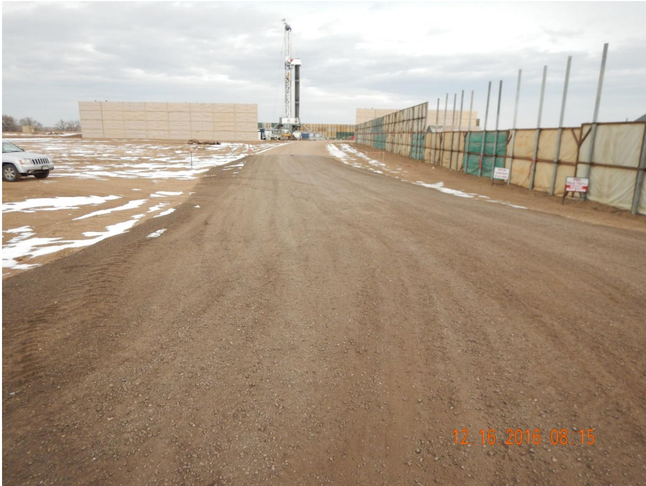
Photo 1. Photo taken from the entrance of location, facing South. Vehicle tracking pad installed at entrance to mitigate sediment discharge offsite.
