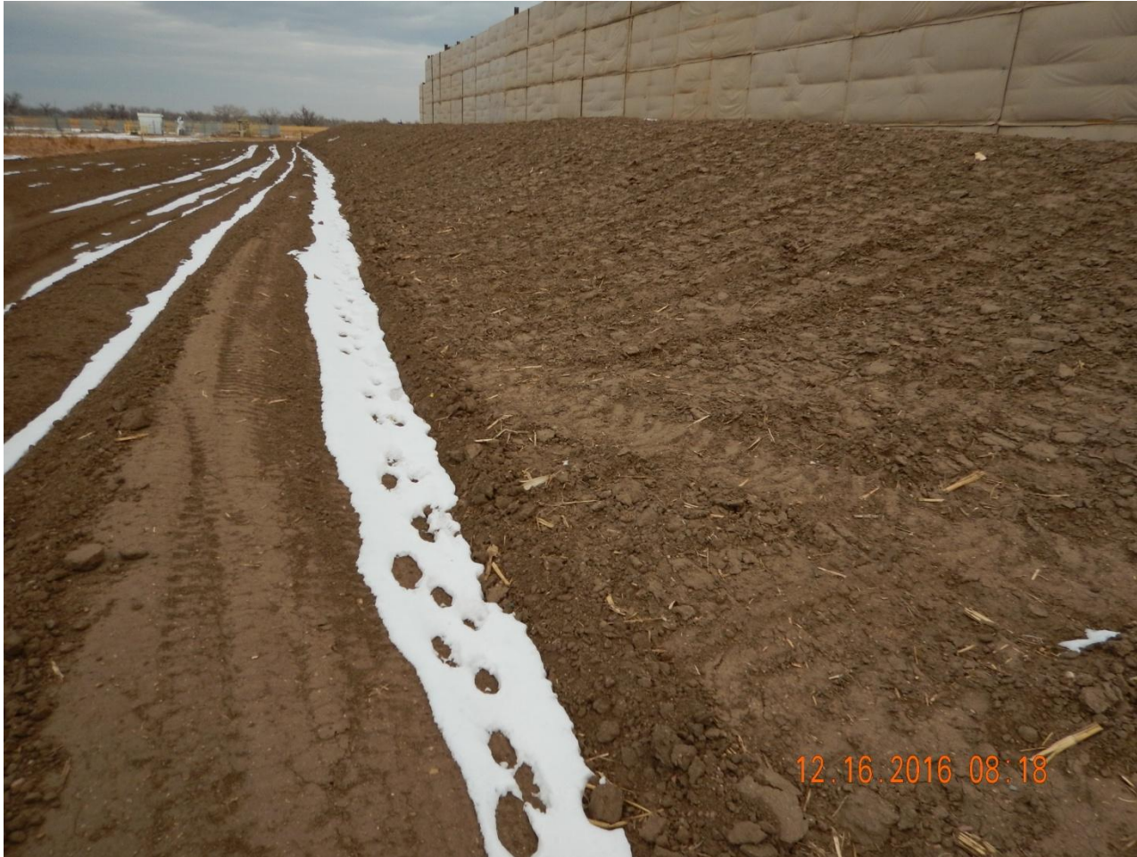
Photo 3. Photo taken from the western location, facing North, along the topsoil stockpile. Ditch and berm BMP installed around the perimeter of the location.
