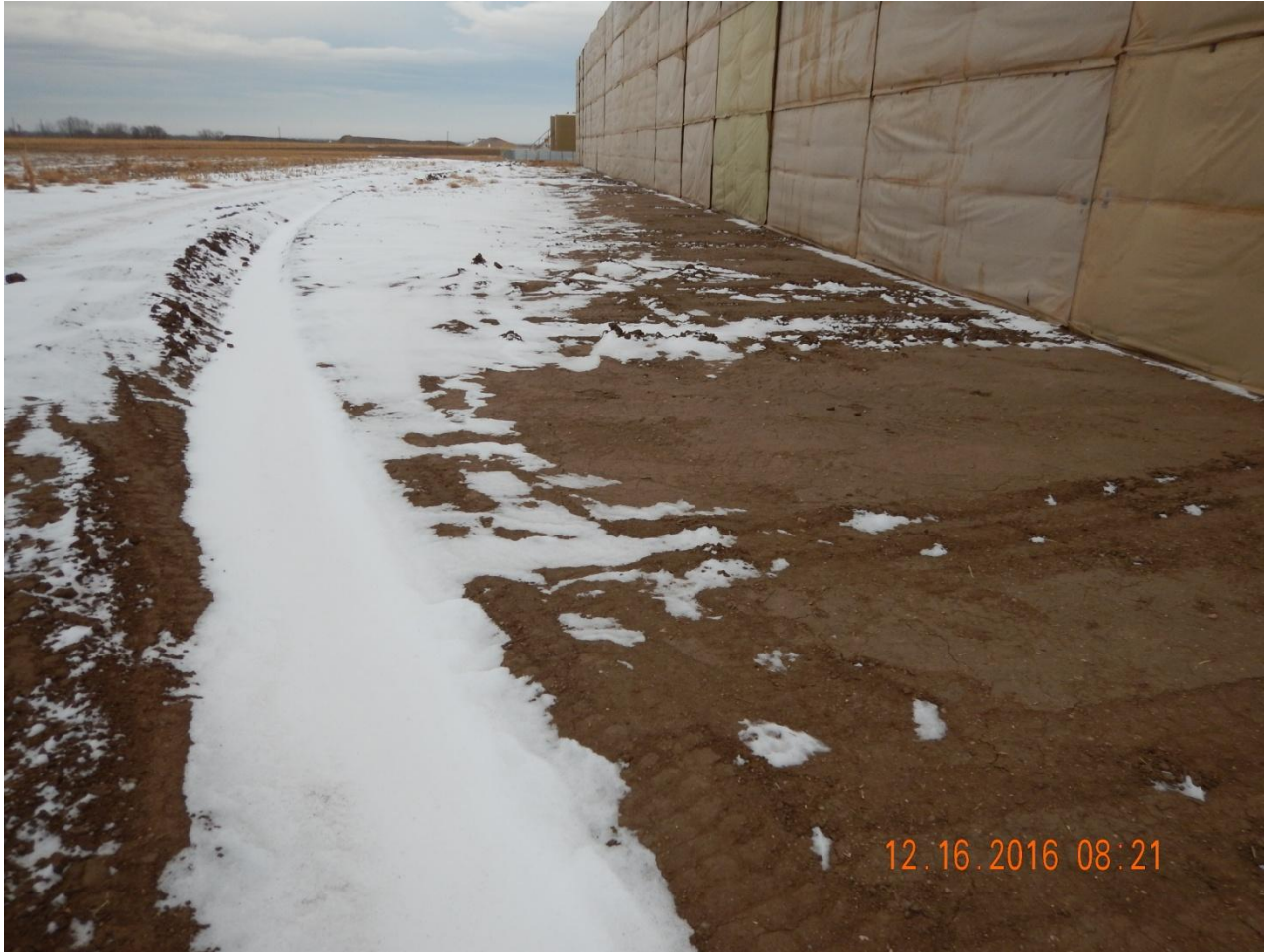
Photo 4. Photo taken from the northern location, facing East. Ditch and berm BMP installed around the perimeter of the location.
