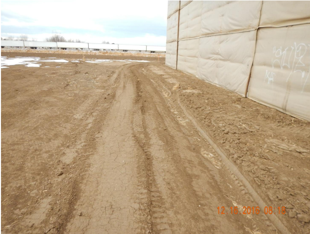
Photo 2. Photo taken from the southern location, facing West. Ditch and berm BMP installed around the perimeter of the location.
