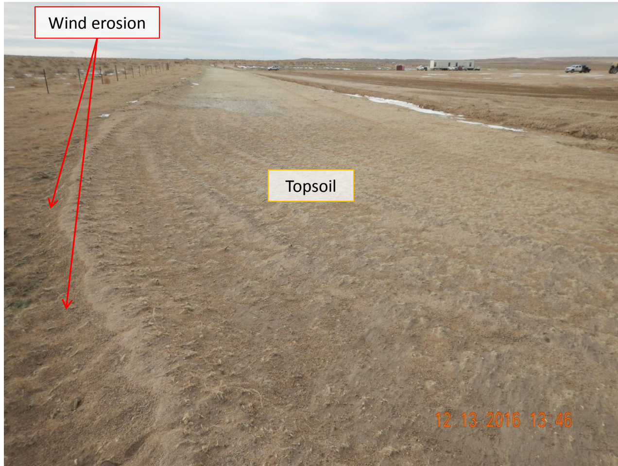
Photo 3. Photo taken from the southeast corner of location, facing West. Based on documentation, topsoil has been stored along the entire perimeter of the location. Tackifier has started to lose its stabilization capability. Need additional tackifier along this area. Also, need to install sufficient stormwater BMPs for the location.
