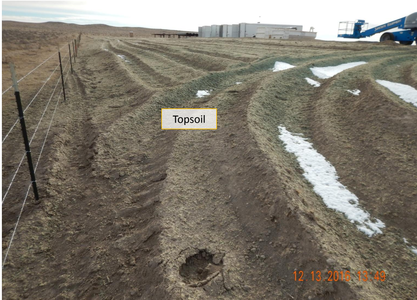
Photo 5. Photo taken from the northeast corner of location, facing South. Based on documentation, topsoil has been stored along the entire perimeter of the location. Tackifier has been applied to the topsoil but areas need additional tackifier because the application rate was too low- see Photos 3 & 4. Also, need to install sufficient stormwater BMPs for the location.
