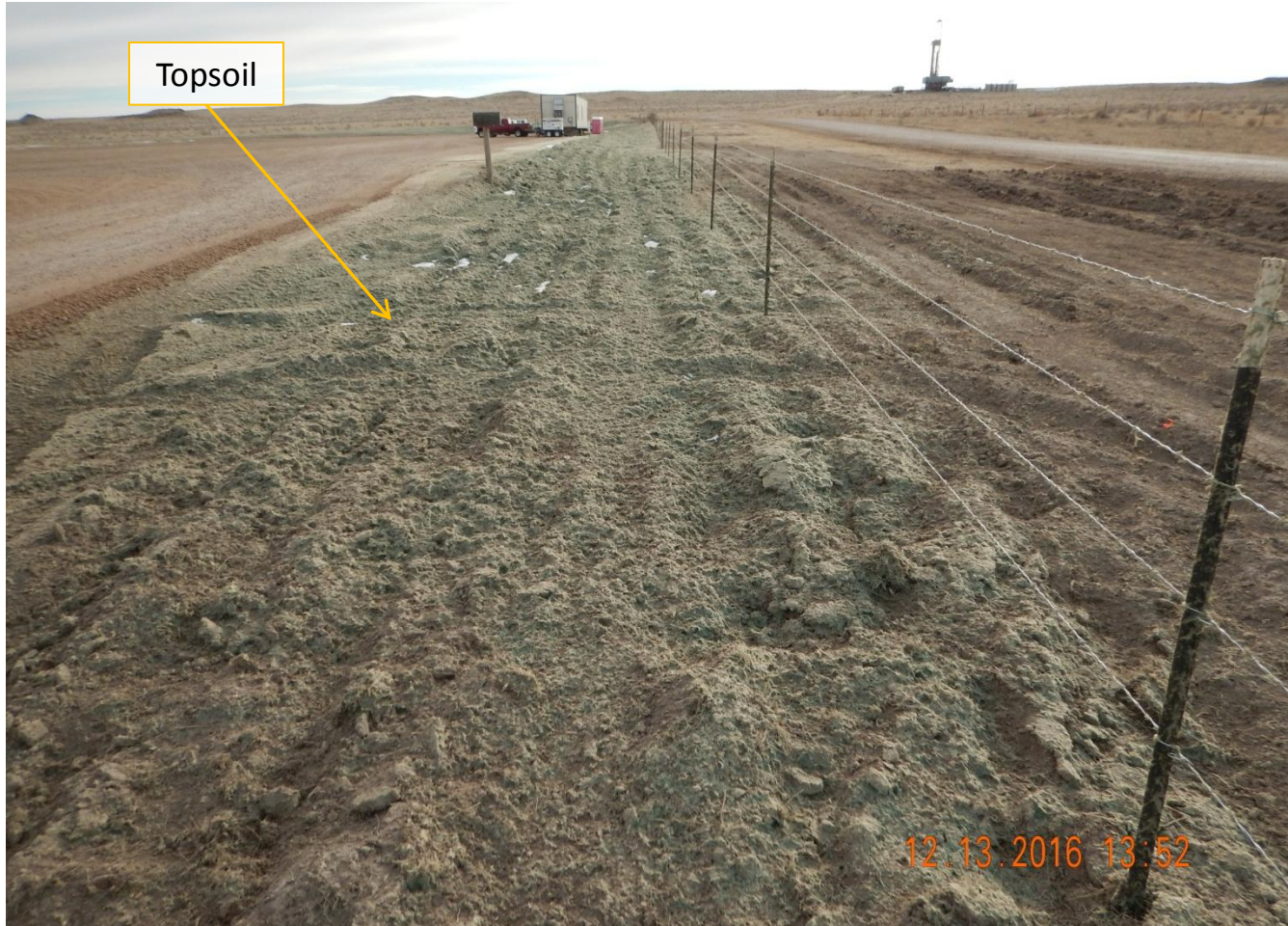
Photo 8. Photo taken from the northwest corner of location, facing South. Based on documentation, topsoil has been stored along the entire perimeter of the location. Tackifier has been applied to the topsoil but areas need additional tackifier because the application rate was too low- see Photos 3 & 4. Also, need to install sufficient stormwater BMPs for the location.
