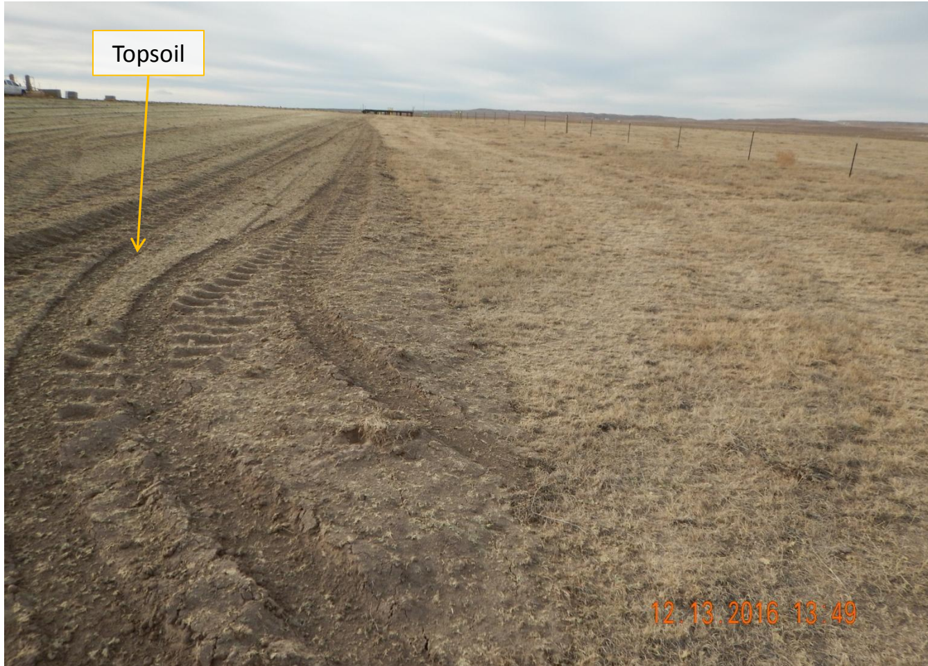
Photo 7. Photo taken from the northern corner of location, facing West. Based on documentation, topsoil has been stored along the entire perimeter of the location. Tackifier has been applied to the topsoil but areas need additional tackifier because the application rate was too low- see Photos 3 & 4. Also, need to install sufficient stormwater BMPs for the location.
