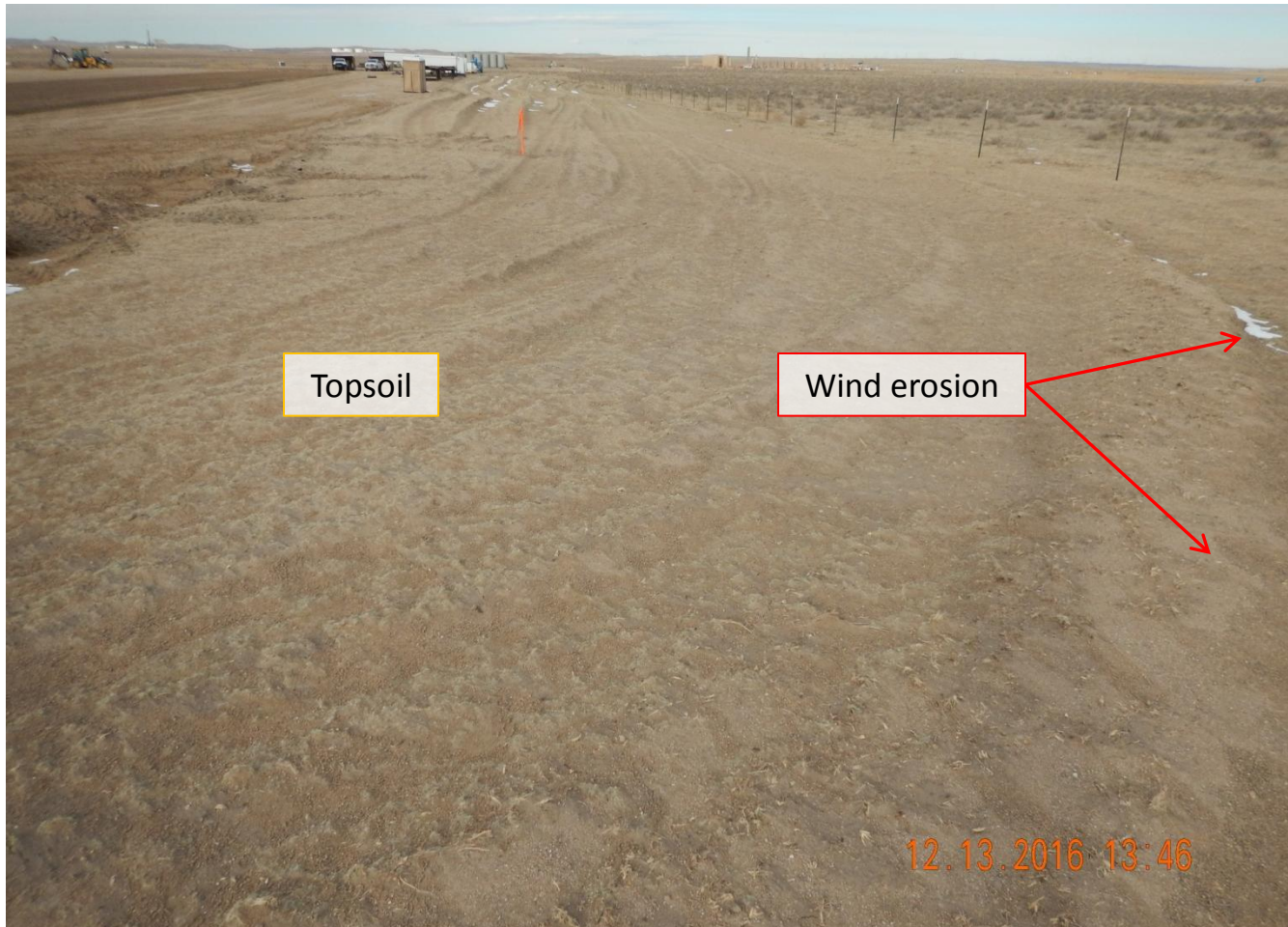
Photo 4. Photo taken from the southeast corner of location, facing North. Based on documentation, topsoil has been stored along the entire perimeter of the location. Tackifier has started to lose its stabilization capability. Need additional tackifier along this area. Also, need to install sufficient stormwater BMPs for the location.
