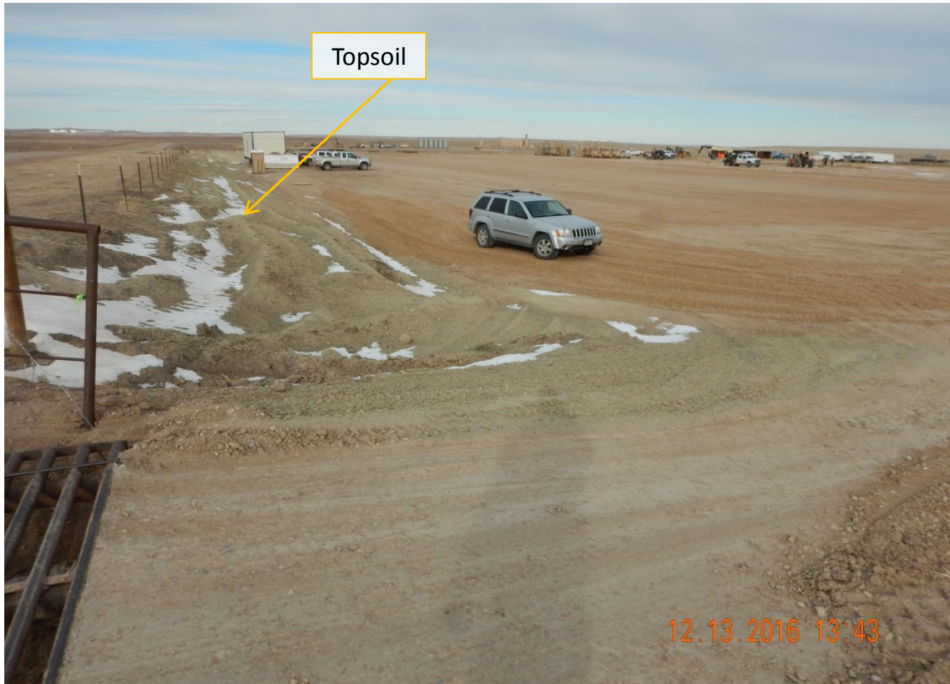
Photo 1. Photo taken from the southwest corner of location, facing North. Based on documentation, topsoil has been stored along the entire perimeter of the location. Tackifier has been applied to the topsoil but areas need additional tackifier because the application rate was too low- see Photos 3 & 4. Also, need to install sufficient stormwater BMPs for the location.
