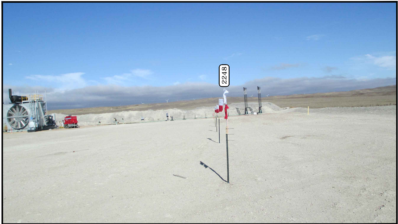
PHOTO: VIEW OF LOCATION STAKES
