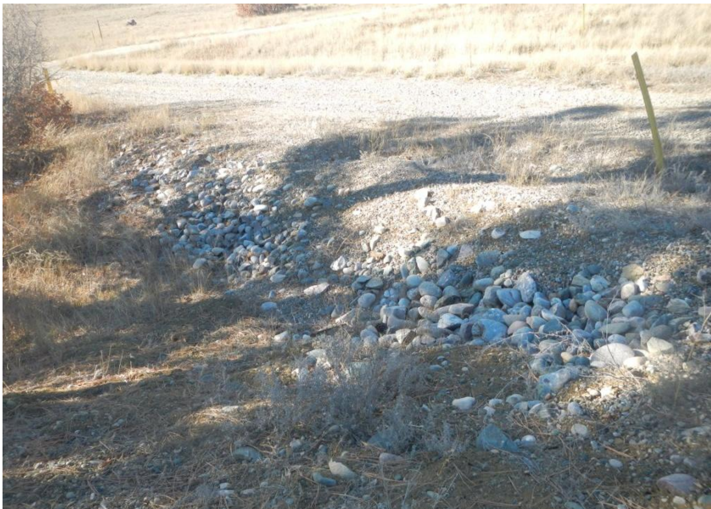
Photo 4. View of cobble armouring along well pad entrance and access ramp appears to be functioning.
