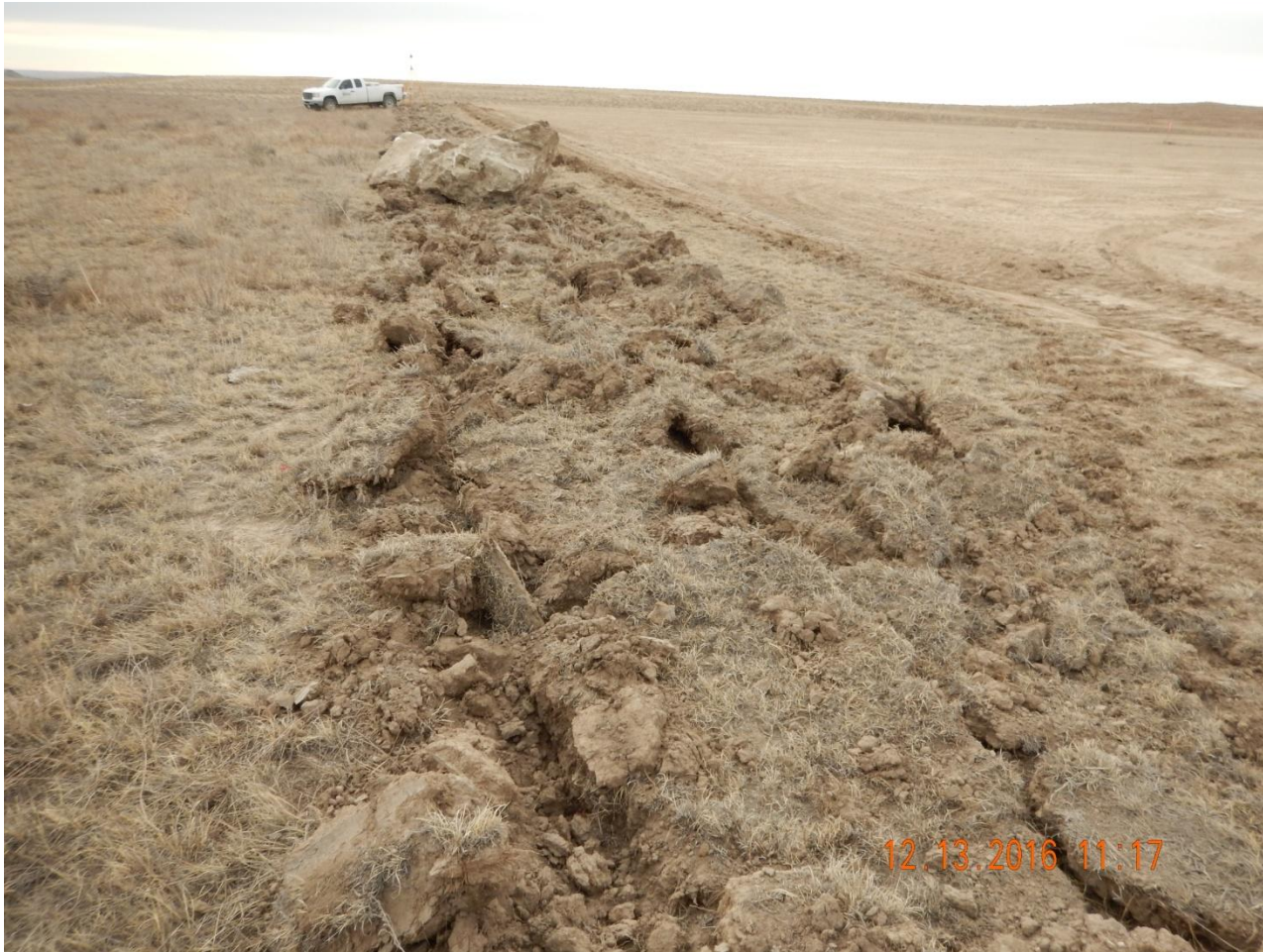
Photo 2. Photo taken from the northeast location, facing South. Temporary BMP, surface roughening, installed around perimeter of location.
