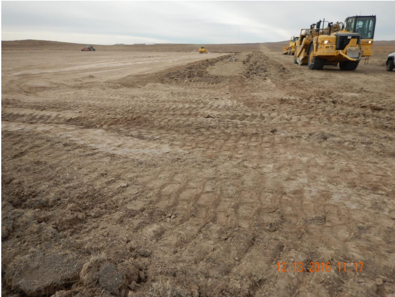
Photo 1. Photo taken from the northeast location, facing West. Temporary BMP, surface roughening, installed around perimeter of location.
