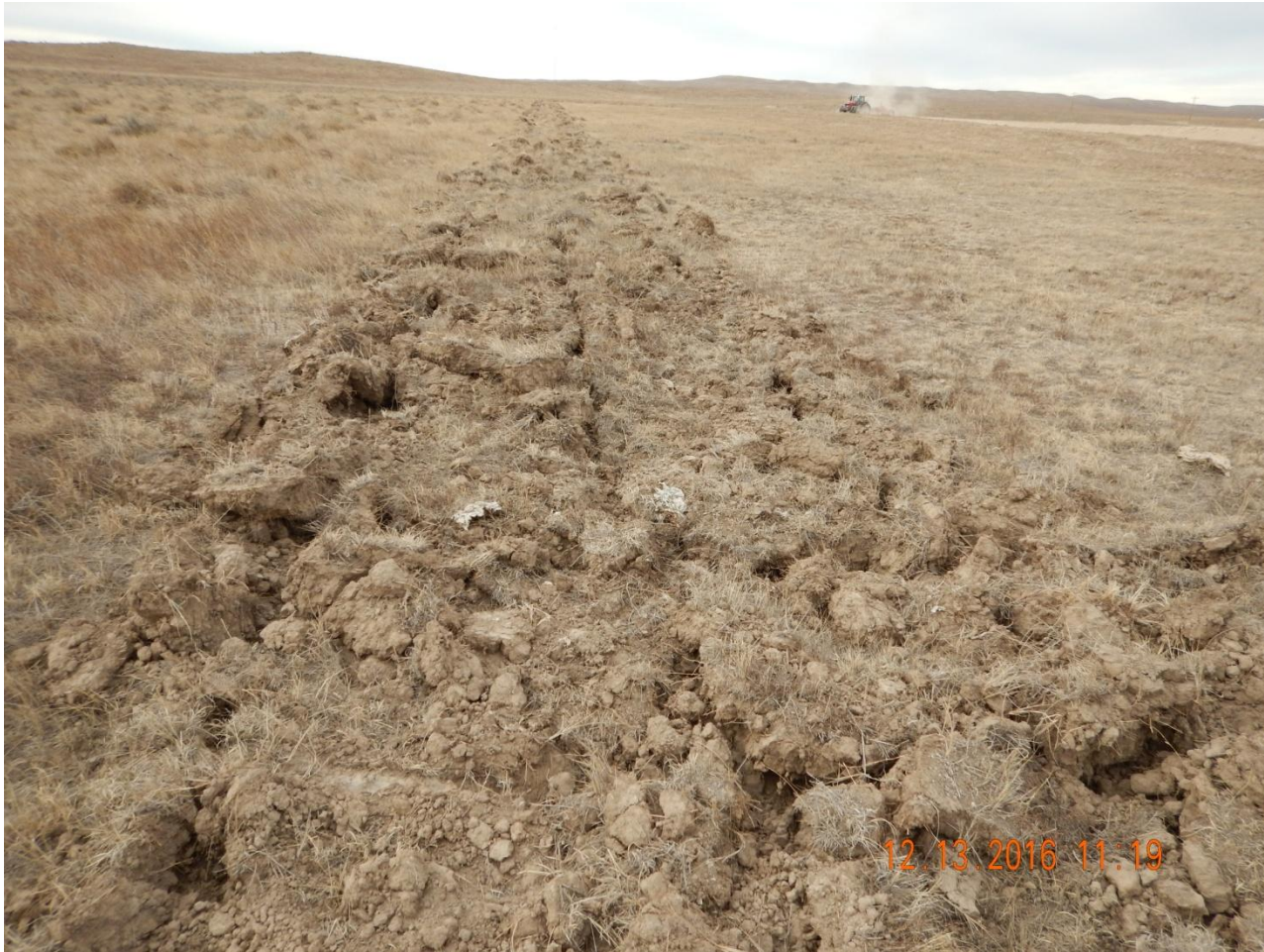
Photo 3. Photo taken from the southeast location, facing West. Temporary BMP, surface roughening, installed around perimeter of location.
