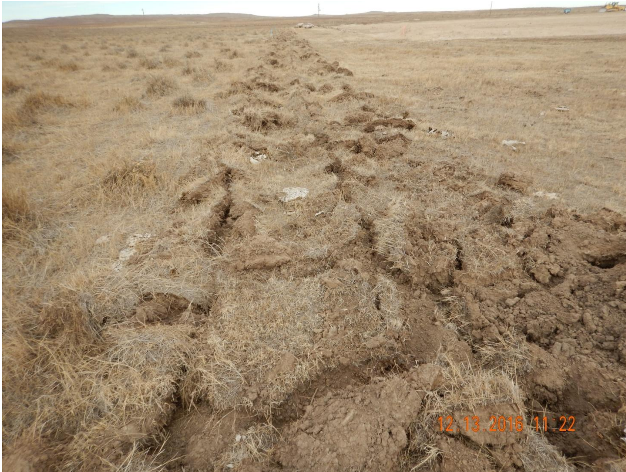
Photo 4. Photo taken from the southwest location, facing North. Temporary BMP, surface roughening, installed around perimeter of location.
