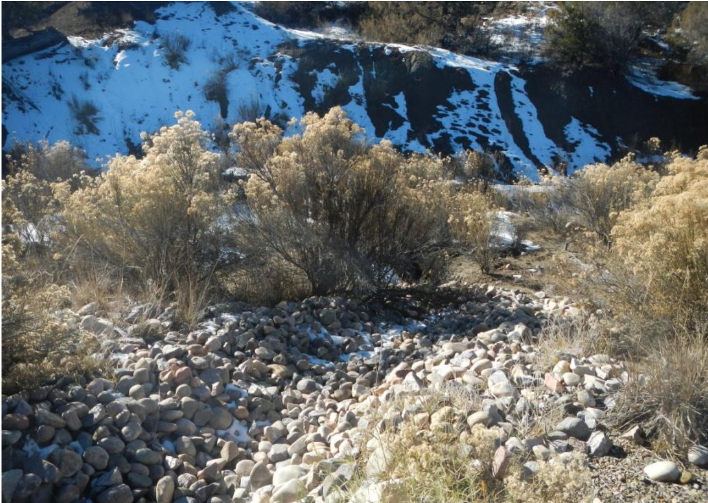
Photo 5. View of cobble run-down in the southwestern corner of the project area appears to be functioning at this time.
