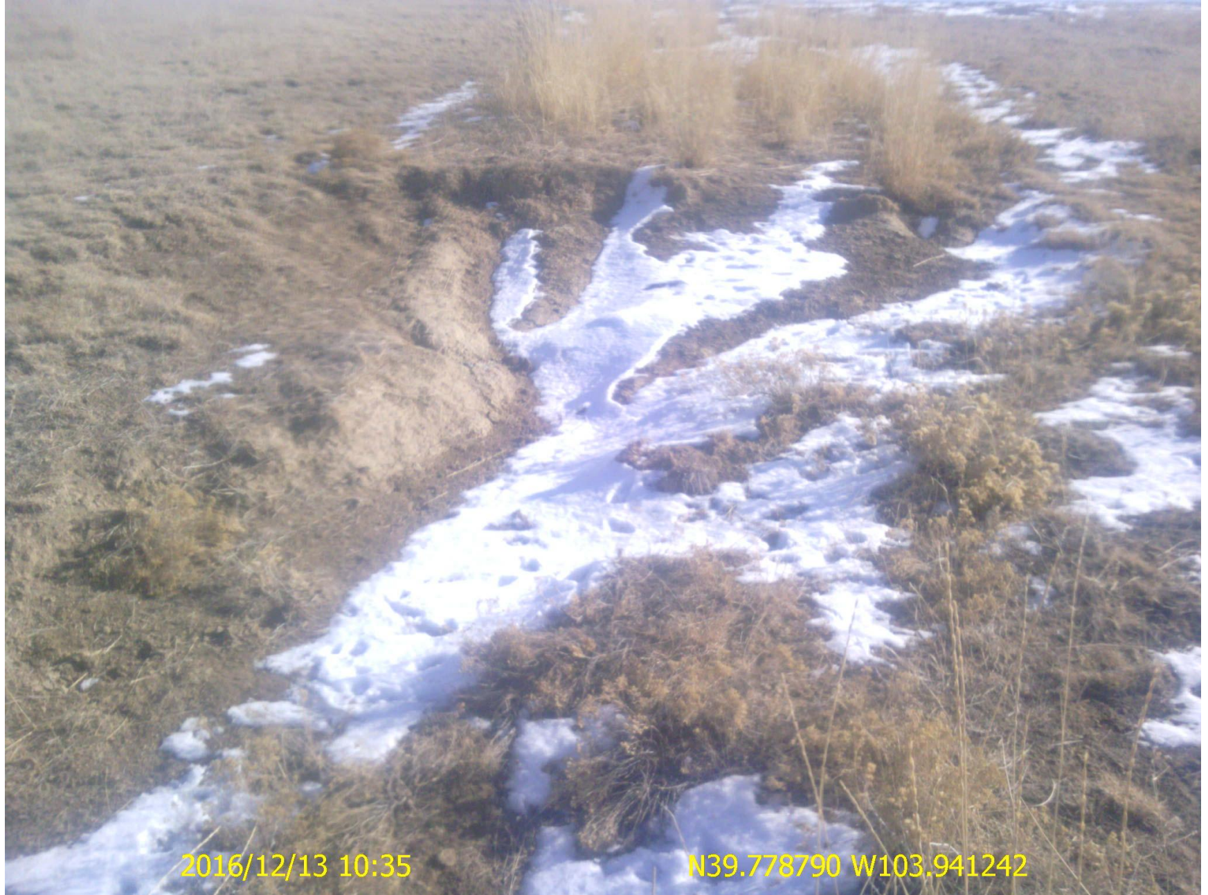
Figure 4: Photo taken from the northern disturbance area, facing east towards the access road. Photo shows erosion has not been stabilized. Refer to photos from inspection Doc. # 682500938 for additional details.
