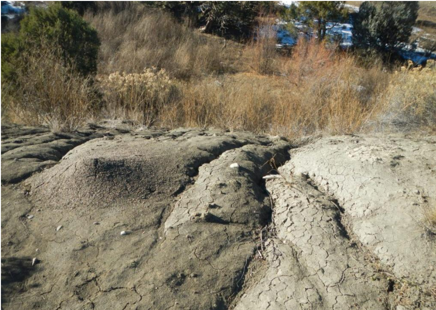
Photo 6. View of rilling that is occurring in the eastern fill slope. Additional reinforcement is needed to reduce the energy of surface flows from the well pad.
