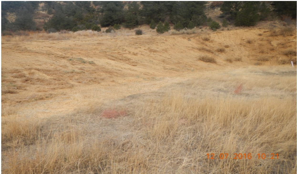
photo 3: Facing toward the northwest cut slope which was seeded and hydro-mulched.
