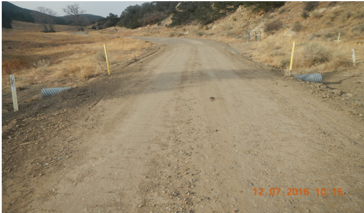
photo 3: Facing southwest along the main access road. Gravel was applied and the culvert is maintained.
