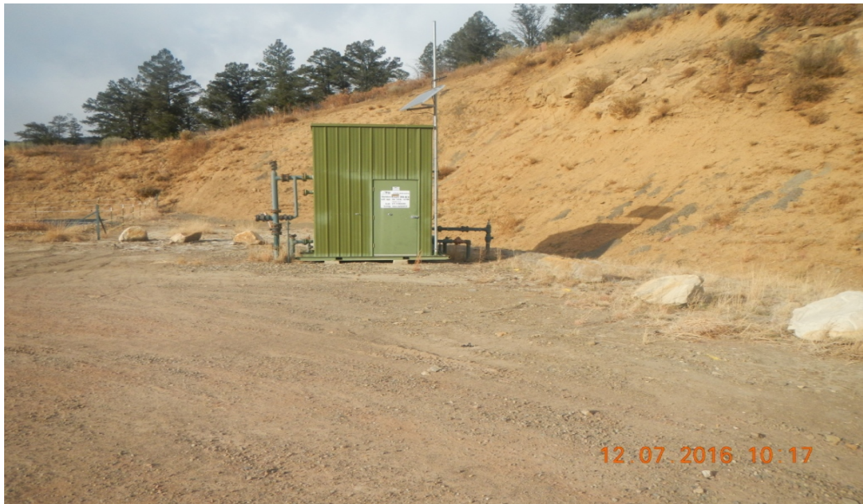
photo 6: Facing southwest toward the location. The cut slope has been seeded and hydromulched.
