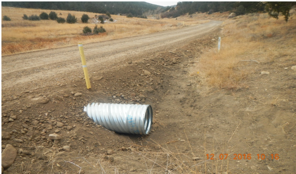
photo 5: A new culvert was installed along the road.
