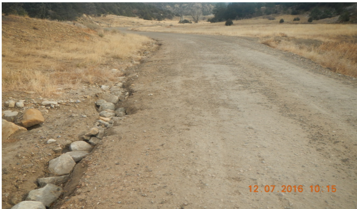
photo 4: Facing back to the northeast along the road. Erosion along the side of the road was repaired.
