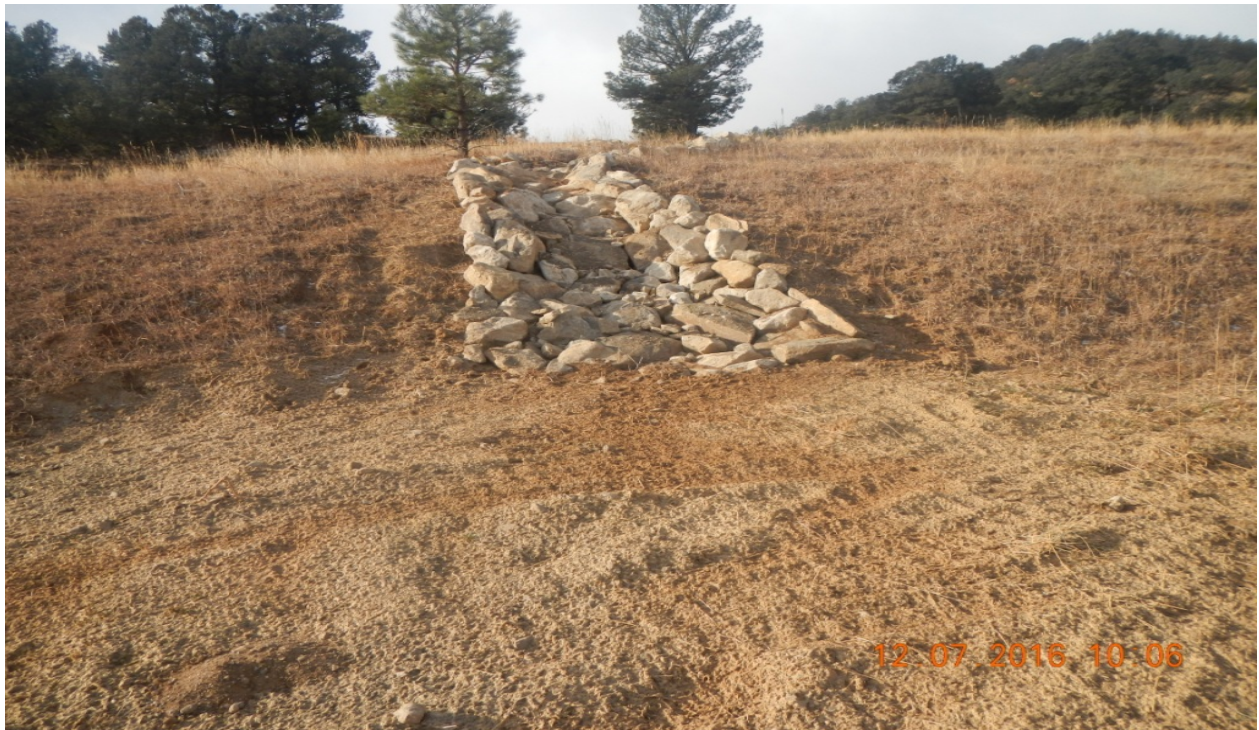
photo 1: Rock rip/rap has been added to area near the access road.
