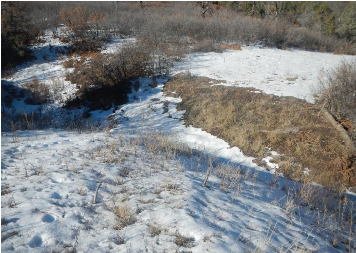
Photo 1. View of recontoured drainage near beginning of access road appears to be functioning and revegetation progressing.
