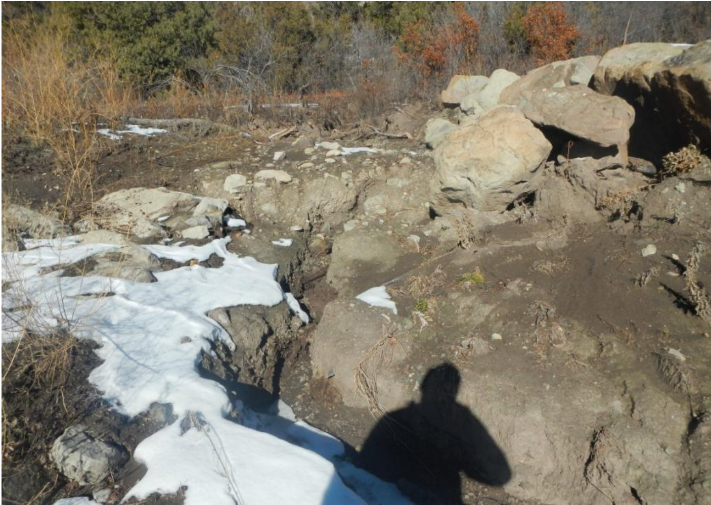
Photo 11. View of area on re-routed drainage within the northeastern portion of the well pad that is not sufficiently armored and erosion is occurring.
