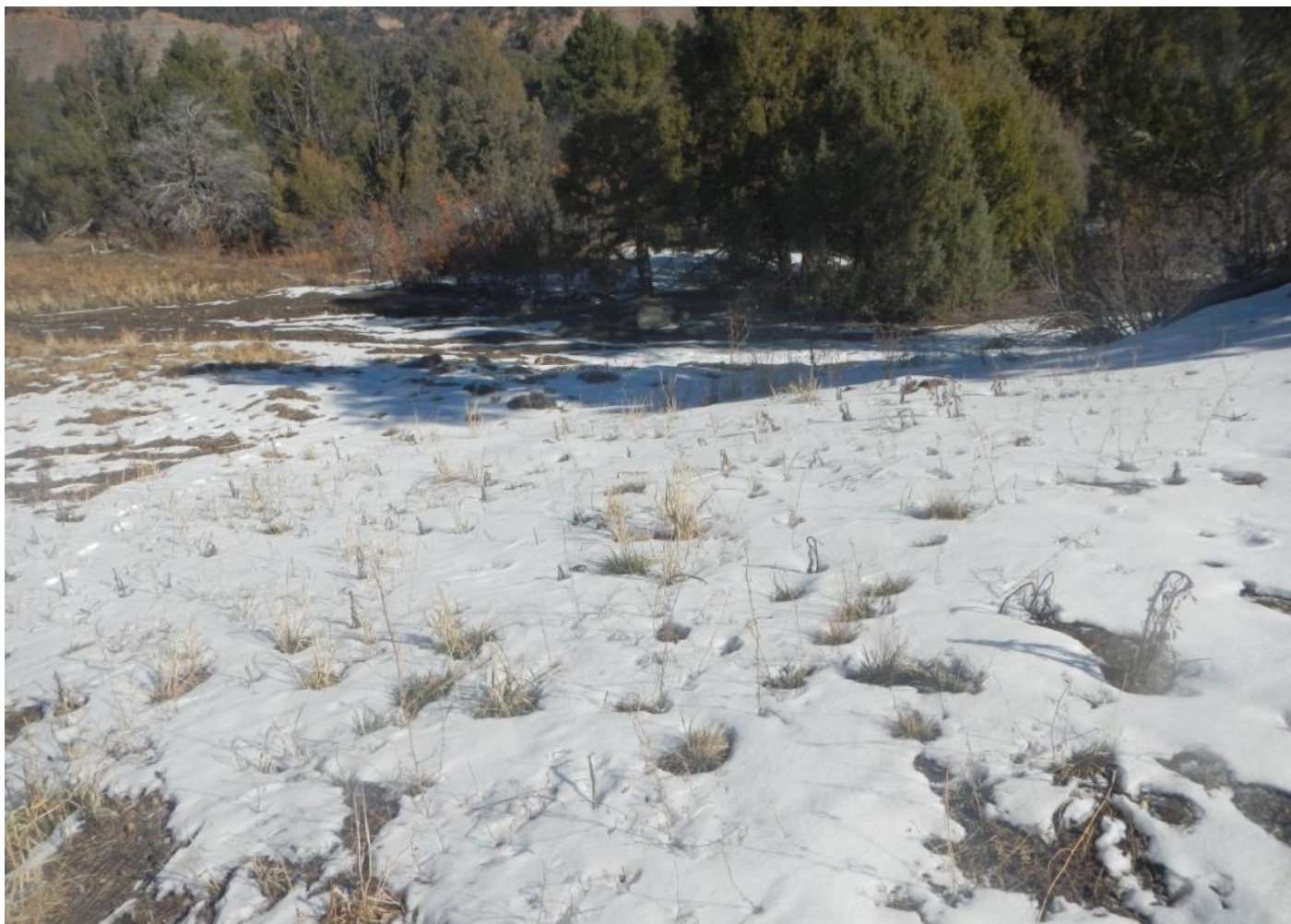
Photo 13. Overview of area shown in Photo 12 that slopes toward the contoured drainage. It appears that surface flows are causing erosion near the banks of the re-routed drainage.
