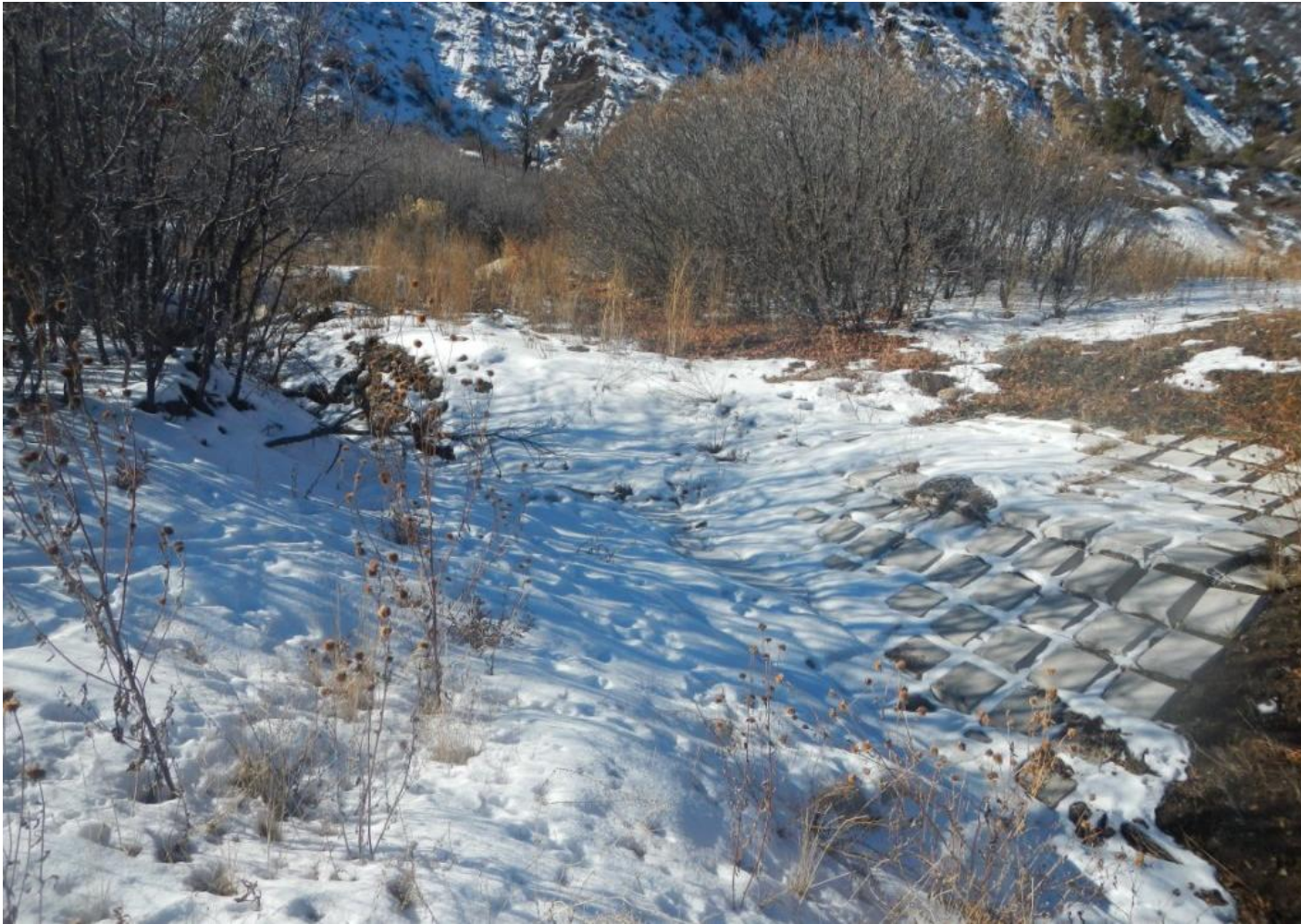
Photo 5. View of channel that was reclaimed and stormwater controls installed near the entrance to the well pad.
