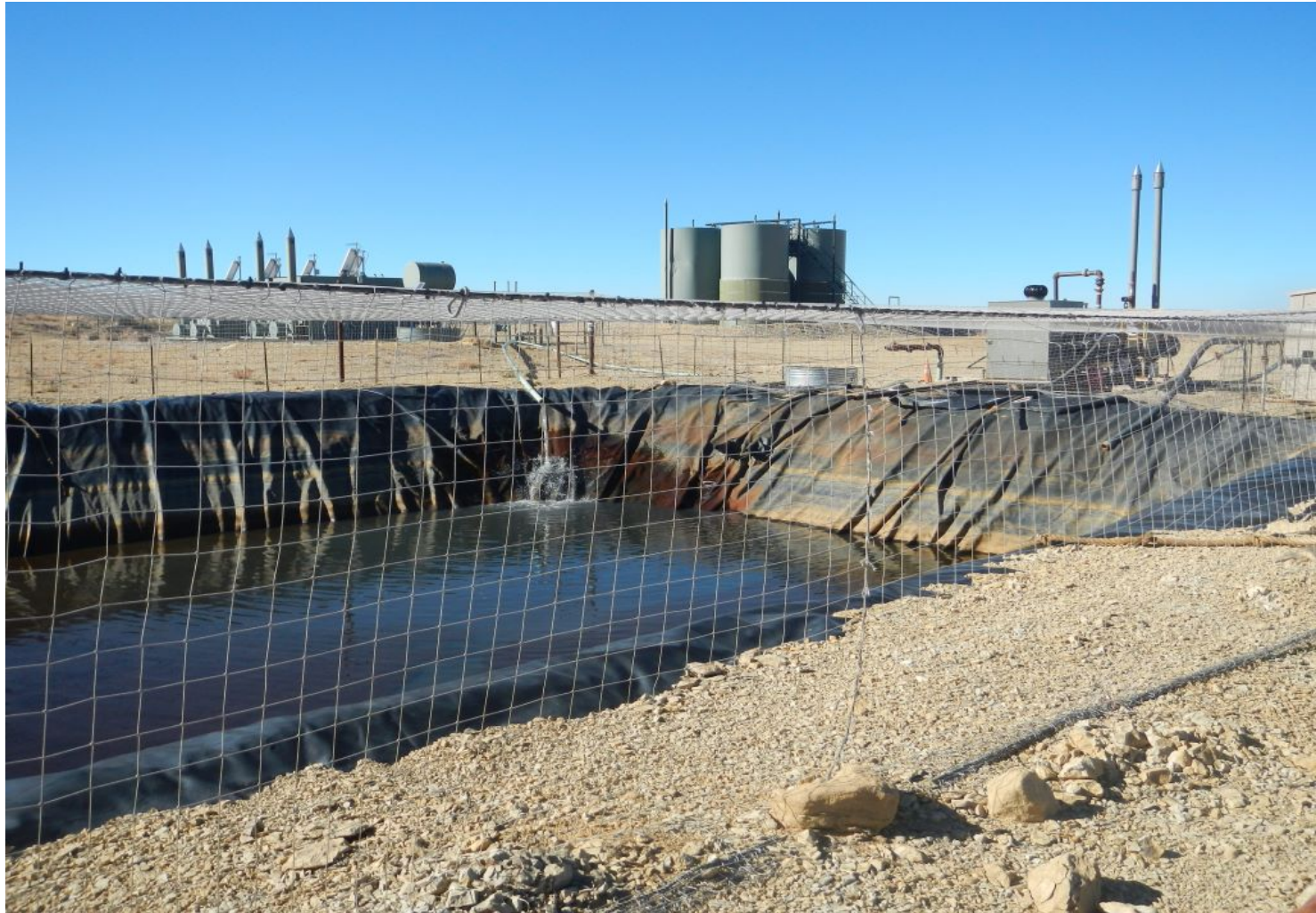
Photo#4: Pit on Location; netted and Fenced
