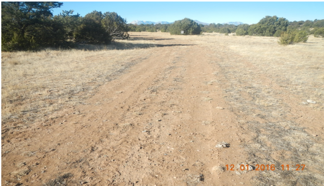
photo 2: Facing west along the former access road. The vegetation has not adequately established.
