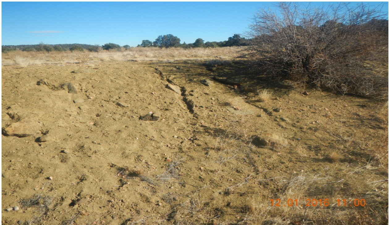
photo 8: There are signs of erosion along west side of the pad.
