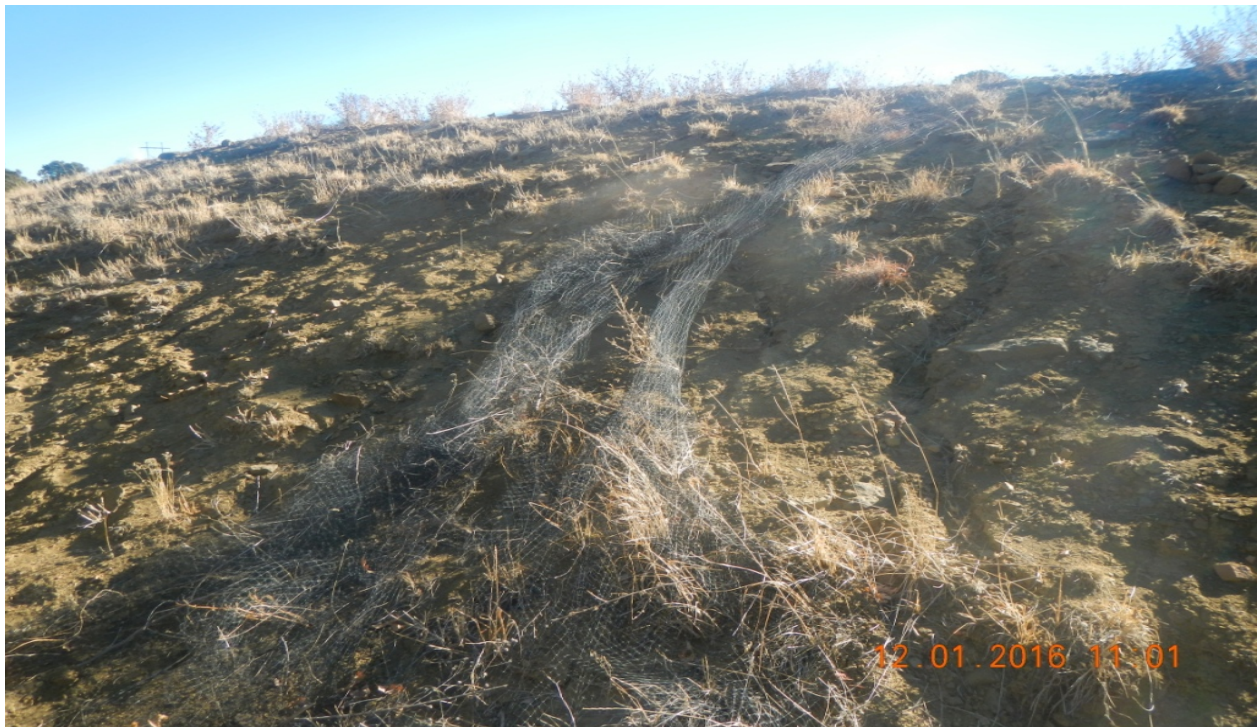
photo 6: The fill slope is not adequately stabilized with vegetation and there are signs of erosion. The plastic netting debris remains.
