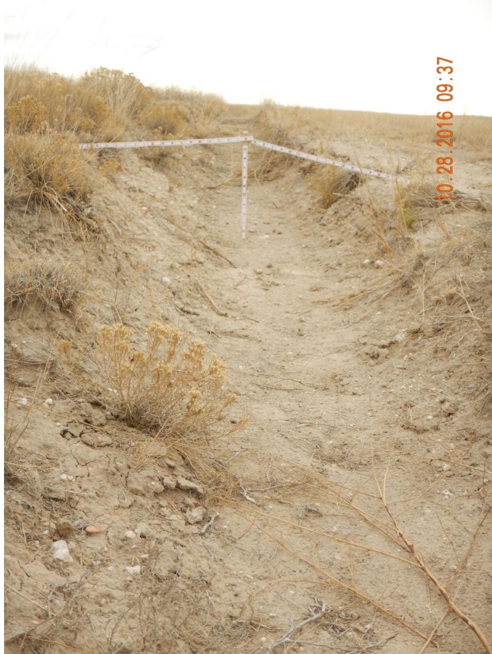
Figure 13: Photo taken from the access road entrance, on the east end of the location, facing east. Photo shows areas where erosion has deepened the ruts in the access road. Measuring stick for reference.
