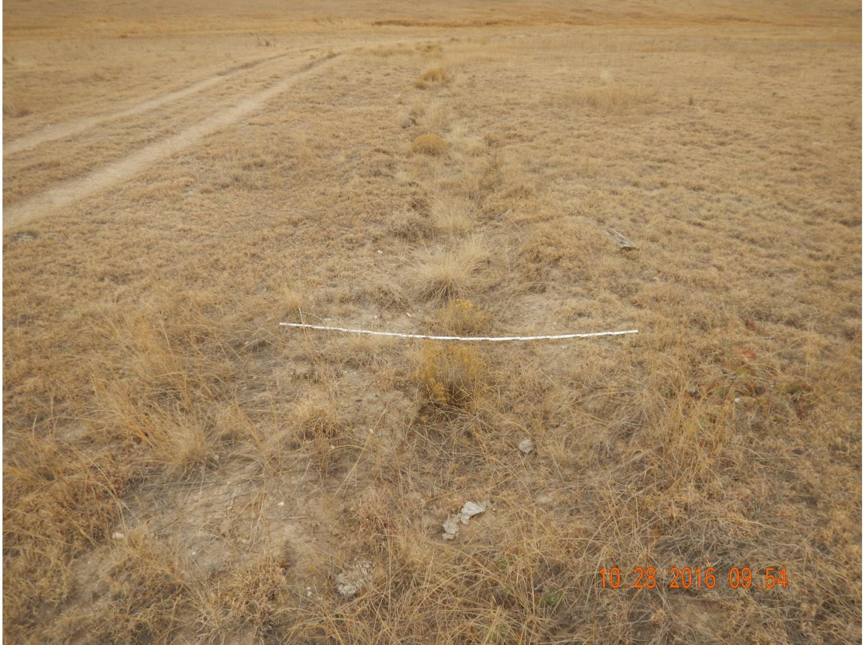
Figure 17: Photo taken west of the location, facing west. Photo shows gully formed by stormwater originating from the location. 6' measuring stick for reference.
