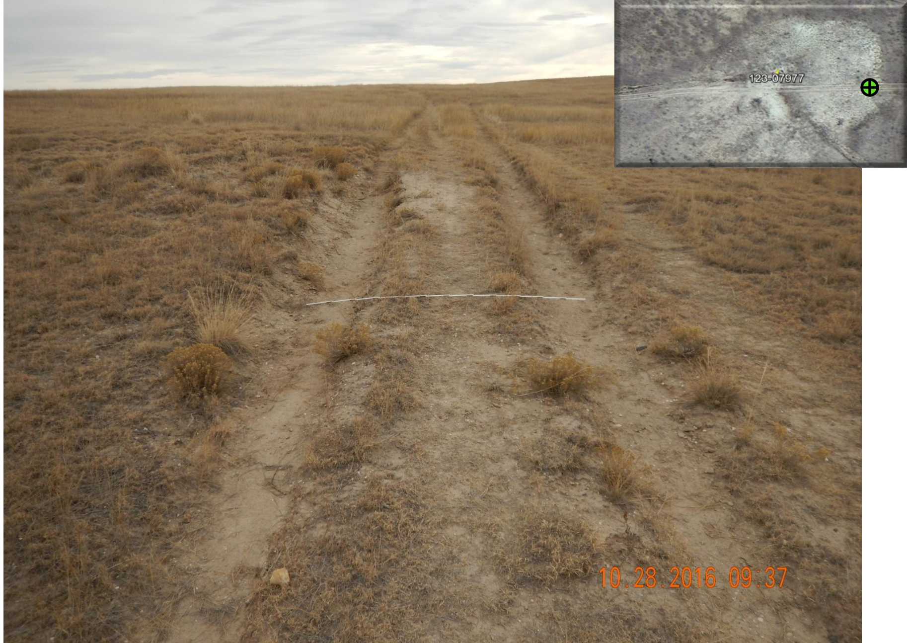
Figure 12: Photo taken from the access road entrance, on the east end of the location, facing east. Photo shows areas where erosion has deepened the ruts in the access road. 6' measuring stick for reference.
