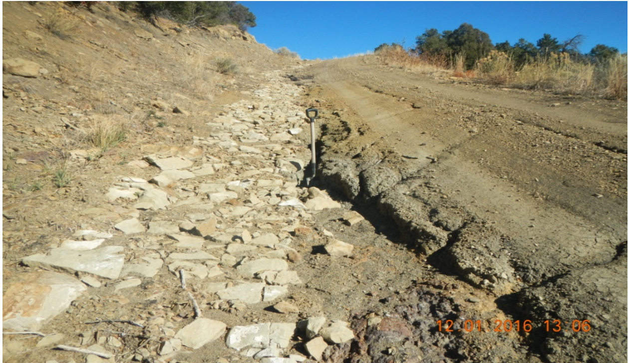
photo 5: Erosion is occurring along the rock rip/rap cutting into the road. It appears sediment has filled into the rip/rap.
