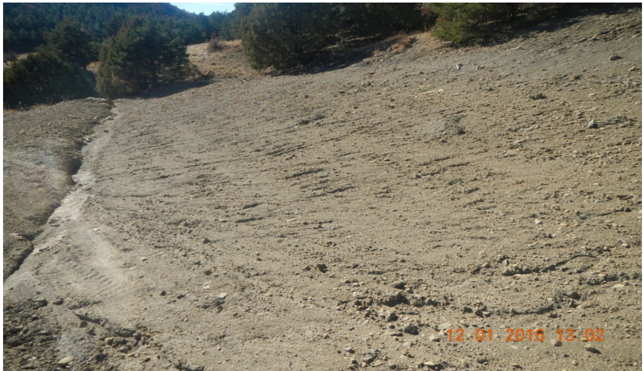
photo 4: The disturbance along the side of the road has not been reclaimed and stabilized.
