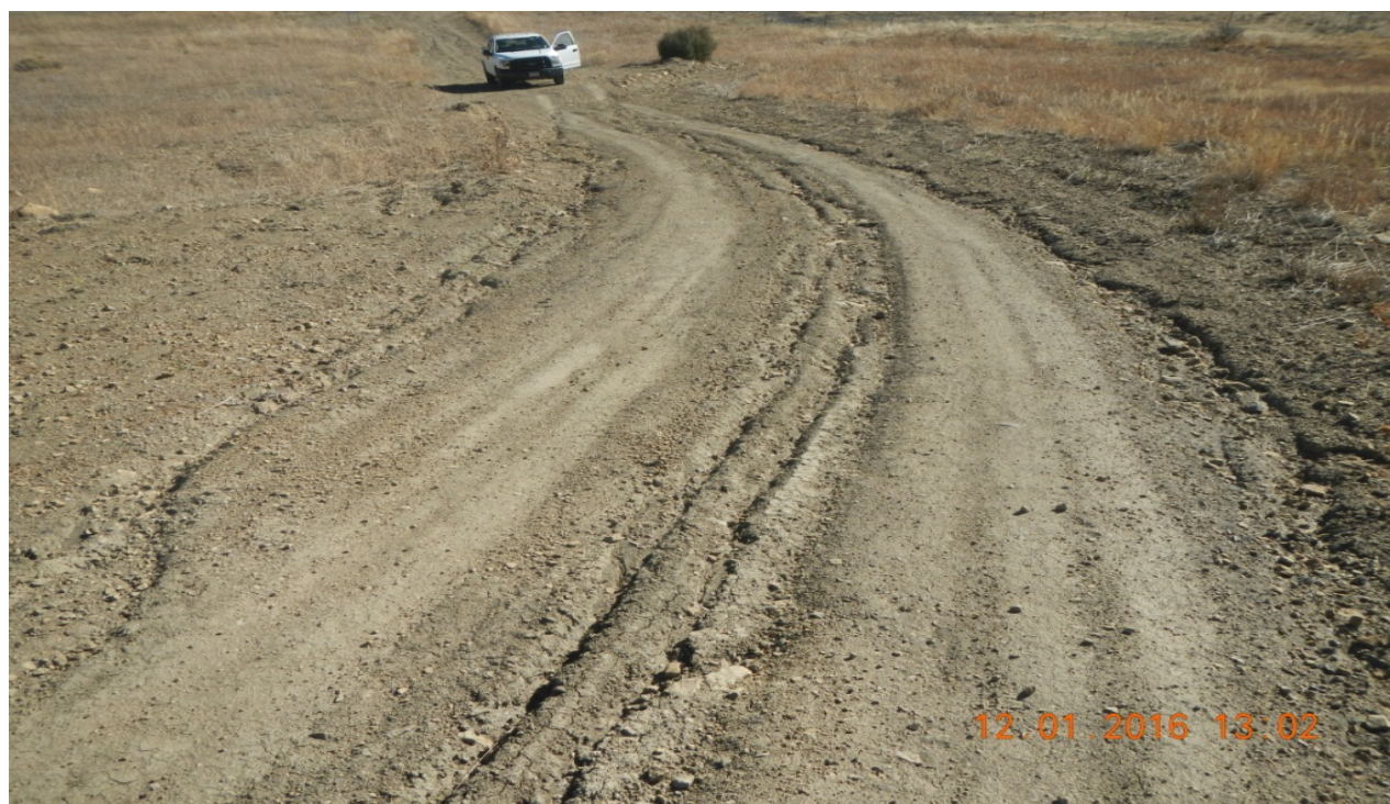
photo 2: Facing back to the southeast along the access road. There are signs of erosion occurring down along the road.
