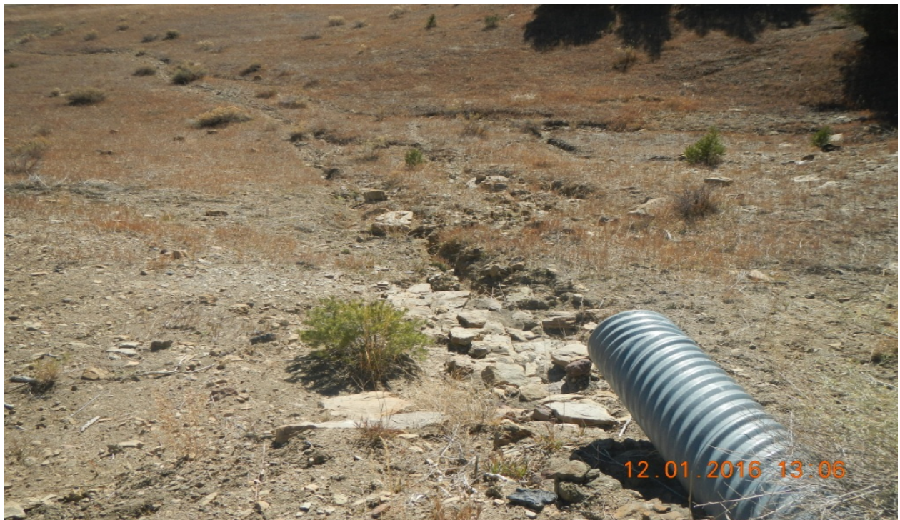
photo 6: Stormwater draining from the culvert is creating erosion out into the pasture.
