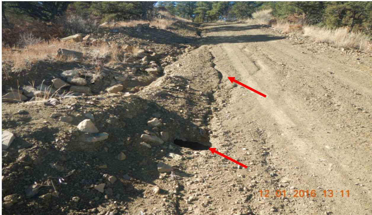
photo 7: There are signs where stormwater is not draining towards the culvert, instead flowing down the road. There is a hole in the culvert where bottom red arrow points to.
