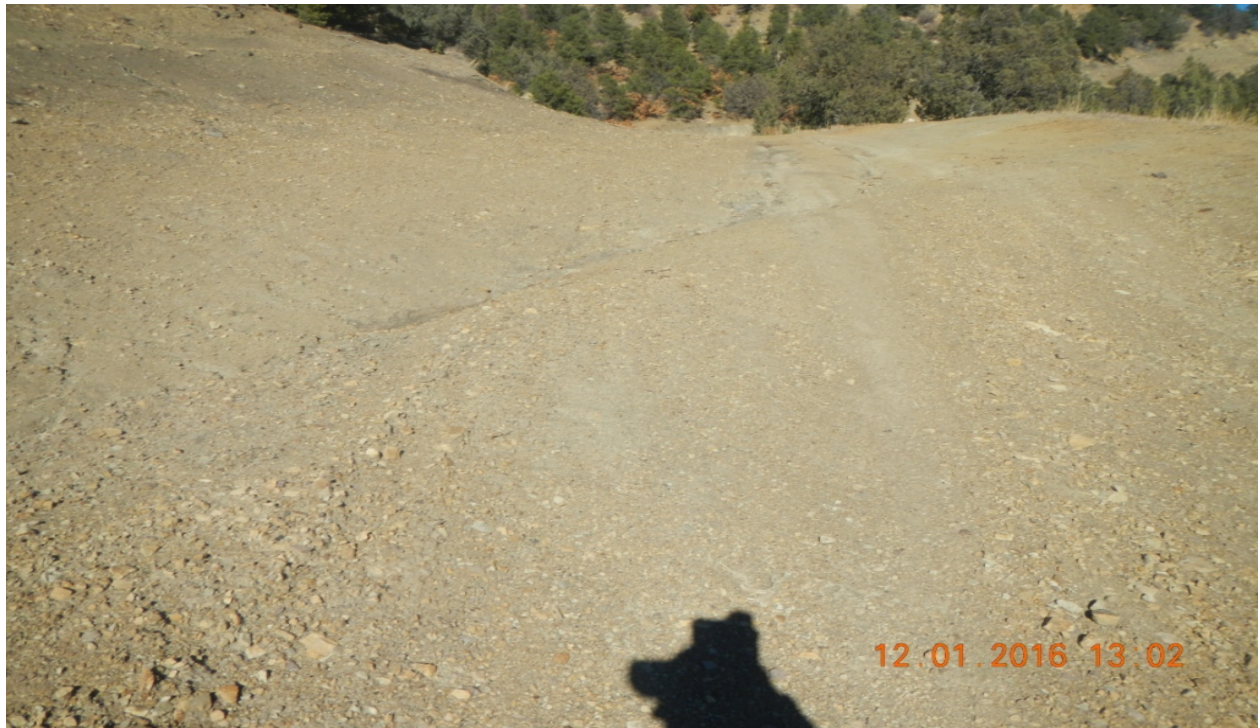
photo 3: There are water bars placed along the road.
