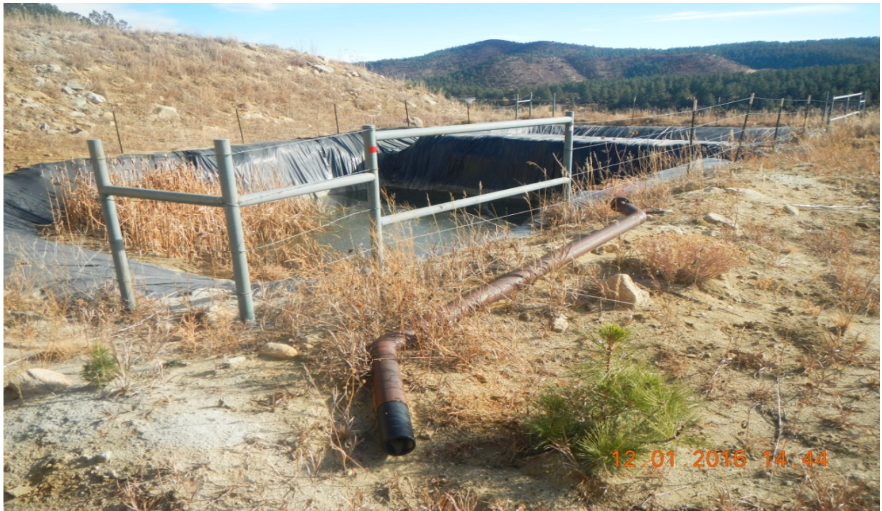
photo 7: The lined pit remains at the east side of the location.
