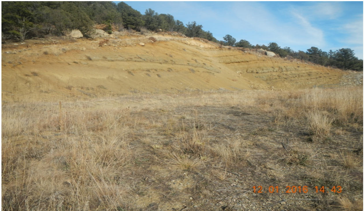
photo 5: Facing northeast toward the cut slope of the location.
