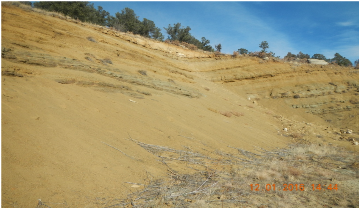
photo 6: Facing northeast toward the cut slope of the location.
