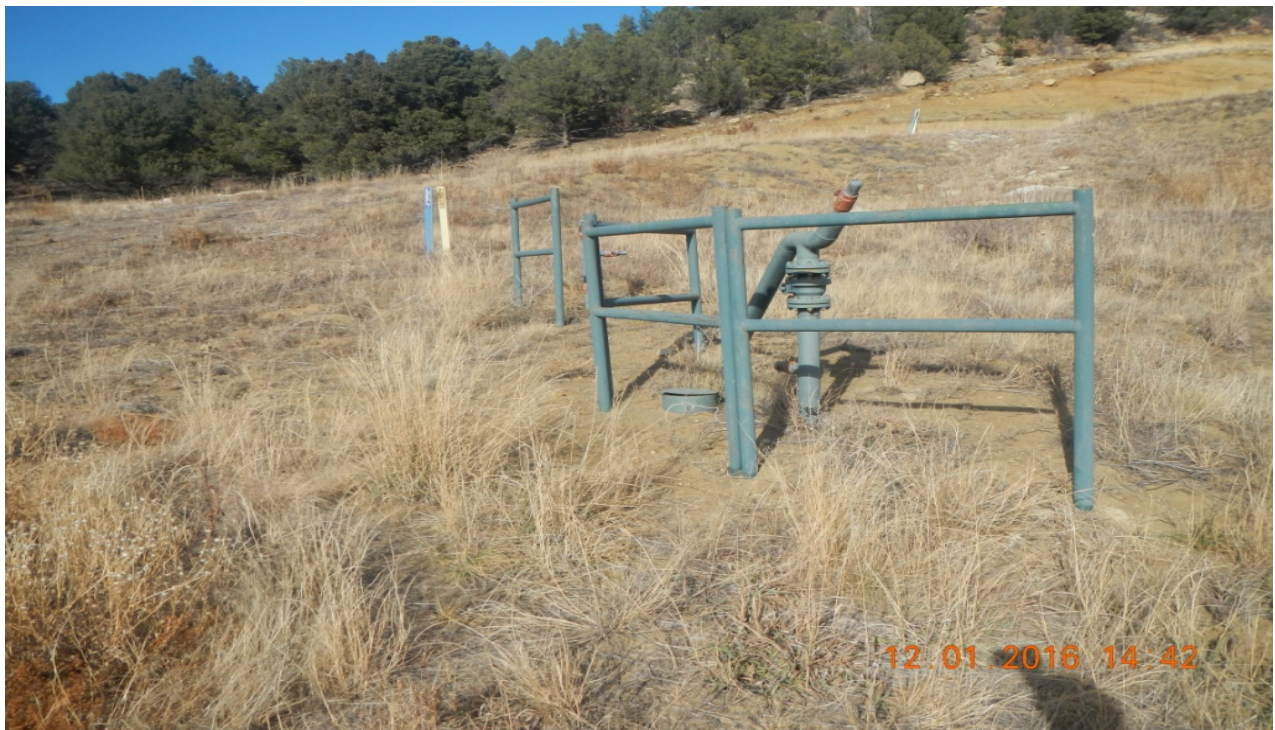
photo 2: Pipe risers remain near the location.
