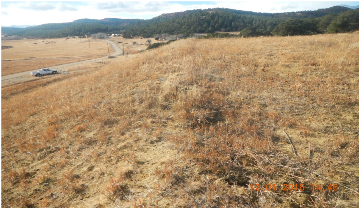
photo 10: Facing west along the south fill slope.
