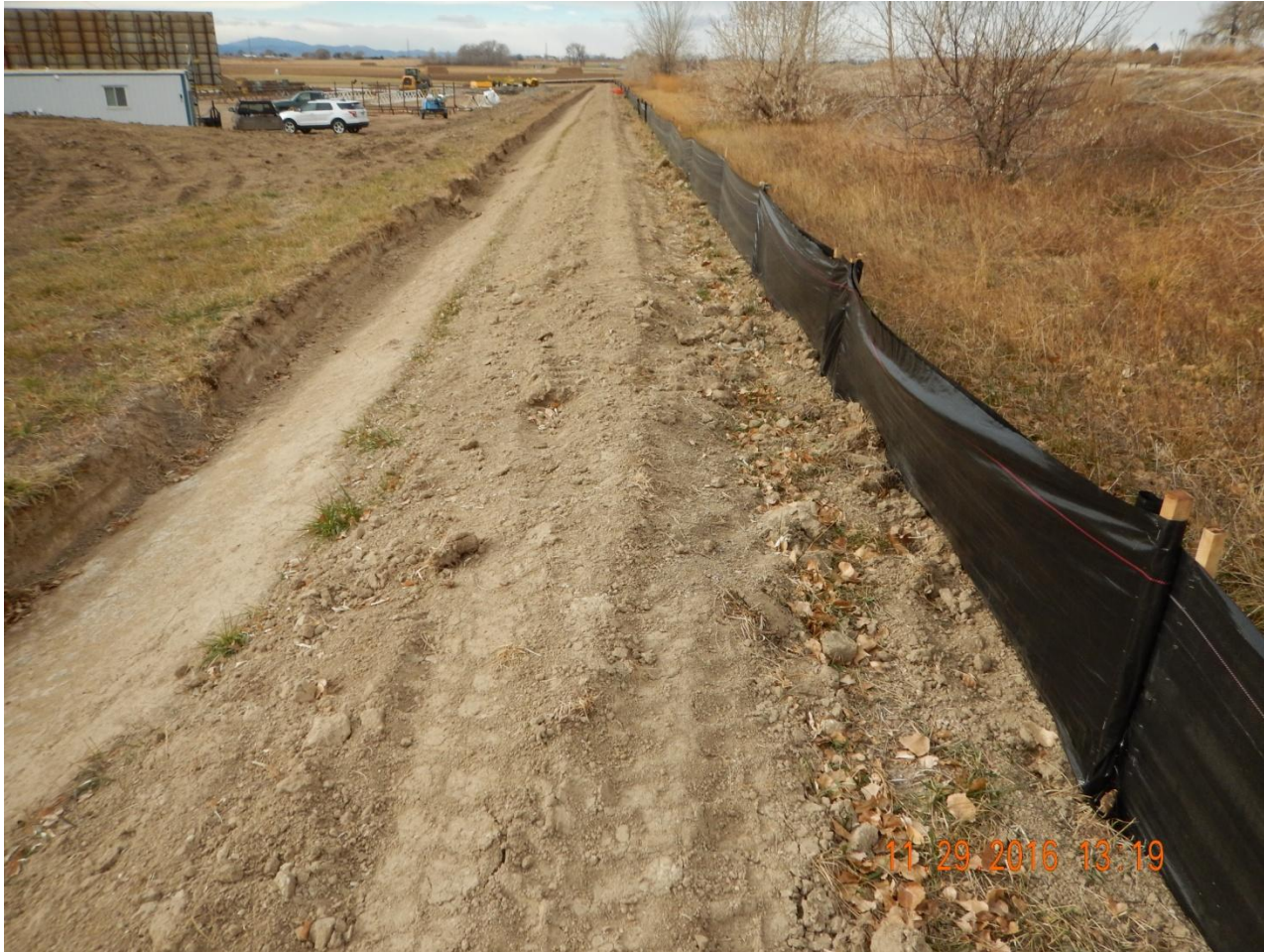
Photo 8. Photo taken from the northeast location, facing West. Ditch and berm installed around the perimeter of location with the addition of a silt fence installed around perimeter of location.
