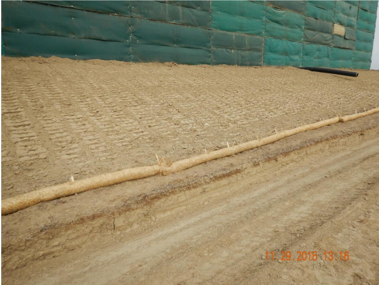
Photo 5. Photo taken from the southern location, facing North. Fill slope has been stabilized and additional, temporary BMP (i.e., wattle) installed at toe of the slope.
