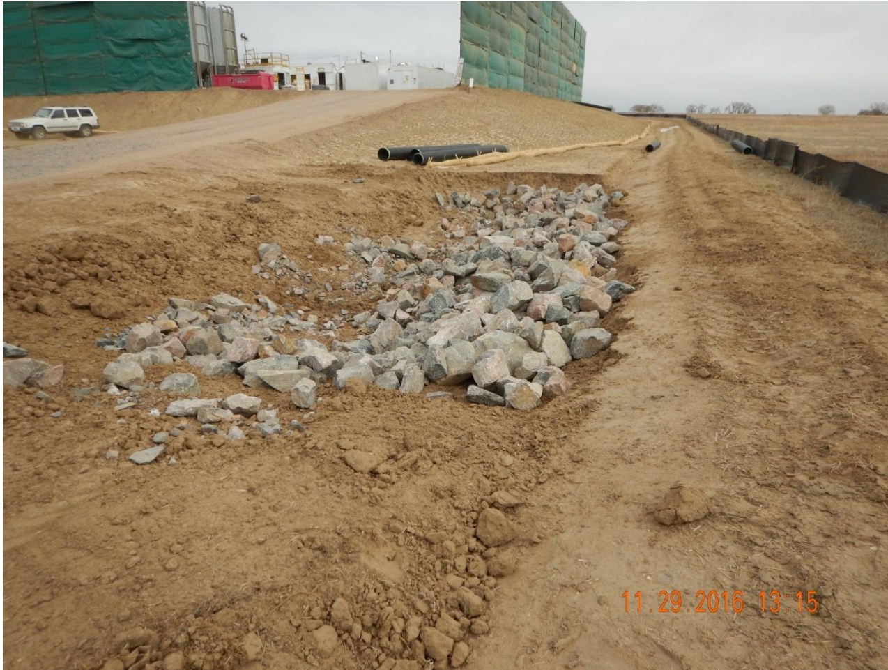
Photo 4. Photo taken from the southwest location, facing East. Ditch and berm installed around the perimeter of location with a sediment trap or retention pond IN-PROCESS. Silt fence installed around perimeter of location.
