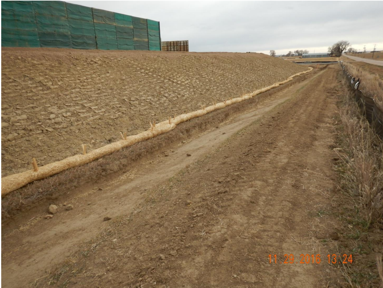
Photo 10. Photo taken from the western location, facing Southeast. Fill slope has been stabilized and additional, temporary BMP (i.e., wattle) installed at toe of the slope.
