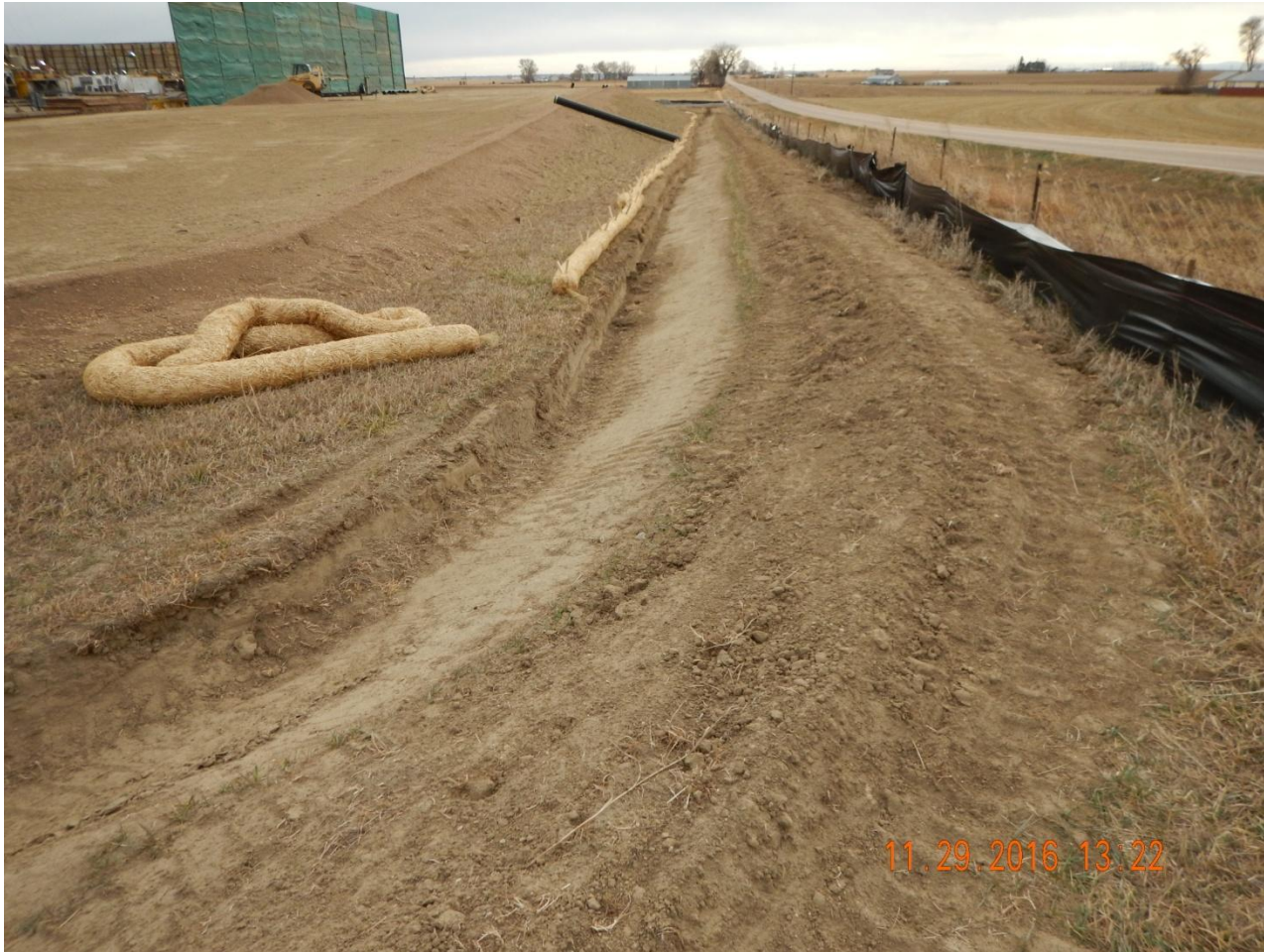
Photo 9. Photo taken from the northwest location, facing South. Ditch and berm installed around the perimeter of location with the addition of a silt fence installed around perimeter of location.
