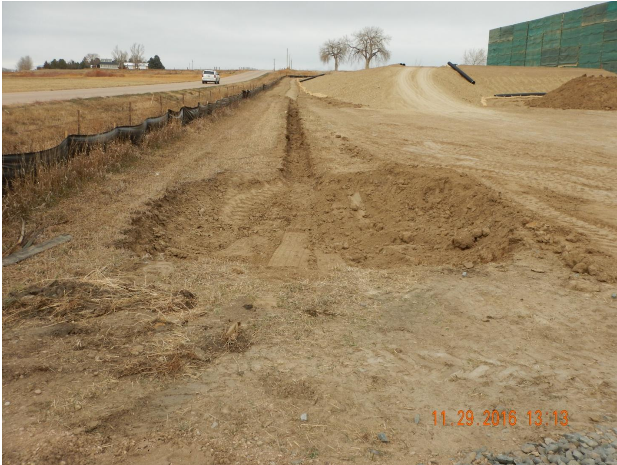
Photo 3. Photo taken from entrance of location, facing North. Sediment trap or retention pond IN-PROCESS. Silt fence installed around perimeter of location.
