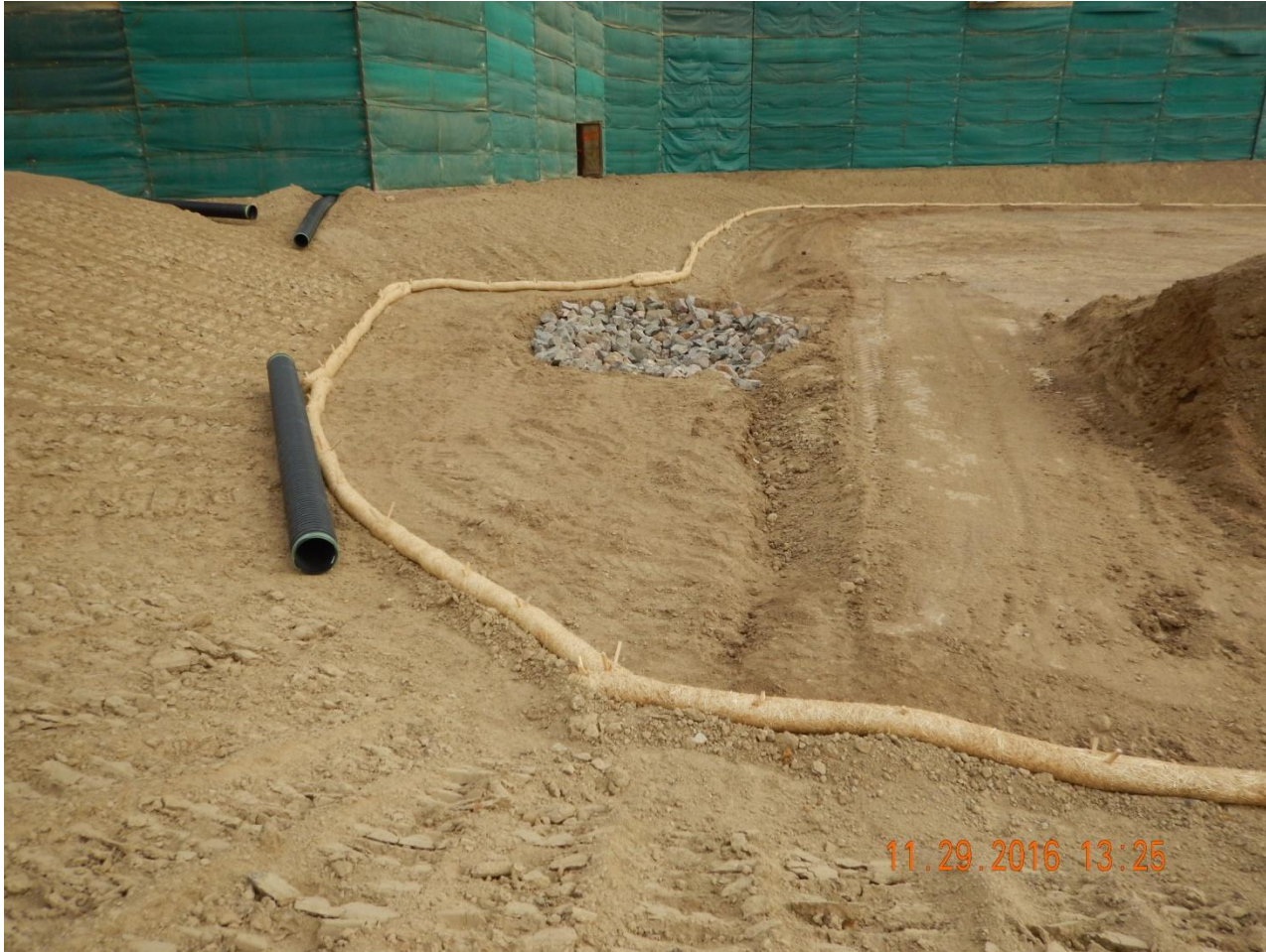
Photo 11. Photo taken from the western location, facing East. Retention pond installed at base of slope, fill slope stabilized with additional, temporary BMP (i.e., wattle) installed at toe of the slope.
