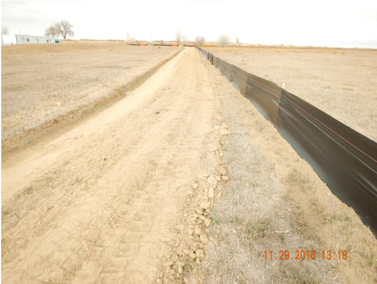
Photo 7. Photo taken from the eastern location, facing North. Ditch and berm installed around the perimeter of location with the addition of a silt fence installed around perimeter of location.
