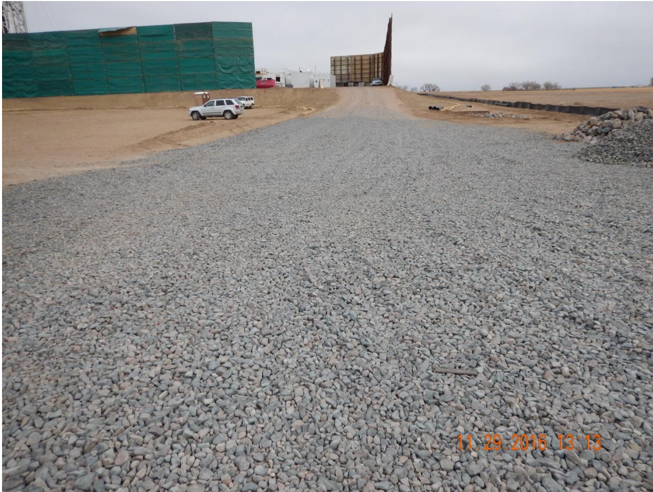
Photo 2. Photo taken from the entrance of location, facing East. Gravel installed to help control vehicle tracking and transport of sediment offsite.
