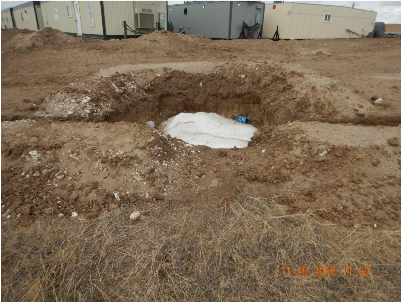
Photo 1. Photo taken from the southeastern location, facing West, towards the sediment trap. Sediment trap does not have a stabilized outlet.
