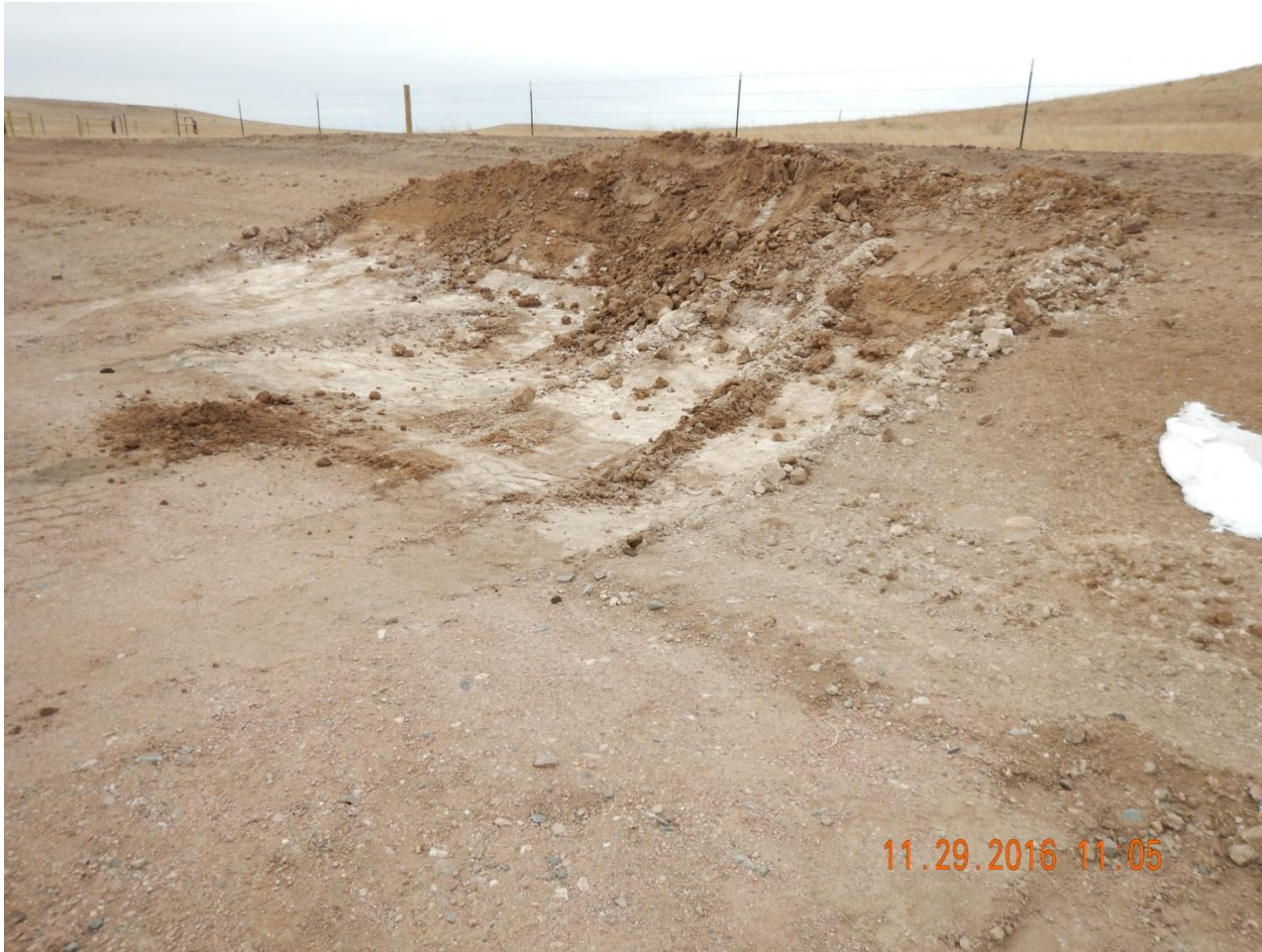
Photo 6. Photo taken from the south, western location , facing South. Stabilize the cut slope where soil was moved.
