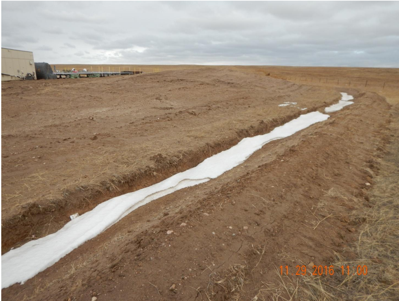
Photo 2. Photo taken from the eastern location, facing West, towards the topsoil stockpile. Topsoil has not been stabilized and protected from degradation due to wind and water erosion.
