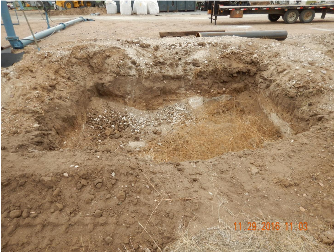
Photo 4. Photo taken from the northern location, facing South, towards the sediment trap. Sediment trap does not have a stabilized outlet.
