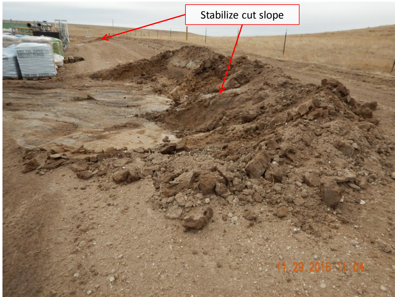
Photo 5. Photo taken from the north, western location , facing South. Stabilize the cut slope where soil was moved.
