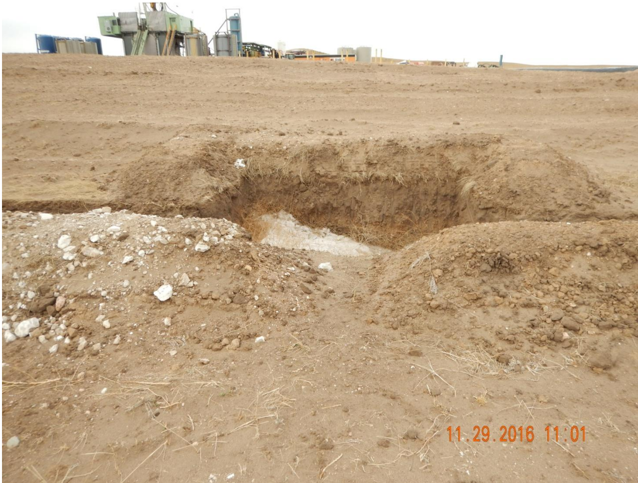
Photo 3. Photo taken from the northeastern location, facing West, towards the sediment trap. Sediment trap does not have a stabilized outlet.
