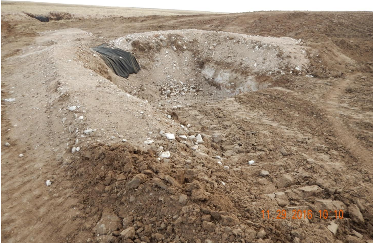
Photo 3. Photo taken from the northeastern location, facing East, towards the sediment trap. Sediment trap side slopes should not be steeper than 2:1 and the inlet and outlet should be stabilized. Berms around sediment trap have been stabilized.
