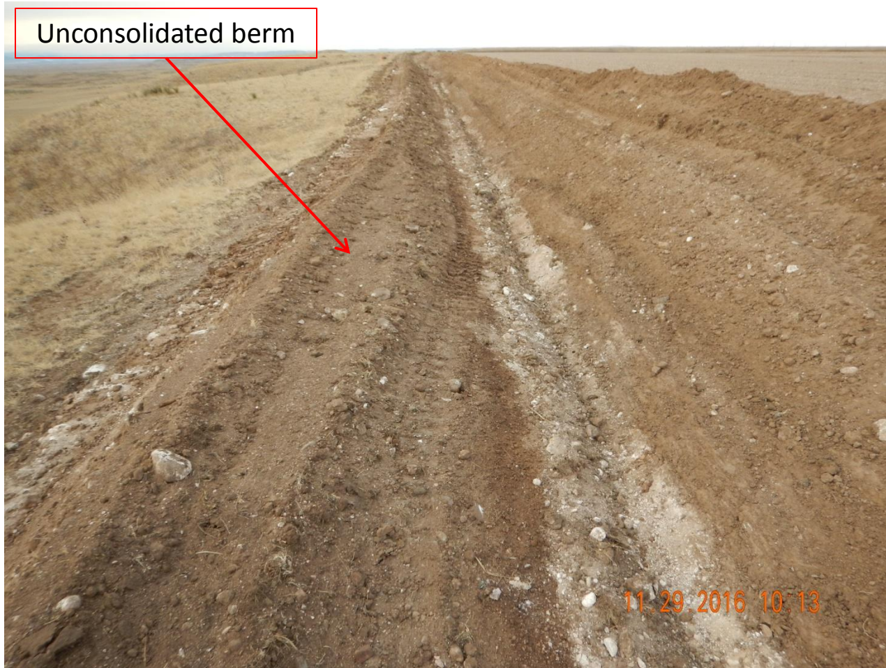
Photo 5. Photo taken from the southern location , facing West. Ditch and berm BMP installed around the location perimeter. Berm shall be compacted to ensure containment of sediment laden storm runoff is directed to the sediment trap.
