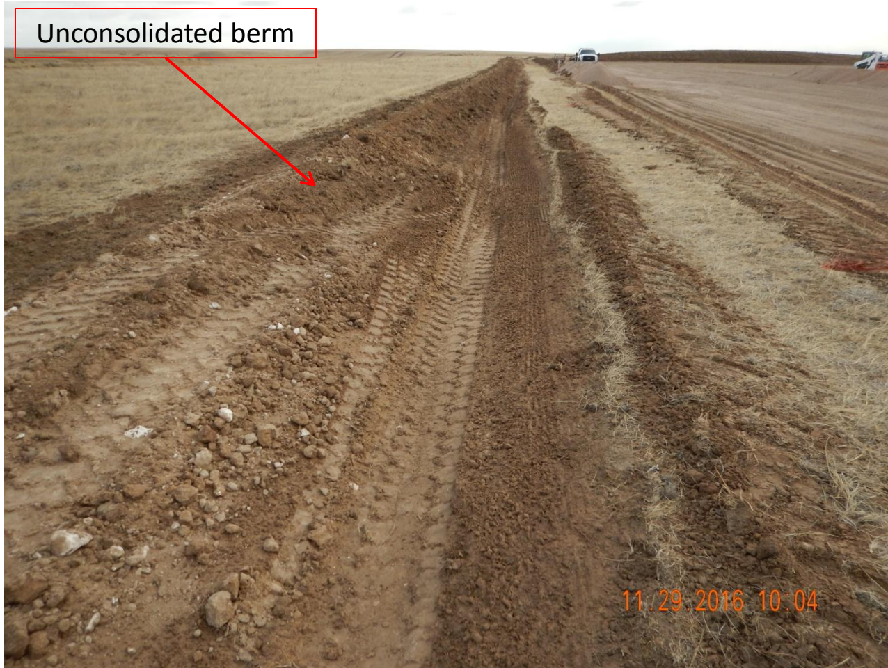
Photo 2. Photo taken from entrance of location , facing East. Ditch and berm BMP installed around the location perimeter. Berm shall be compacted to ensure containment of sediment laden storm runoff is directed to the sediment trap.
