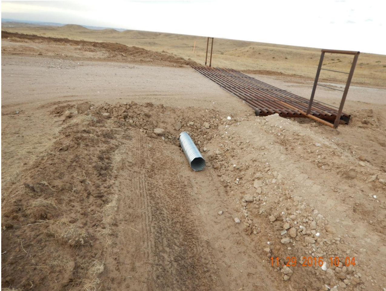
Photo 1. Photo taken from entrance of location , facing West. Ditch and berm BMP installed around the location perimeter. Berm shall be compacted to ensure containment of sediment laden storm runoff is directed to the sediment trap. Culvert installed in conjunction with ditch and berm BMP.
