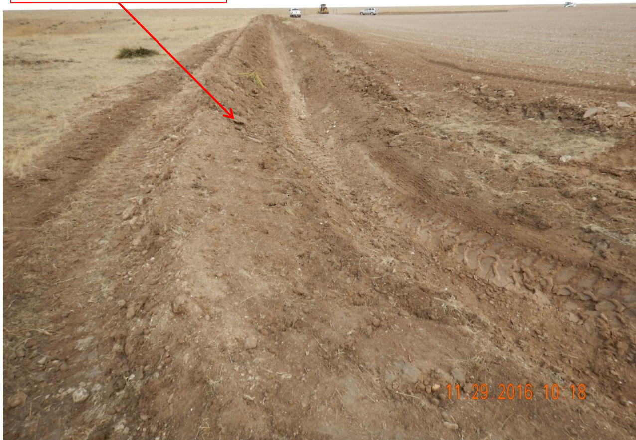
Photo 6. Photo taken from the western location , facing North. Ditch and berm BMP installed around the location perimeter. Berm shall be compacted to ensure containment of sediment laden storm runoff is directed to the sediment trap.
