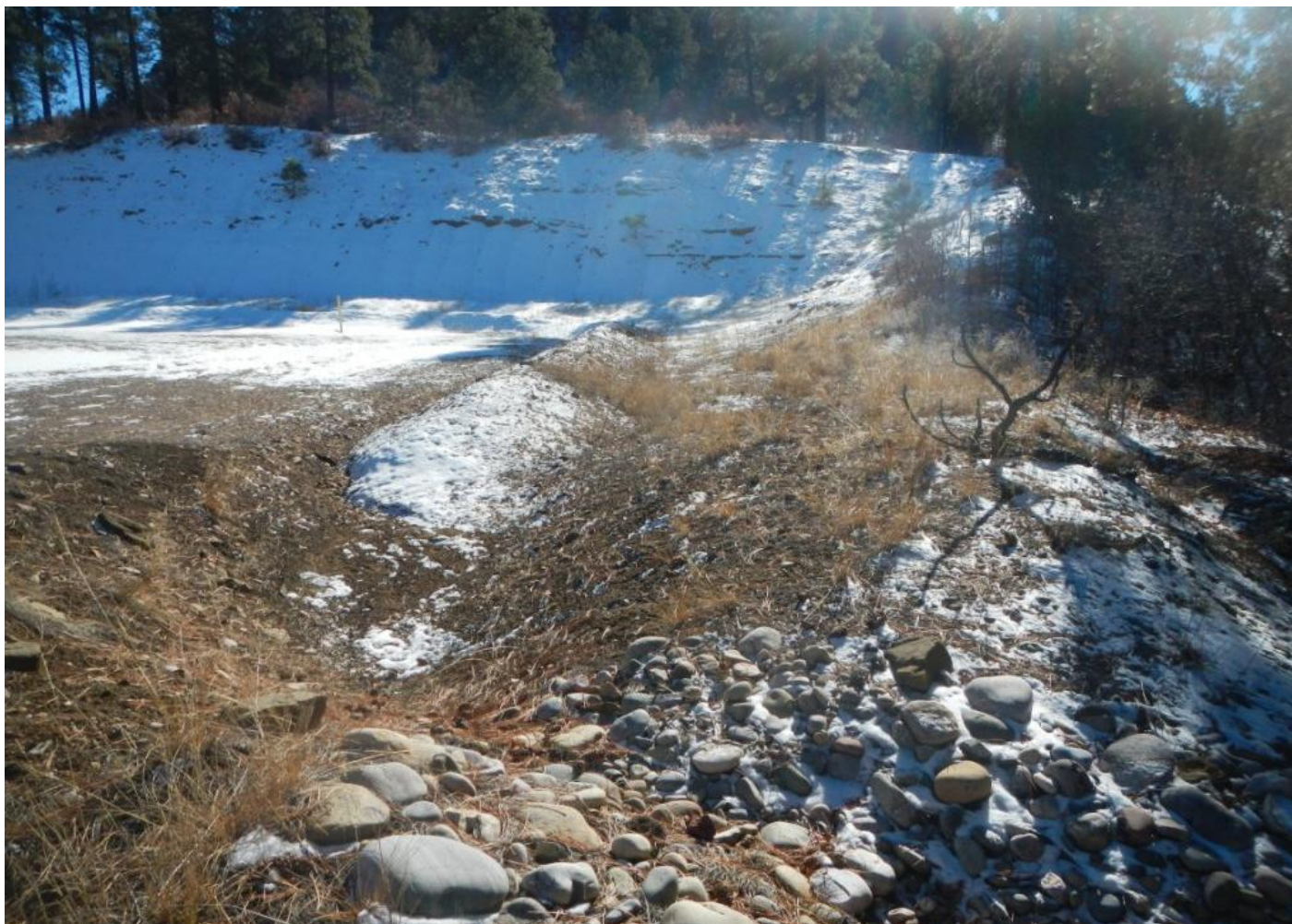
Photo 3. View of the western portion of the project area from the northwestern edge facing southward. Stormwater diversion is in good condition and revegetation is progressing on fill slopes.
