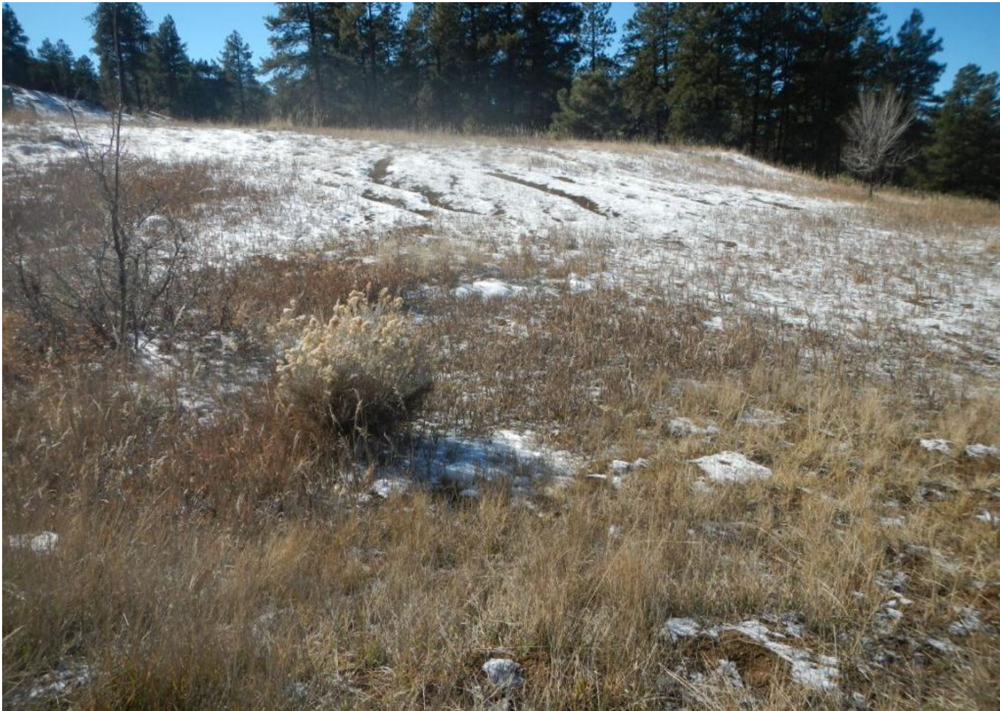
Photo 5. View of the northern portion of the project area from the access road facing southwestward. Rill erosion is occurring on the fill slopes. This should be monitored and BMPs applied if erosion worsens.
