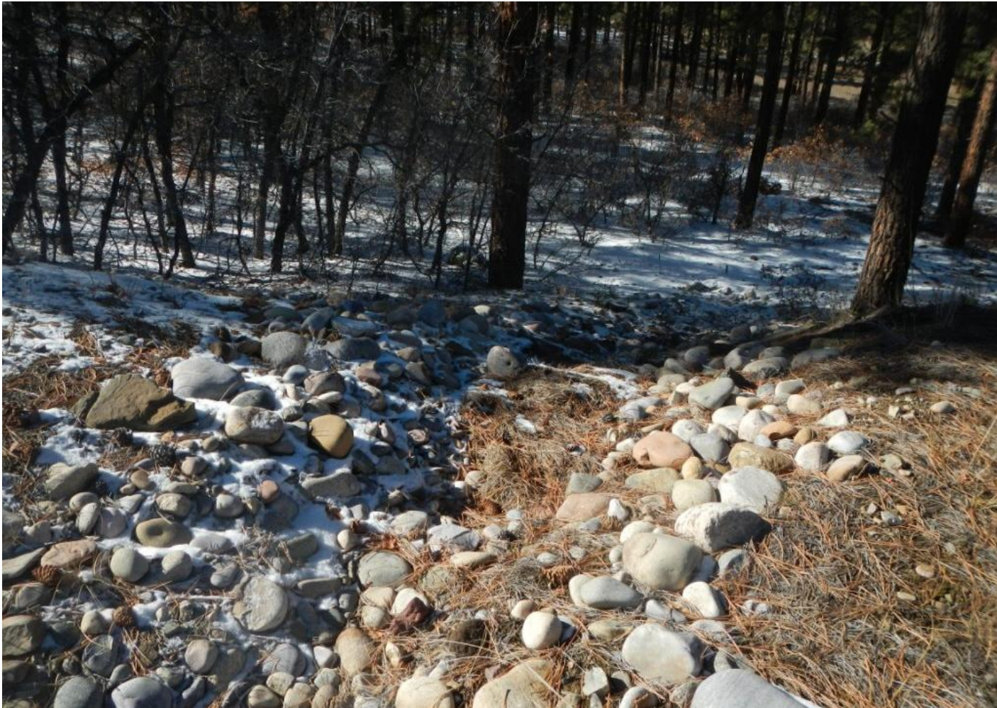
Photo 4. View of cobble run-down in northwestern portion of the project area that is downstream from diversion in Photo 3. Run-down is in good condition.
